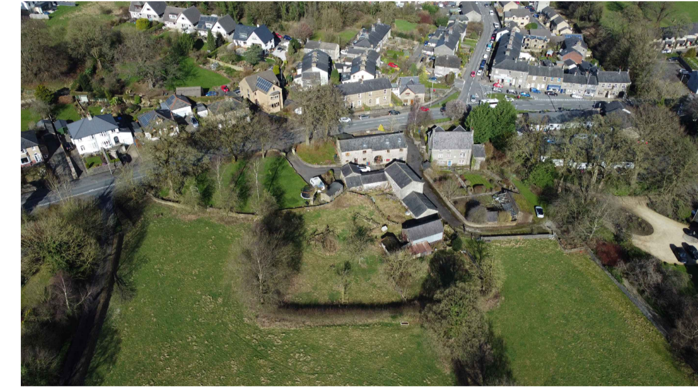
Aerial view of the site looking towards the northern boundary
