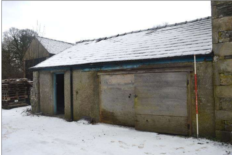
Plate 86 (shot 31): Northeast elevation of the workshop, looking south, 2, scale
