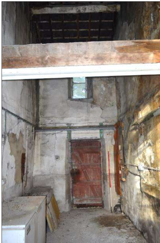
Plate 53 (shot 130): View of extension, looking south-southeast, 2m scale
