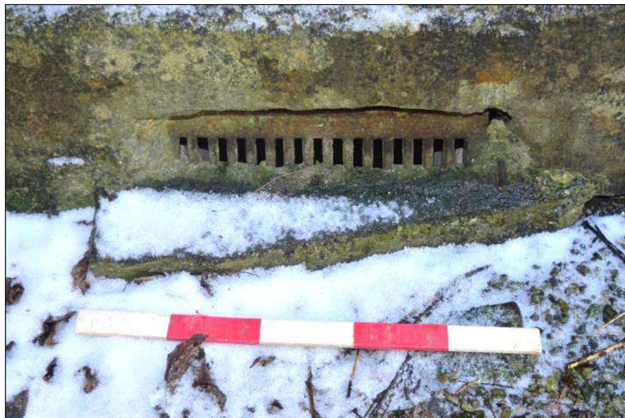
Plate 6 (shot 89): Ventilation brick for the cellar, looking southwest, 0.5m scale
