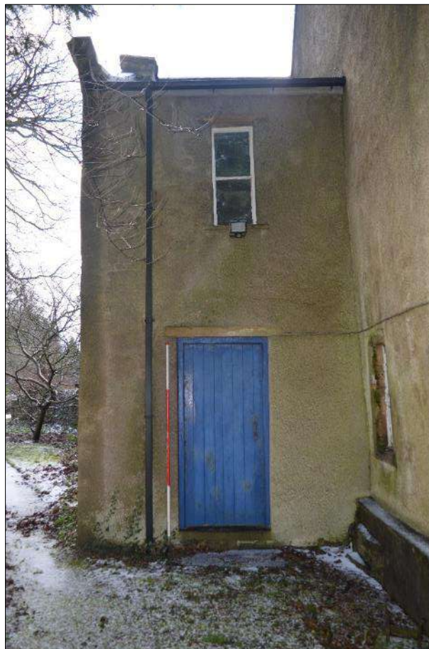
Plate 49 (shot 85): Northwest elevation, looking south-southeast, 2m scale
