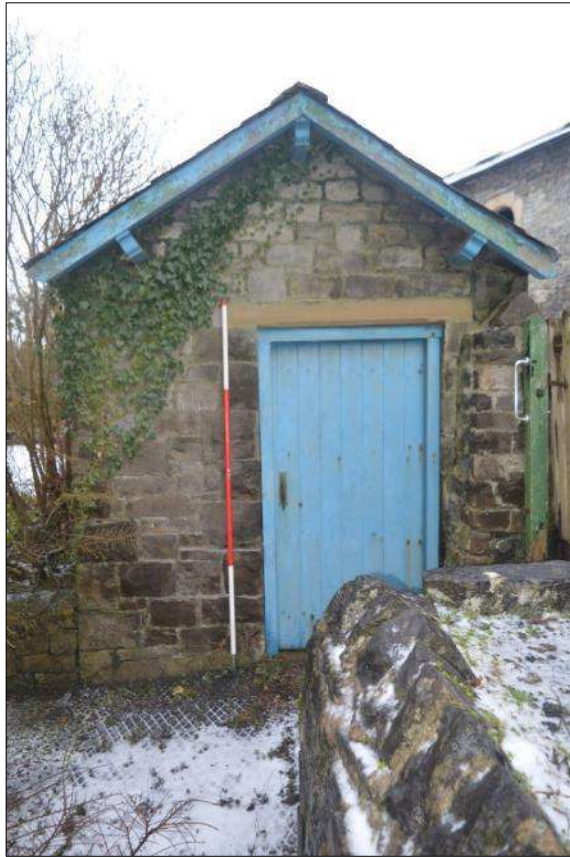
Plate 61 (shot 62): The coalhouse southwest of the farmhouse, looking south-southeast, 2m scale
