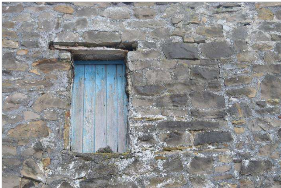
Plate 74 (shot 51): Reduced first floor opening, looking northeast
