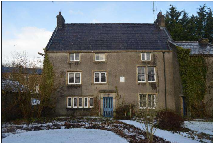
Plate 8 (shot 108): Southeast elevation with extension A2 to the right, looking north-northwest, 2m scale
