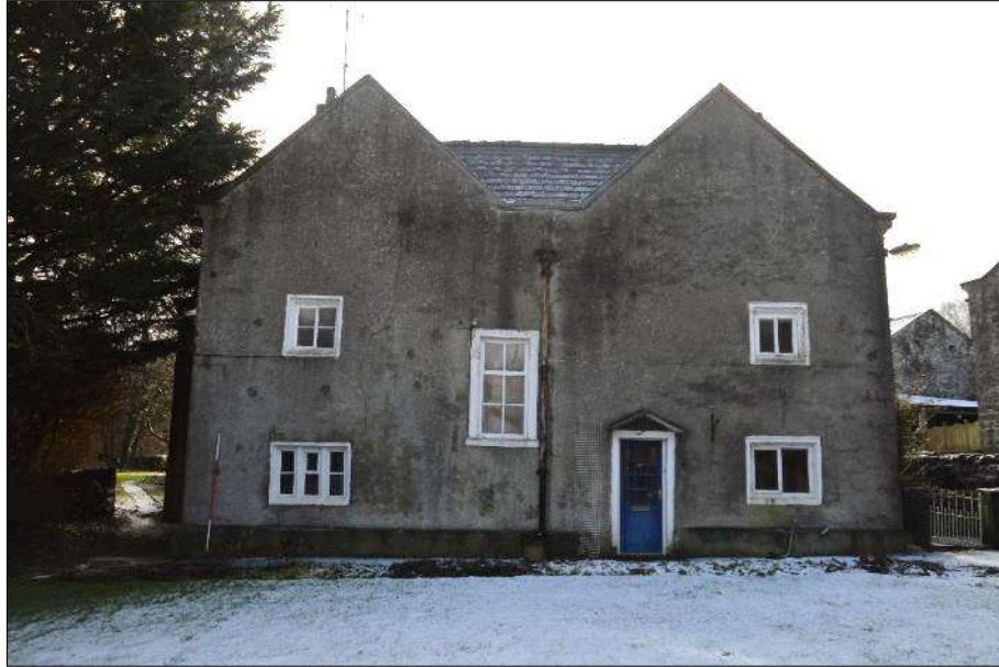
Plate 2 (shot 94): Northwest elevation of the farmhouse, looking south-southeast, 2m scale
