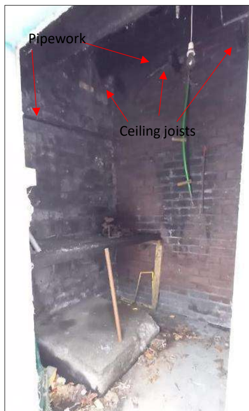
Plate 91 (shot 34): Restricted view of workshop room (3.1), looking south
