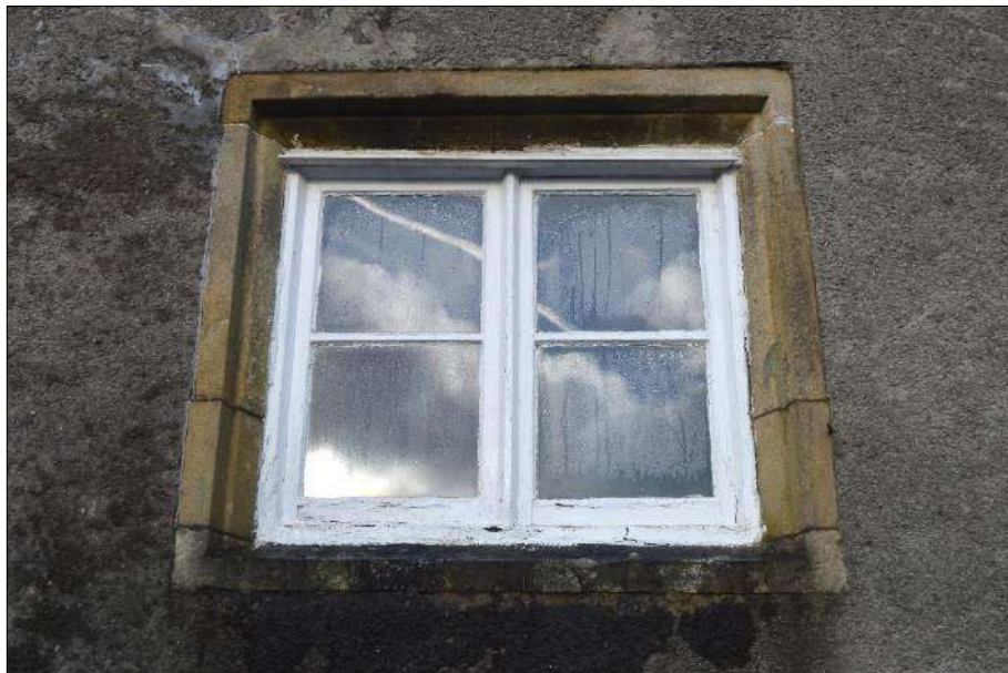
Plate 10 (shot 109): Close up of first floor window with moulded surround, looking north-northwest
