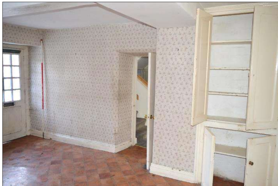
Plate 19 (shot 144): View of altered wall between pantry and kitchen, looking east-northeast, 2m scale
