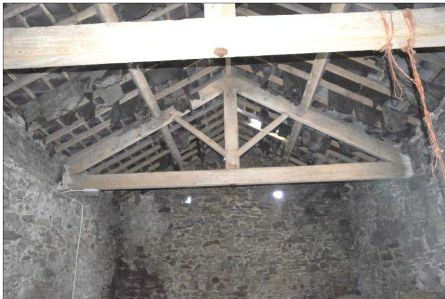
Plate 81 (shot 27): Kingpost roof truss, looking northwest
