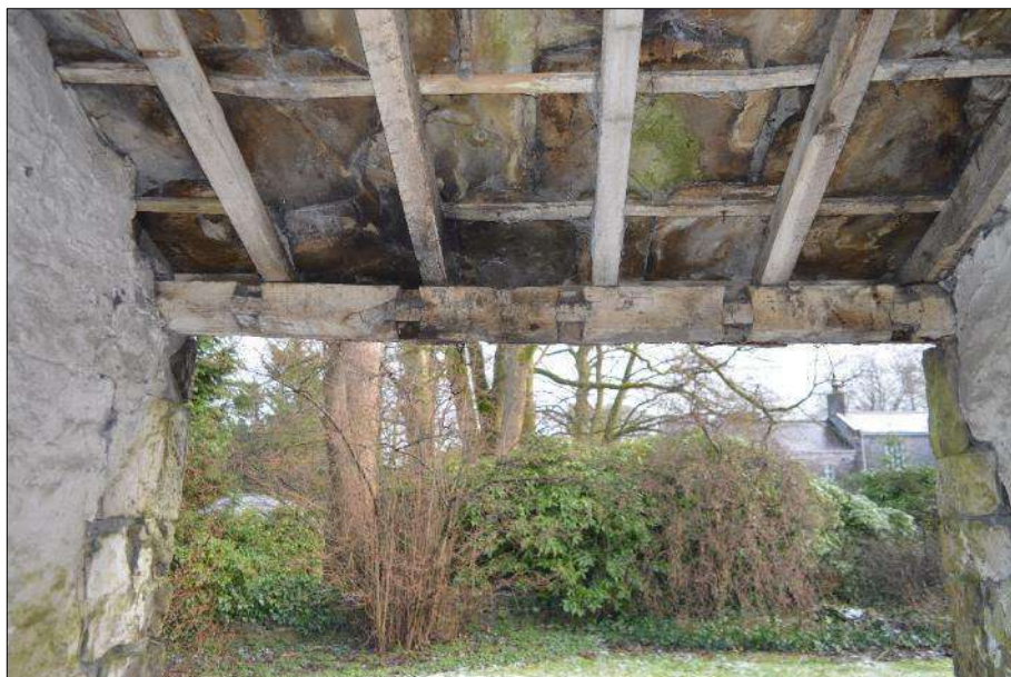
Plate 68 (shot 81): Reused main beam as wall plate, looking northeast
