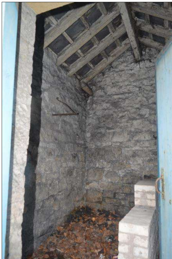
Plate 62 (shot 63): Interior view of the coalhouse, looking east-southeast
