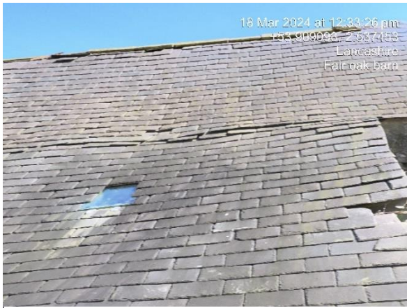
Photo 5: Raised tiles, numerous where the two roofs join and at roof ridge. Raised ridge tiles and some missing tiles.
