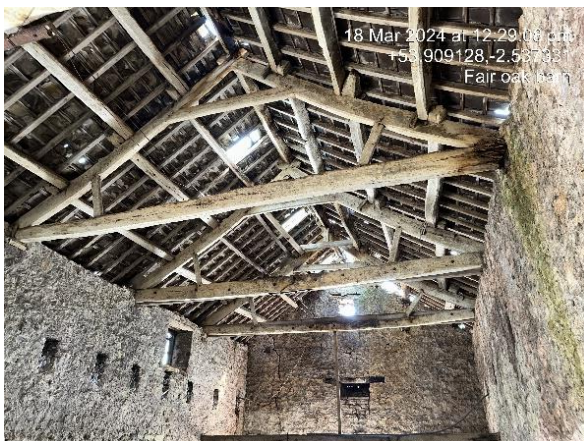
Photo 7: Internal space. Light ingress present. Alcoves in wall, gaps between wooden beams.
