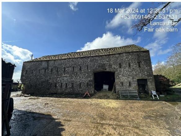
Photo 1: Eastern aspect of the barn.
