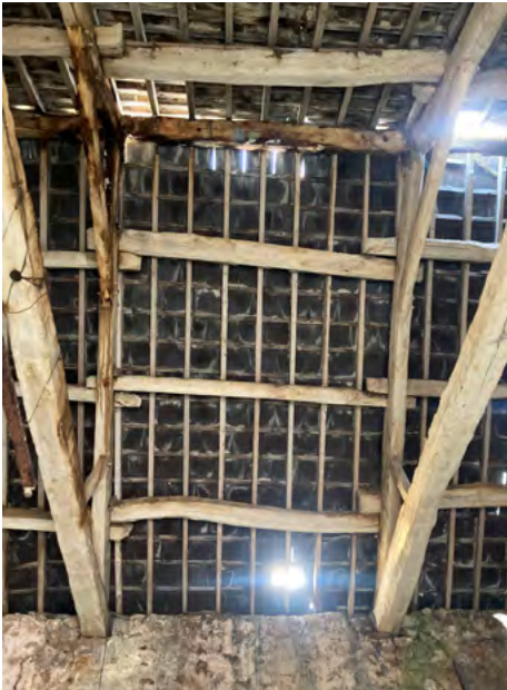
North central bay east side
