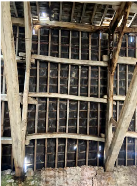
North central bay west side
