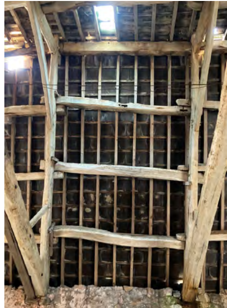
South central bay west side
