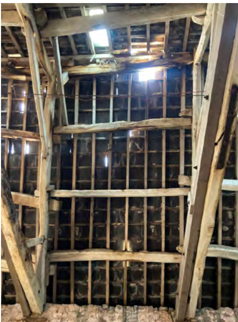
South mid bay west side
