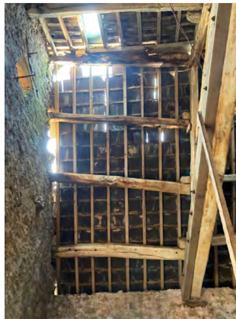
South end bay west side
