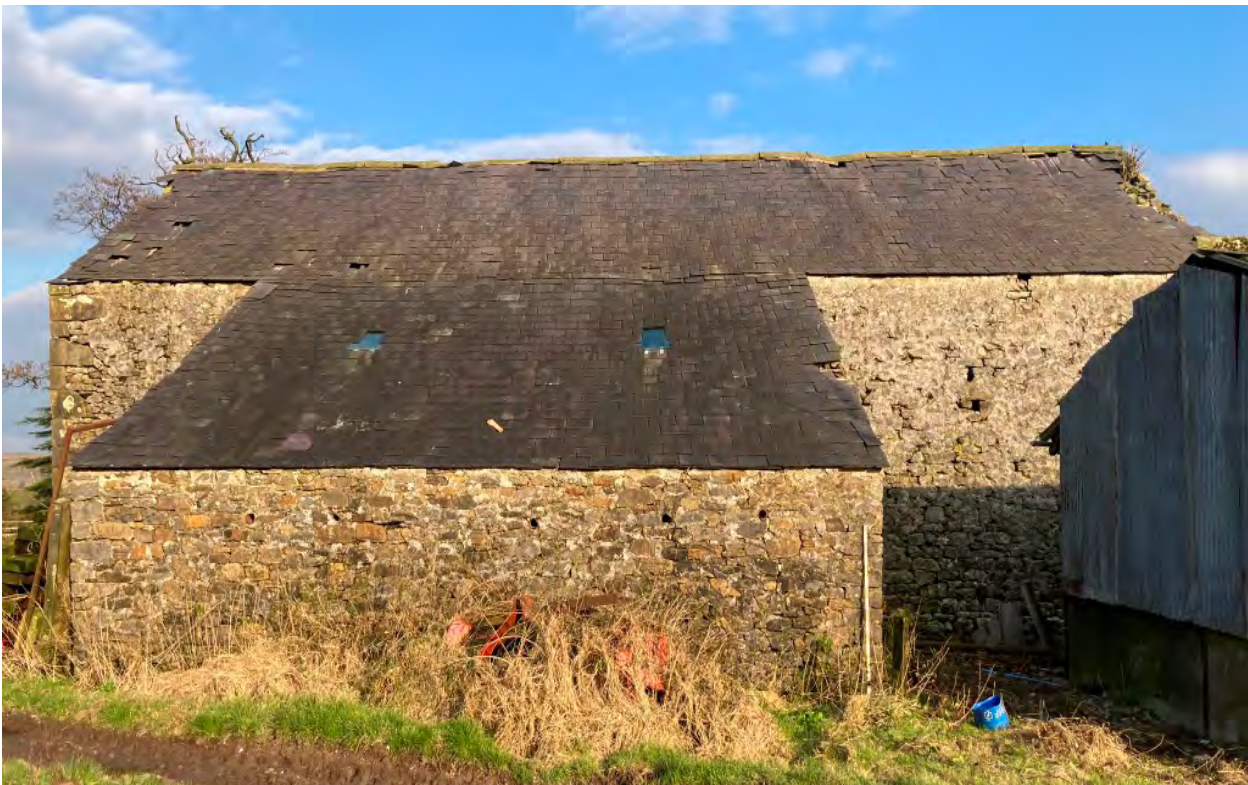
Rear west elevation of barn
