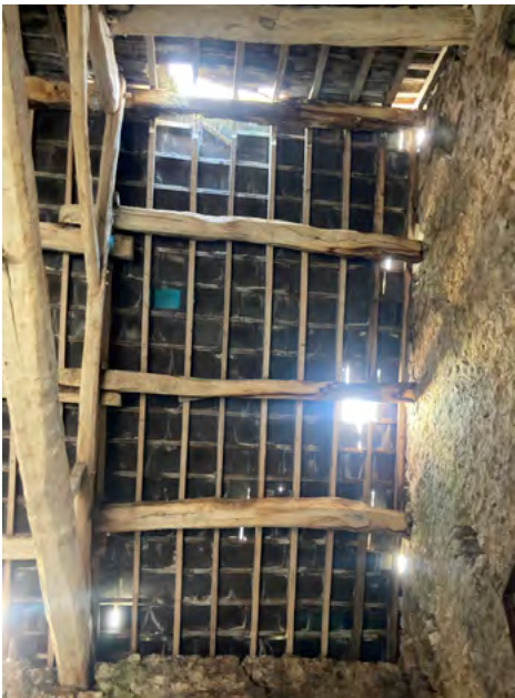
North end bay west side
