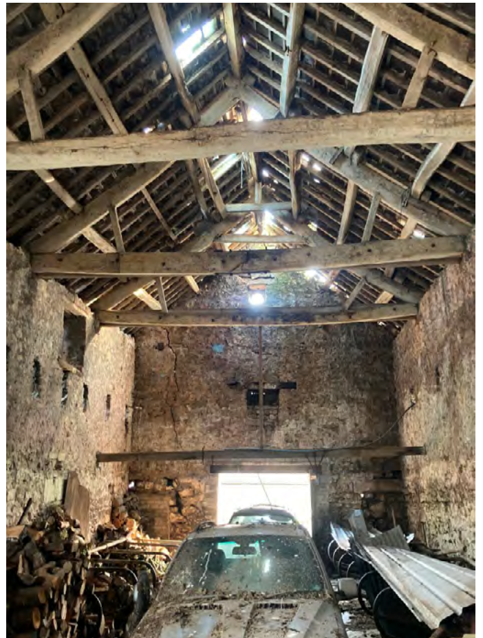
General view of the main barn looking south.
