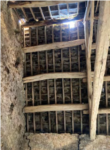
North end bay east side
