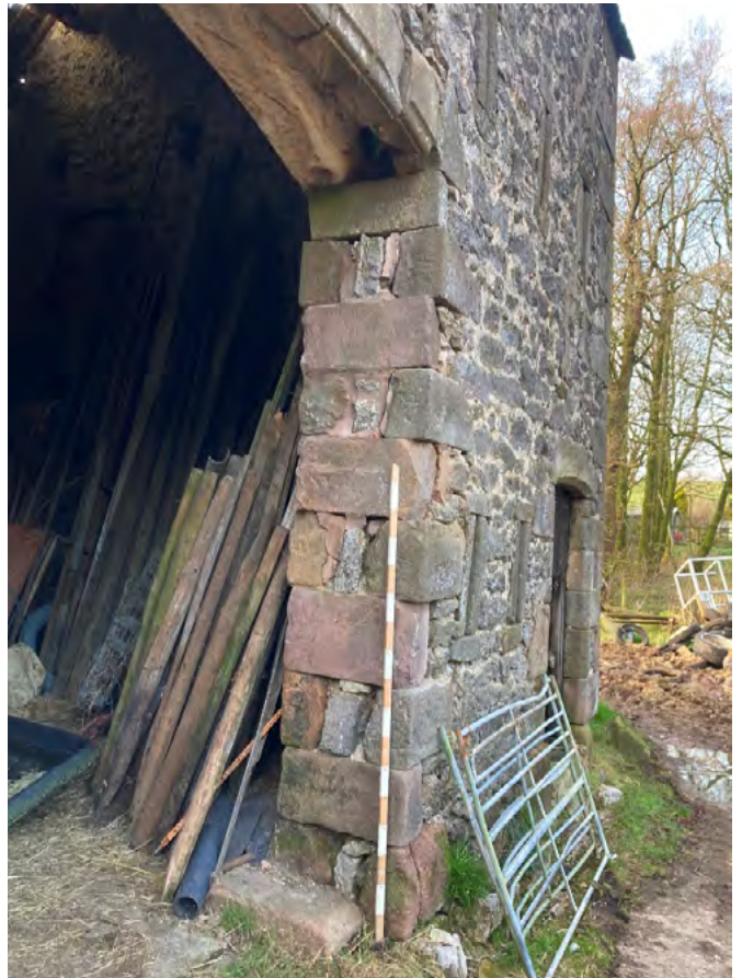
View of north jamb of threshing doorway . Note footing for lost threshing doors.
