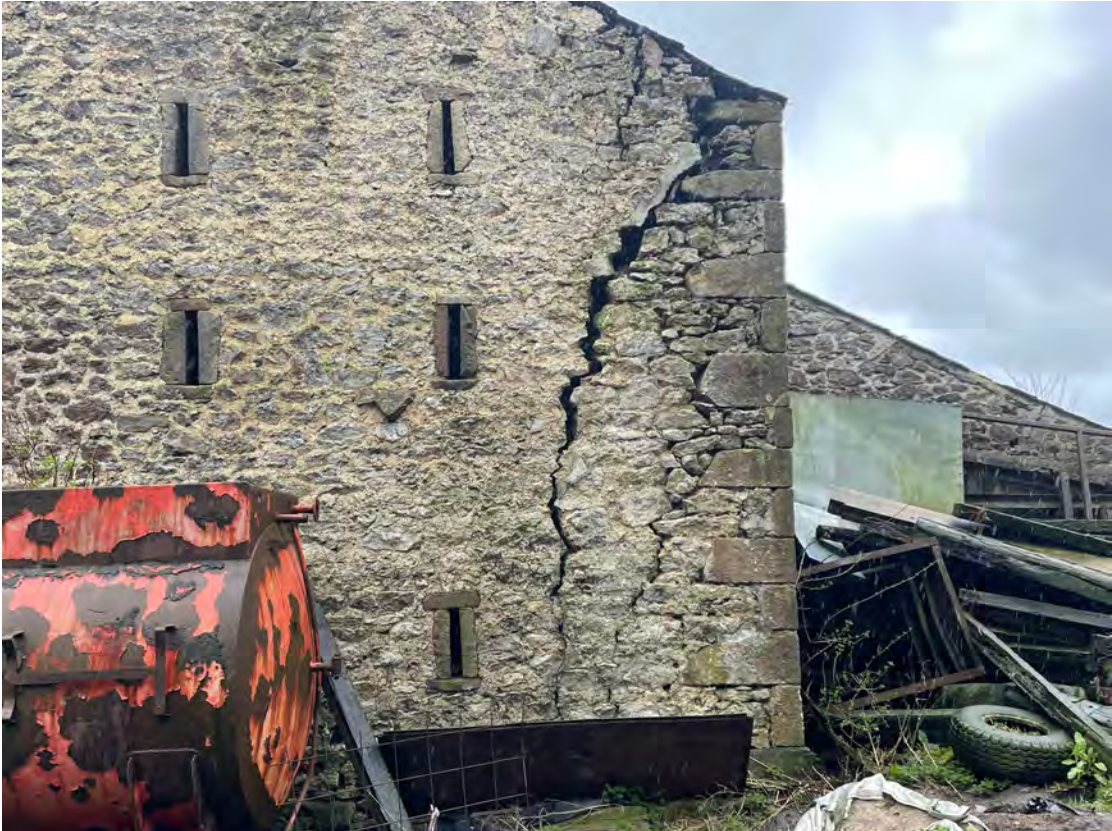
Photo 9: North Gable Wall
