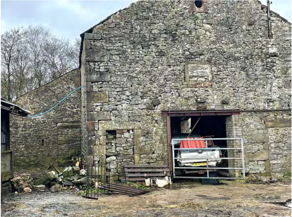
Photo 7: South Gable Wall
