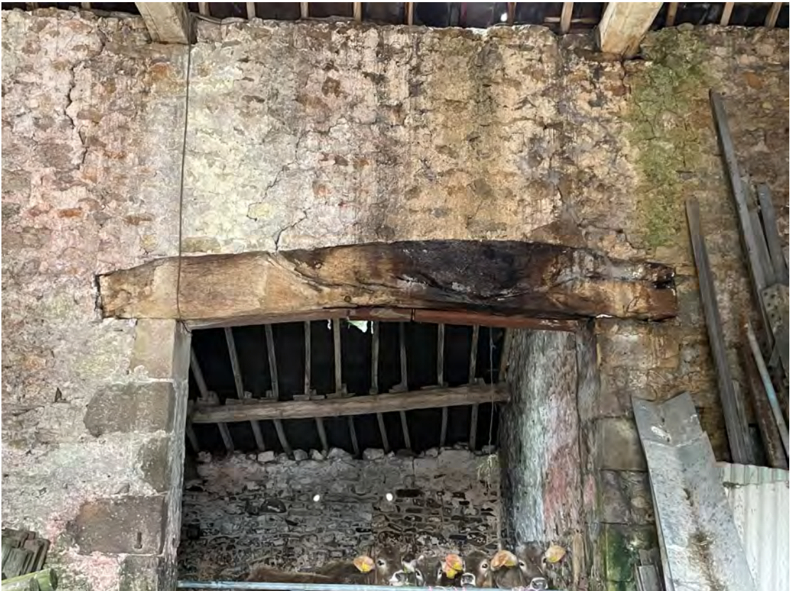
Photo 2: Cart Entrance to Rear Outshut
