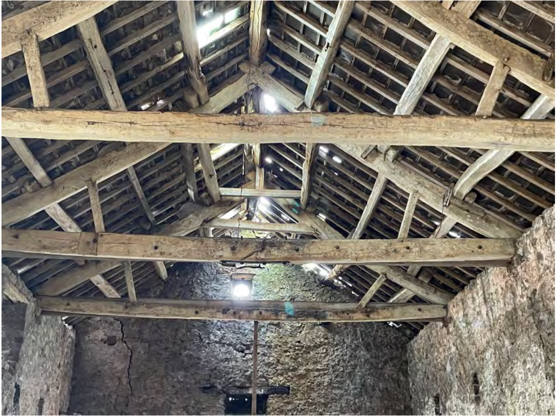
Photo 3: Roof Looking South
