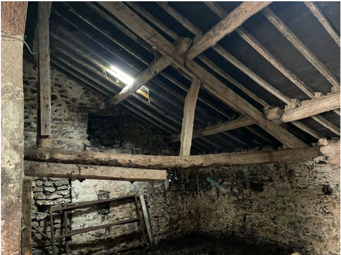
Photo 4: Roof of Outshut
