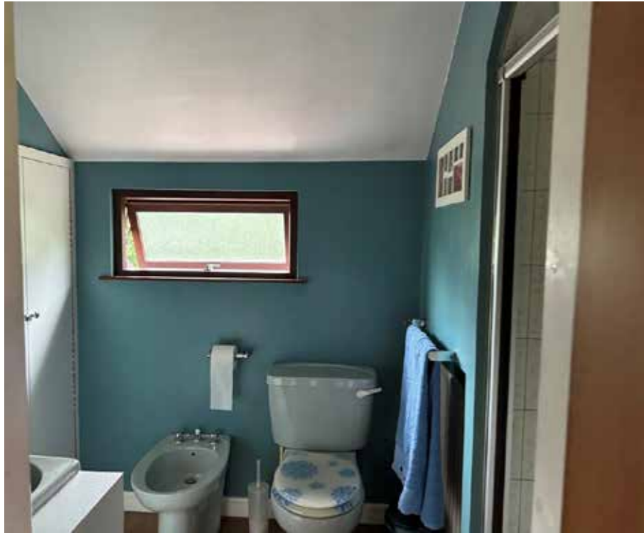
small windows and low ceilings in the existing master bedroom en suite
