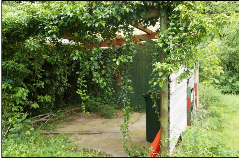
Photo 7: Timber framed carport, clad in plastic and aluminium corrugated sheets and overgrown with ivy.
