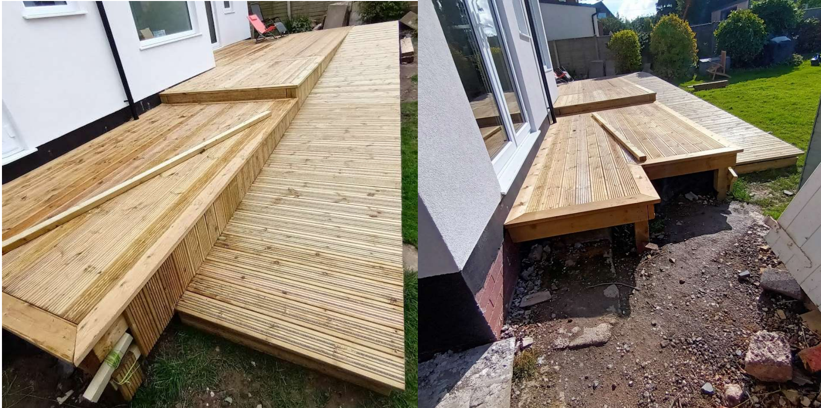
Bottom of ramp with decking at lower side of house
