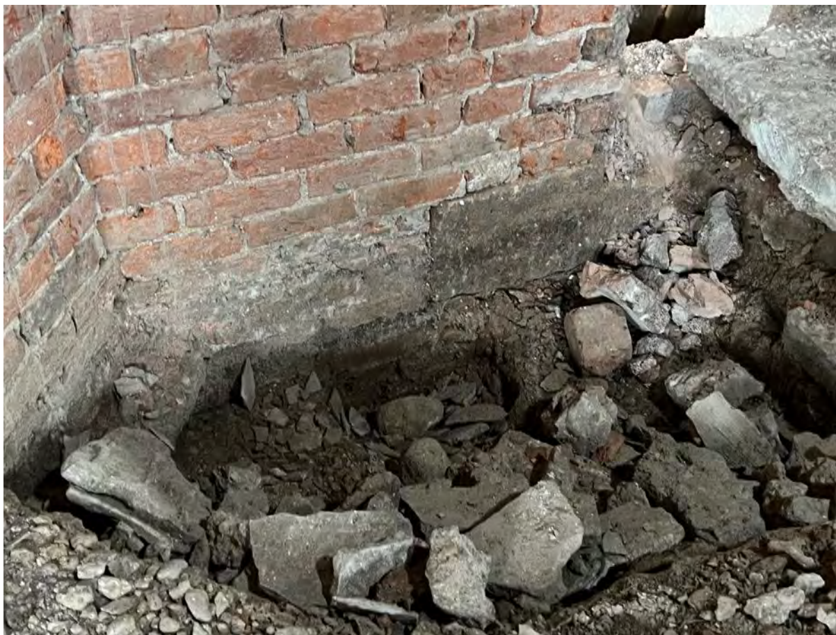
Photo 56 - Internal – main barn – excavation to founding stones
