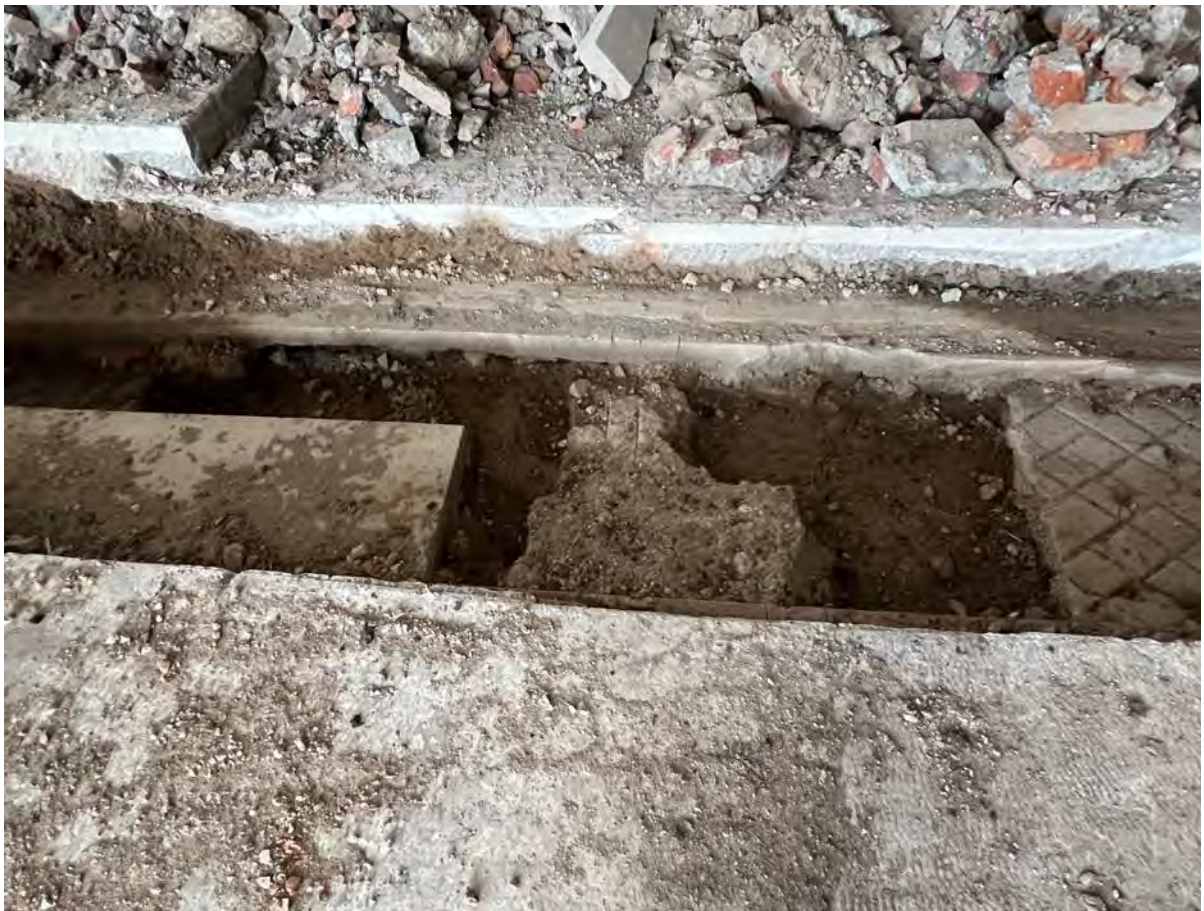
Photo 28 - South West Elevation – excavations to reveal former lean-to section
