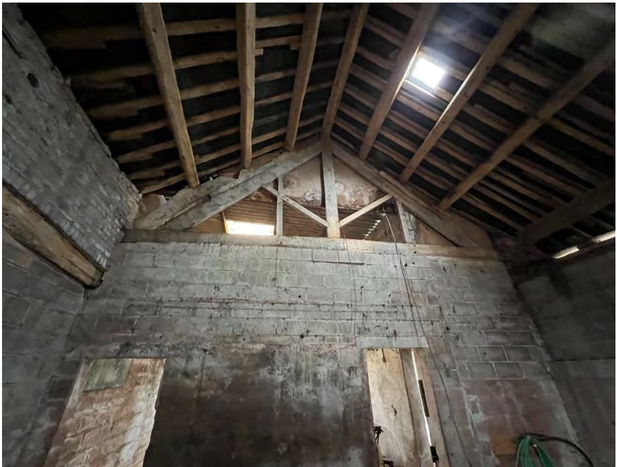
Photo 58 - Internal – main barn – rebuilt gable to main barn to extension at west end
