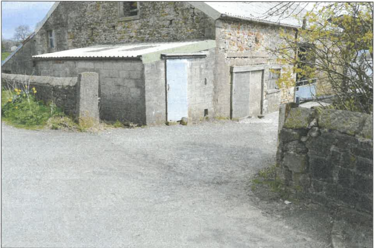
PL06: View of the existing site entrance immediately adjacent to the west corner of the barn.
