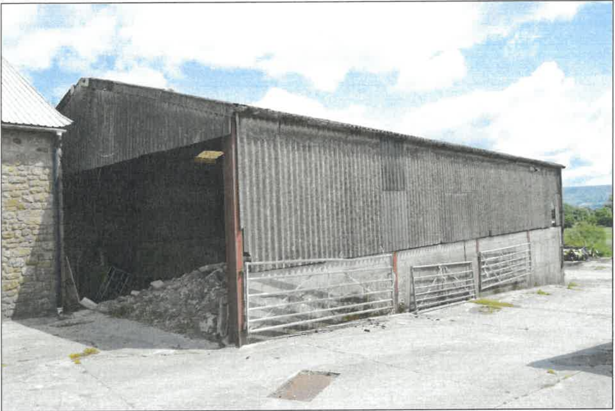
PL07: View of th modern portal frame agricultural building located to the south east of the stone built barn.
