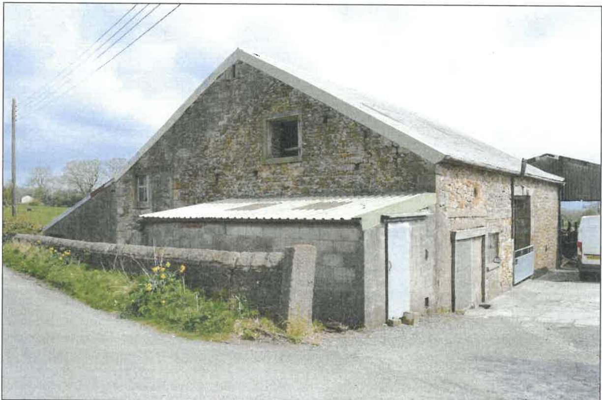
PL02: View of the barn from the north west.
