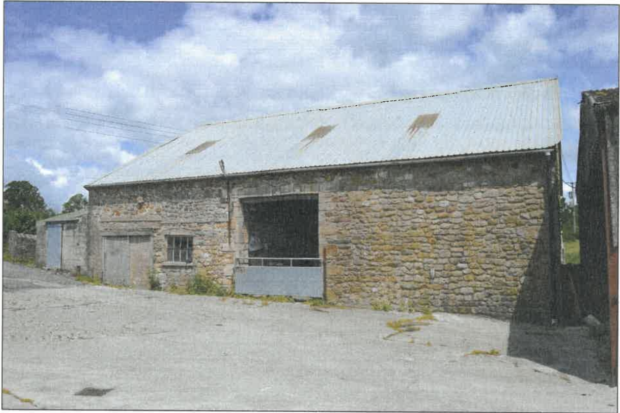
PL01: View of the barn from the south west.
