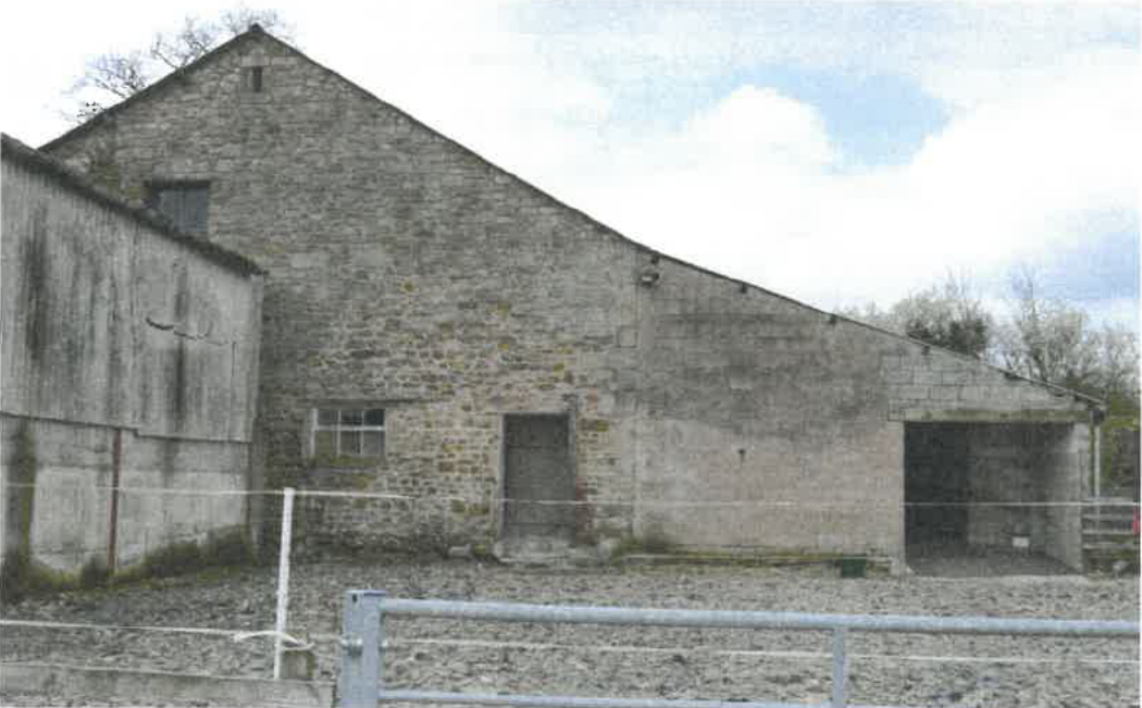
PL03: South East facing photo of Vicarage Farm Barn (Side 2 Elevation)
