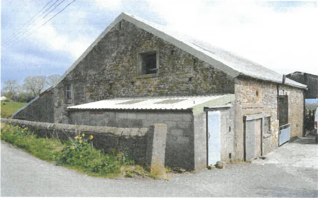
PL02: North West facing photo of Vicarage Farm Barn (Side 1 Elevation)
