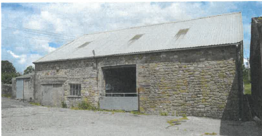
PLO1: South West facing photo of Vicarage Farm Barn (Front Elevation)
