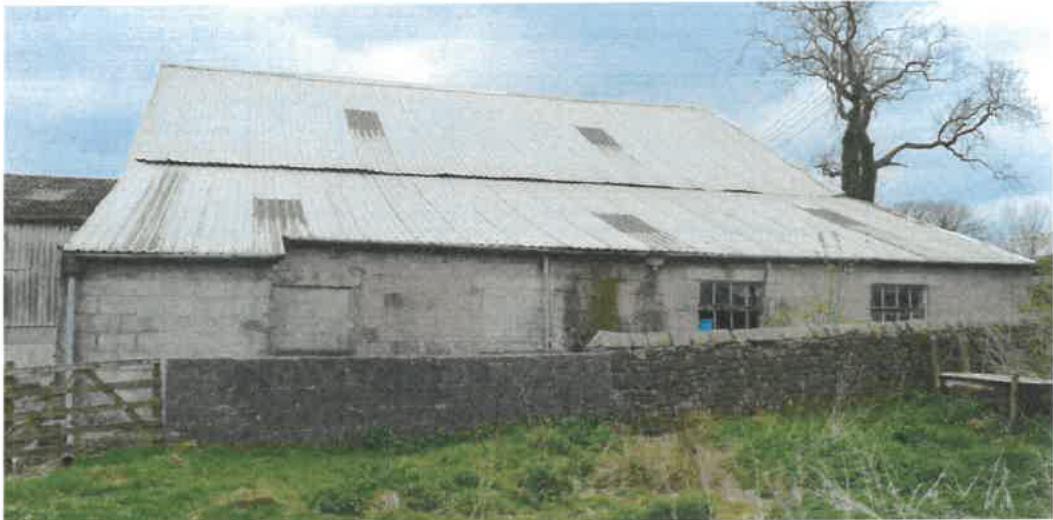
PL04: North East facing photo of Vicarage Farm Barn (Rear Elevation)
