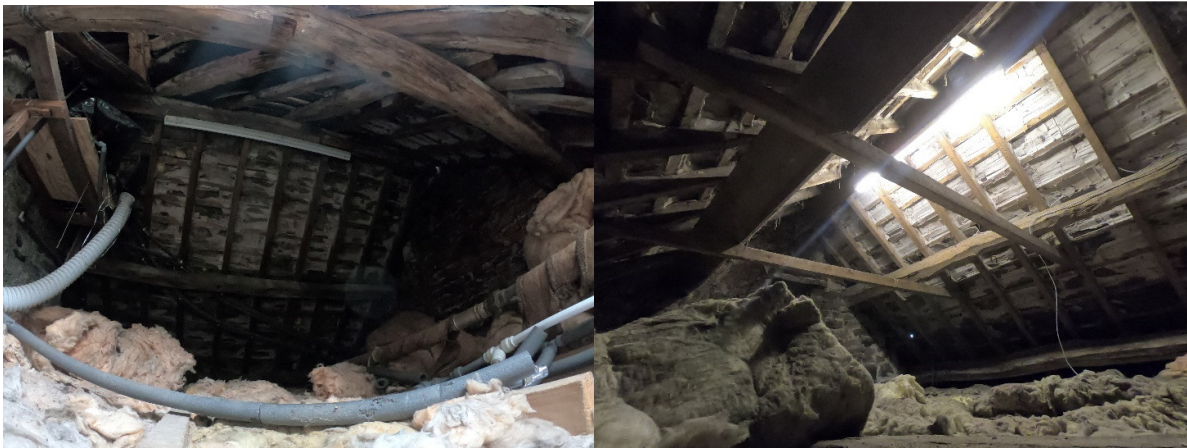
Bare tiles with deteriorating lime mortar application above bedrooms 3 and 4
