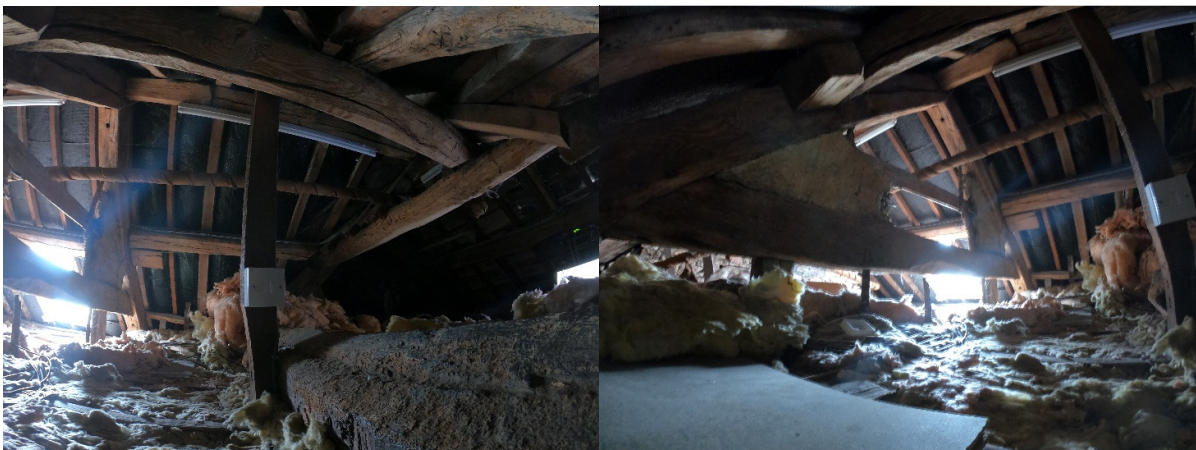
Traditional bitumen underfelt above bathroom 1 and the adjacent corridor
