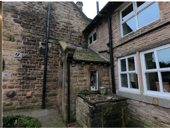
Existing black upvc soil pipes
