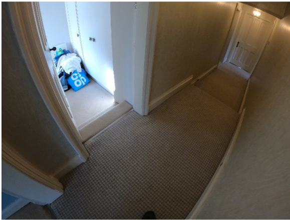
Steps over the floor void extend into the corridor
