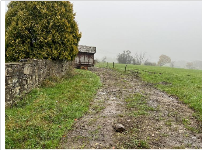
Photo 1: Driveway into the barn
