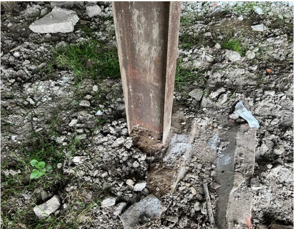
Photo 19 – Internal – column to ridge beam
