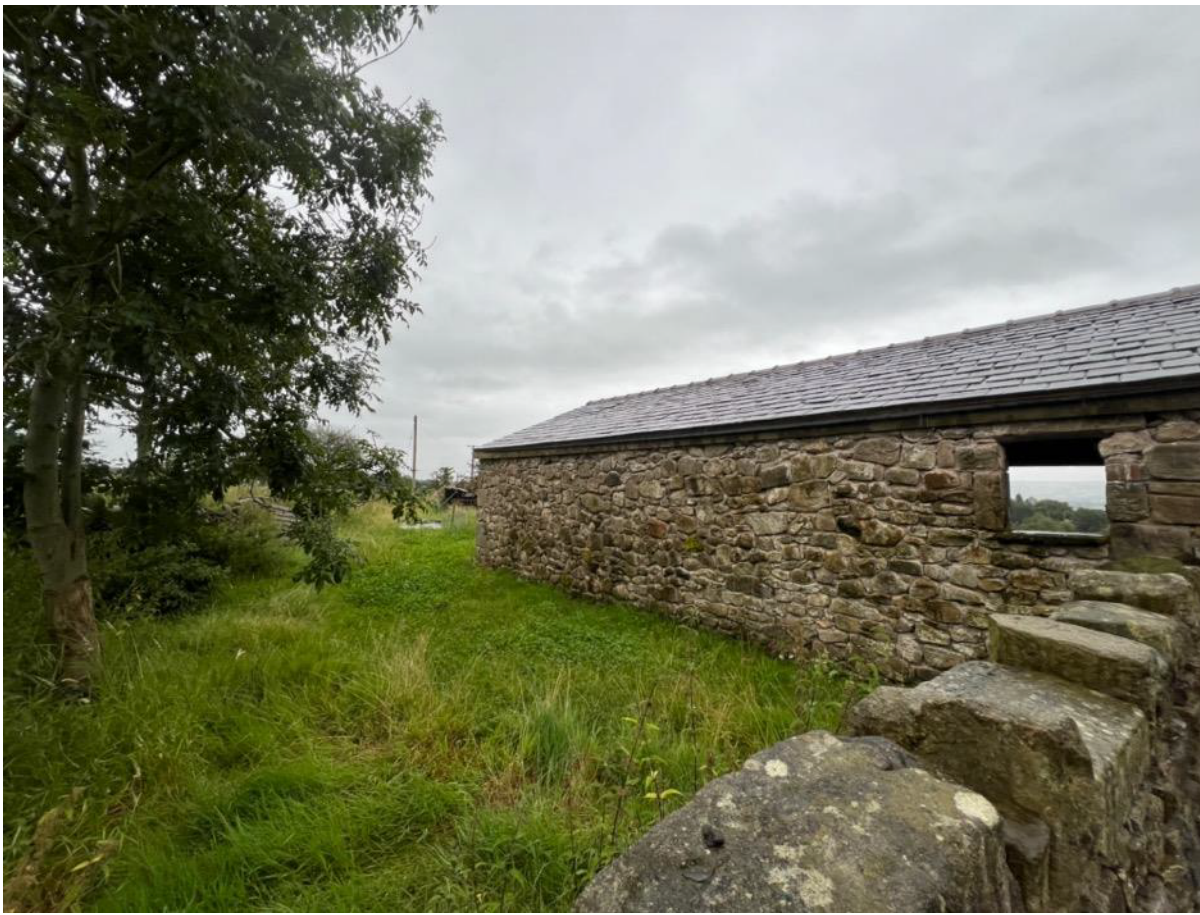
Photo 3- North Elevation – east end
