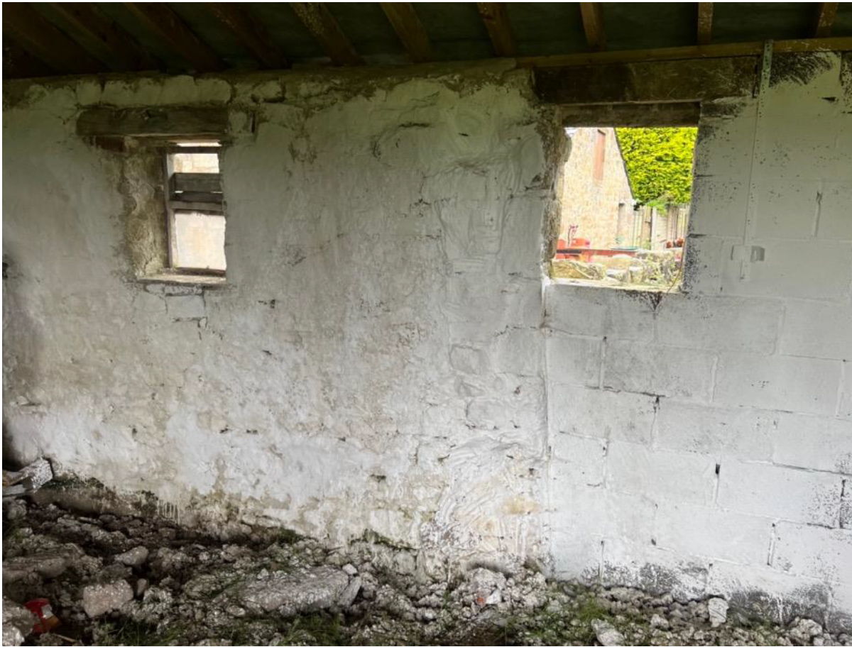
Photo 16 – Internal looking north
