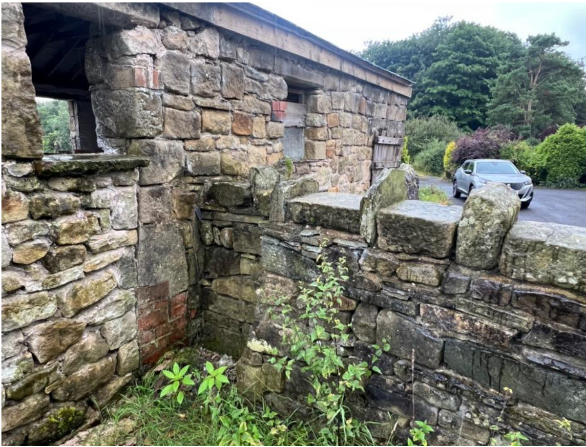
Photo 5 – North Elevation at boundary wall
