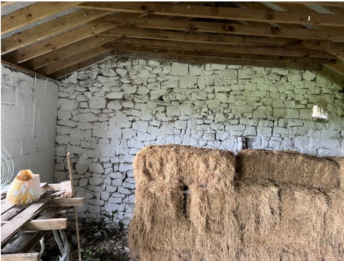
Photo 15 - Internal looking west
