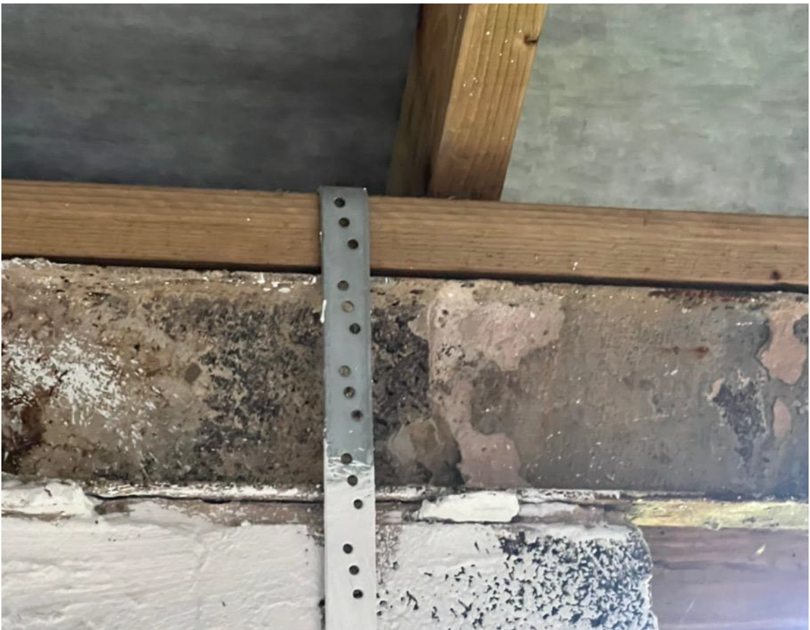
Photo 20 – Internal – wall plate and strapping
