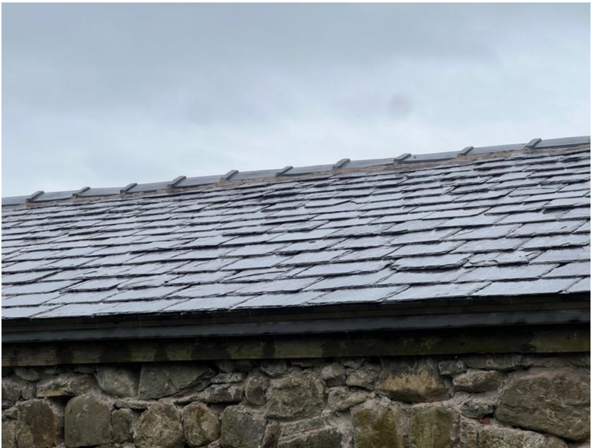
Photo 12 – Roof to south
