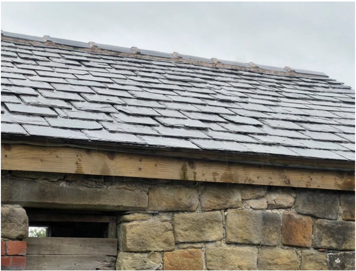
Photo 11 – Roof to North
