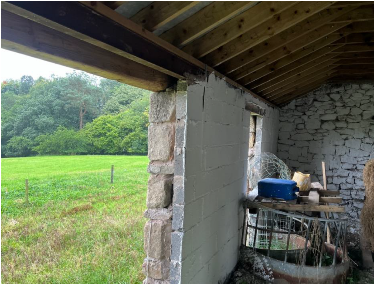
Photo 14 - Internal looking south
