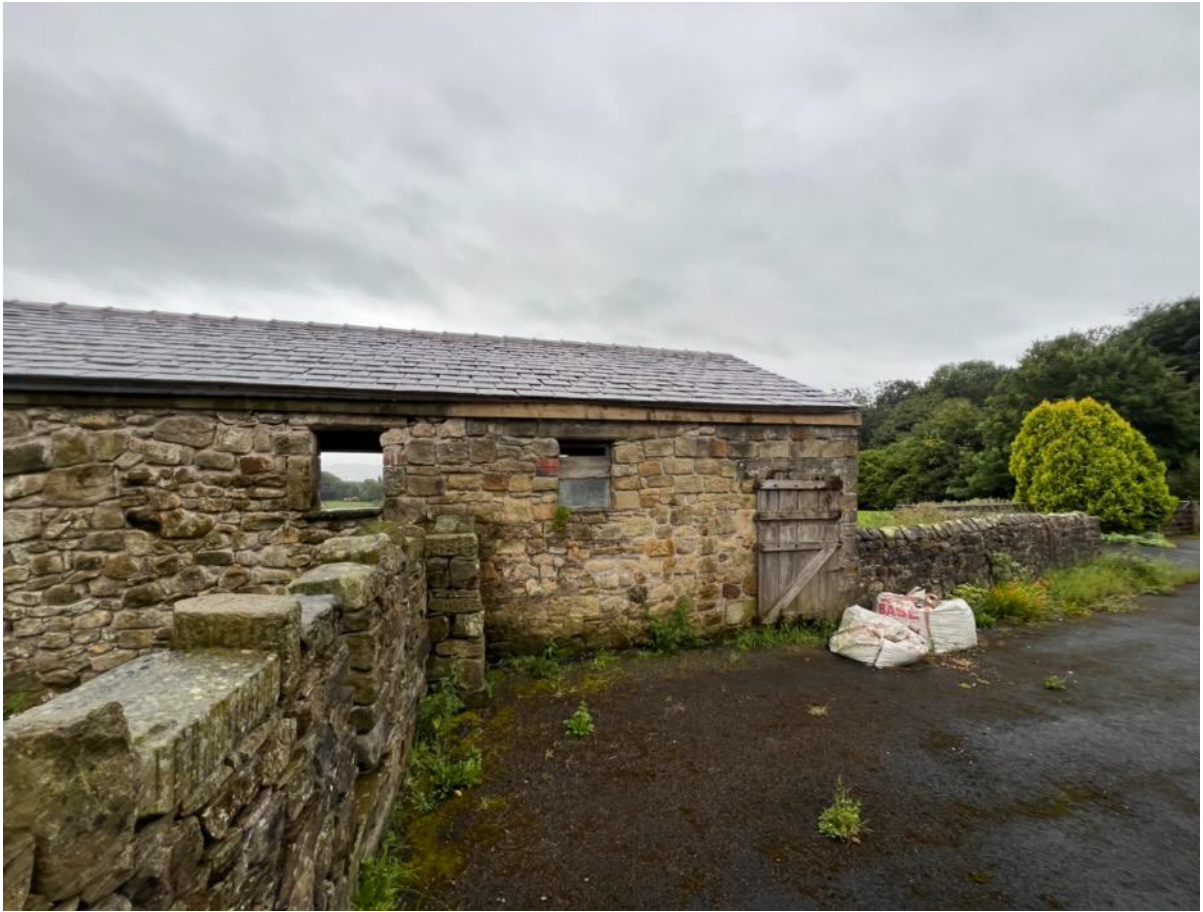
Photo 2 – North Elevation – west end
