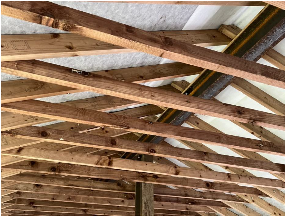
Photo 18 – Internal – roof structure
