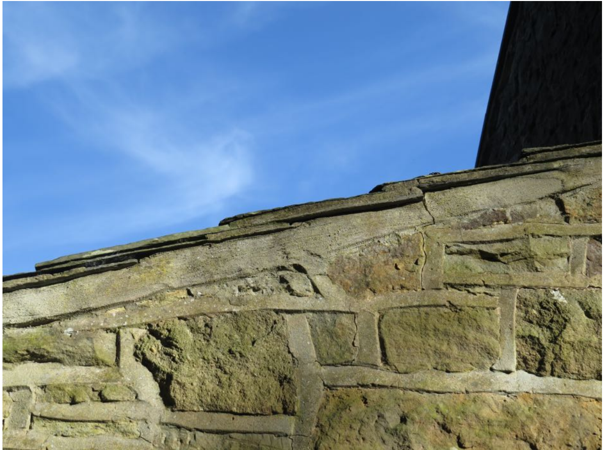
9 – Cement at the verges is intact with no viable gaps.
