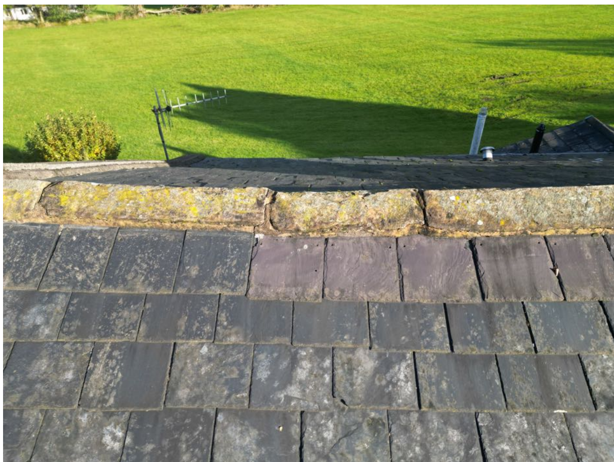
3 – Roof and ridge tiles are in good condition with no suitable gaps.
