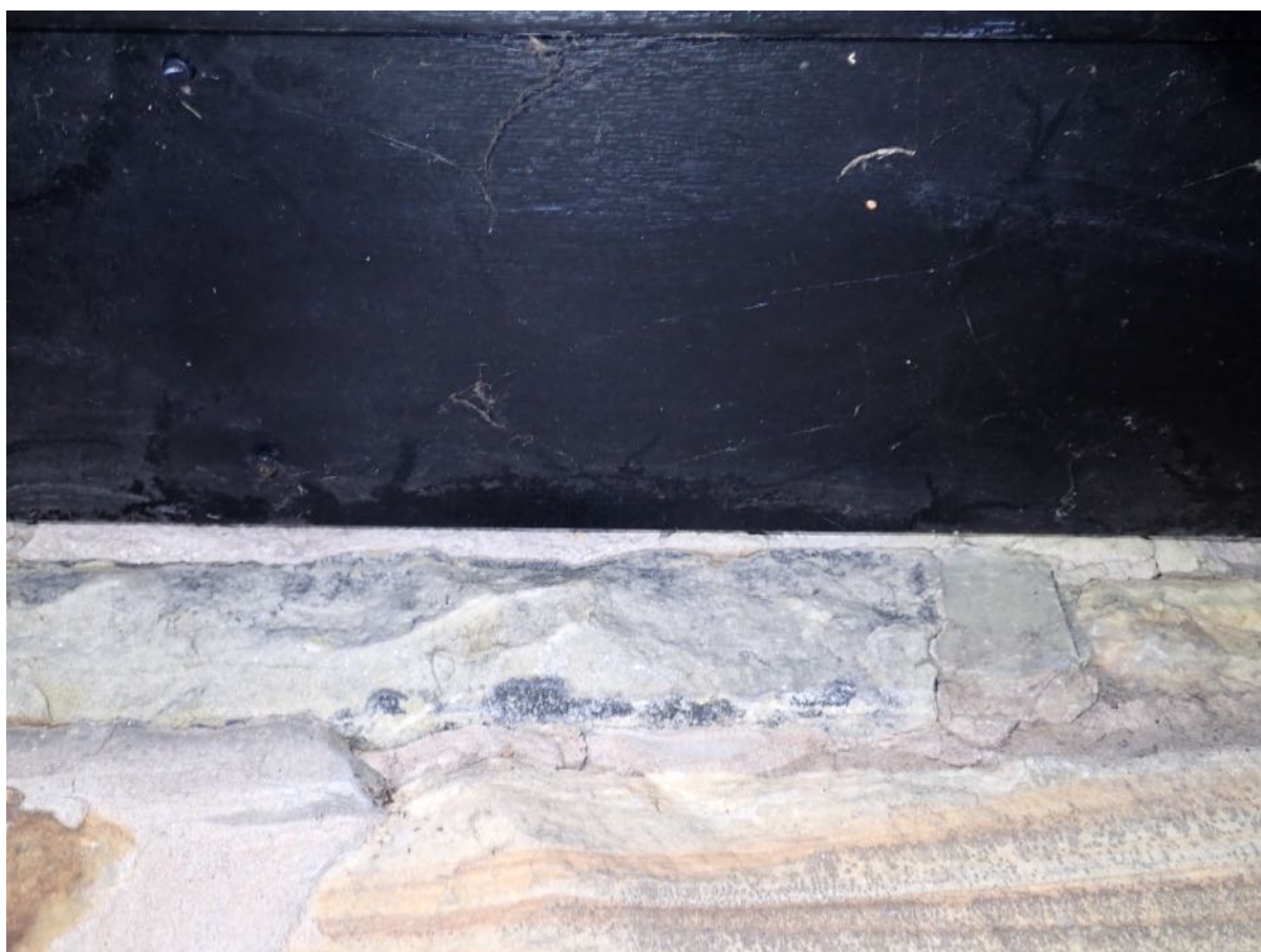
4 – Soffits at the eaves of the extension are fixed tightly against brickwork.
