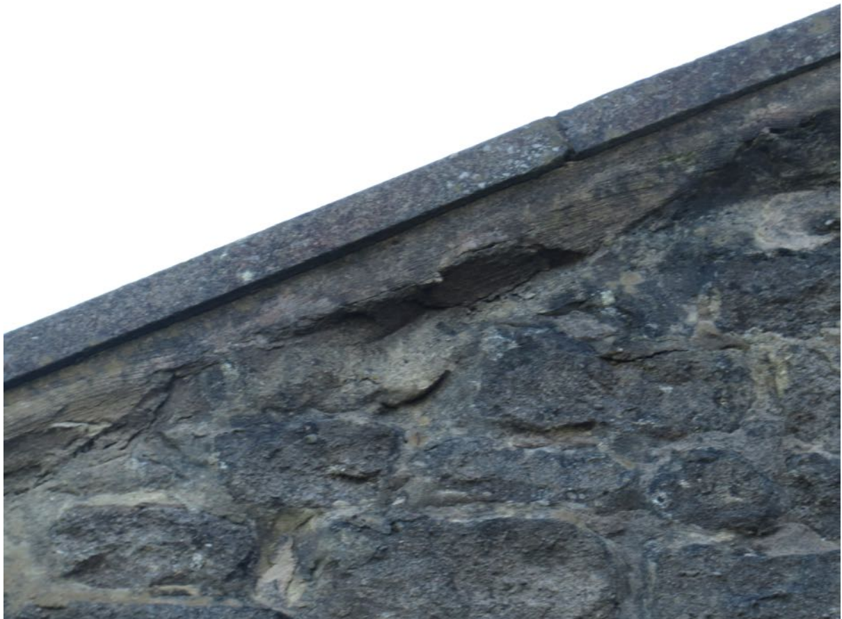
8 – Capping stones at the gable end are fitted tightly with no suitable gaps.
