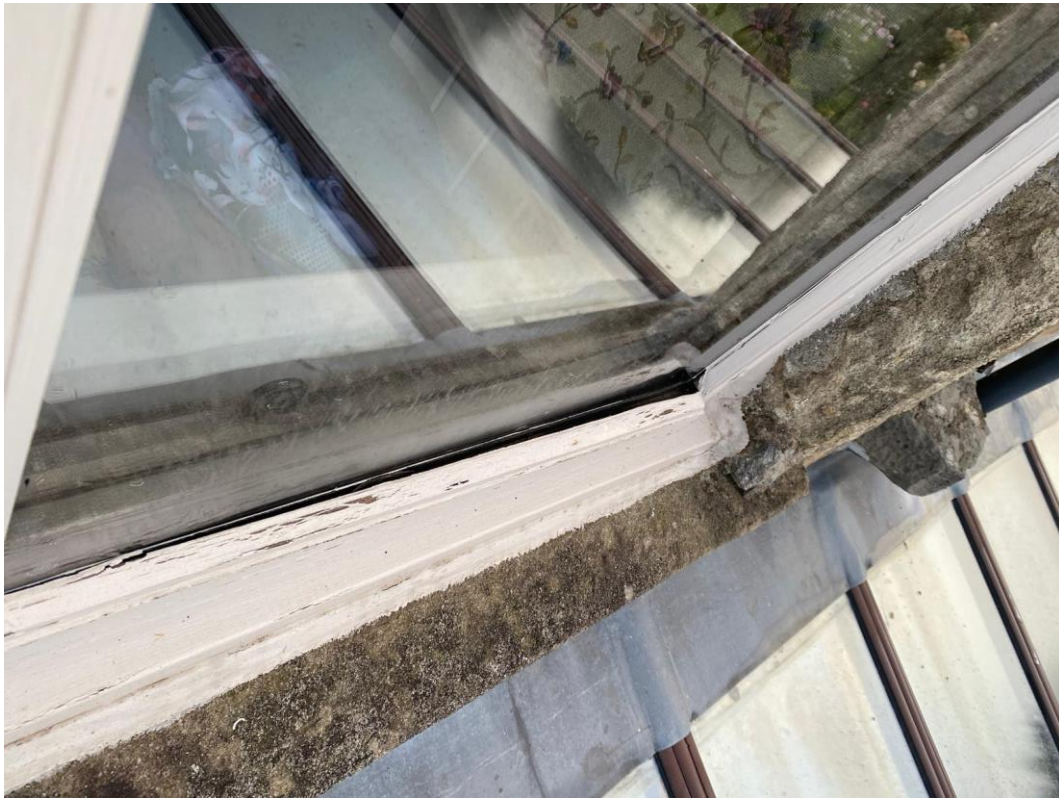
Photo 3: External damage to bottom of side hung sash
