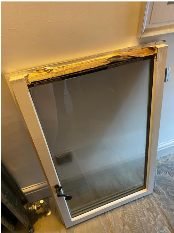
Photo 4: Sash removed for emergency/ temporary repair
