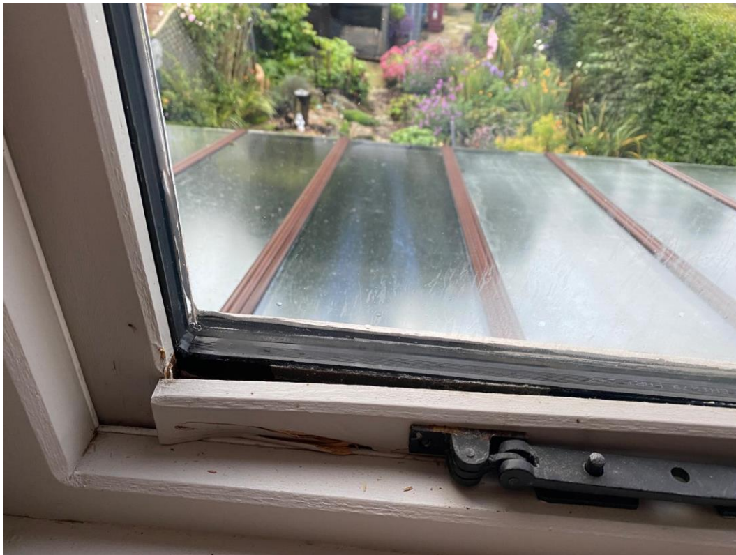
Photo 2: Internal damage to bottom of side hung sash
