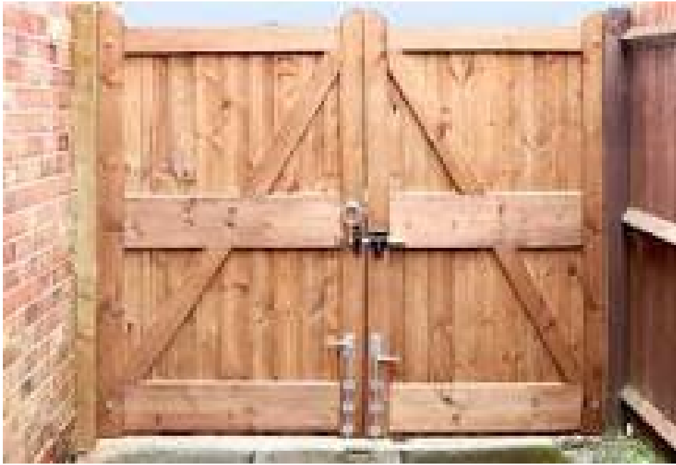
Detail of close boarded timber gates (rear view) to be positioned to north end of courtyard next to original Farmhouse
