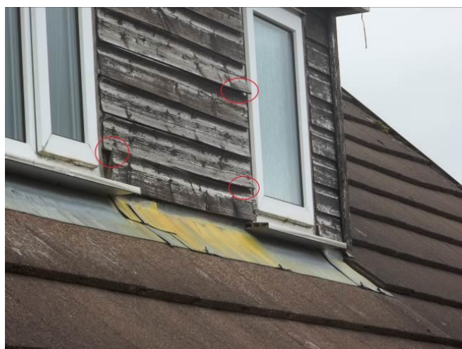
Gaps allowing bat access behind cladding highlighted in red
