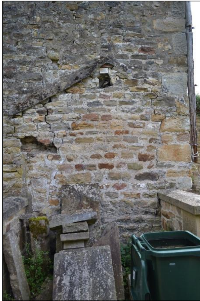
Plate 11. Detail of former porch
