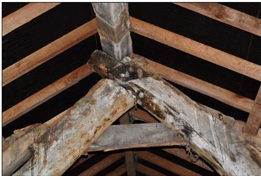
Plate 22. Showing pegs in cruck and ridge purlin
