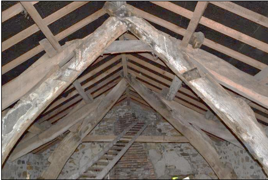
Plate 21. Detail of crucks and other roof timbers
