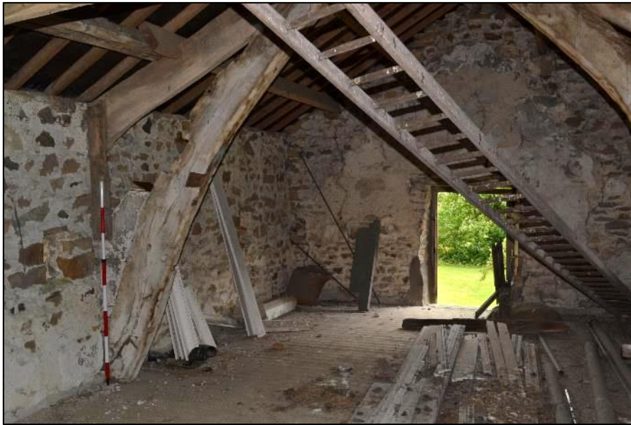
Plate 18. General shot first floor. Looking east (scale 1.6m)
