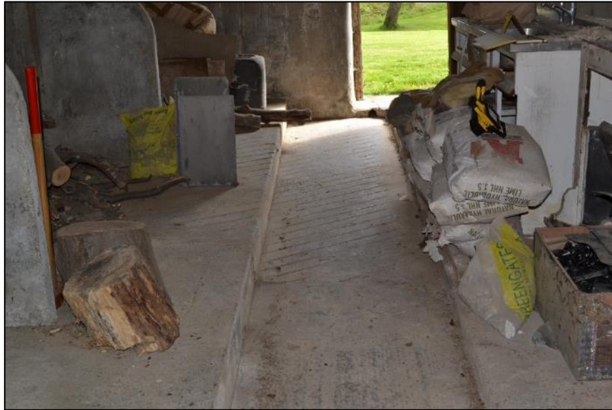
Plate 14. Ground floor, concrete dairy floor
