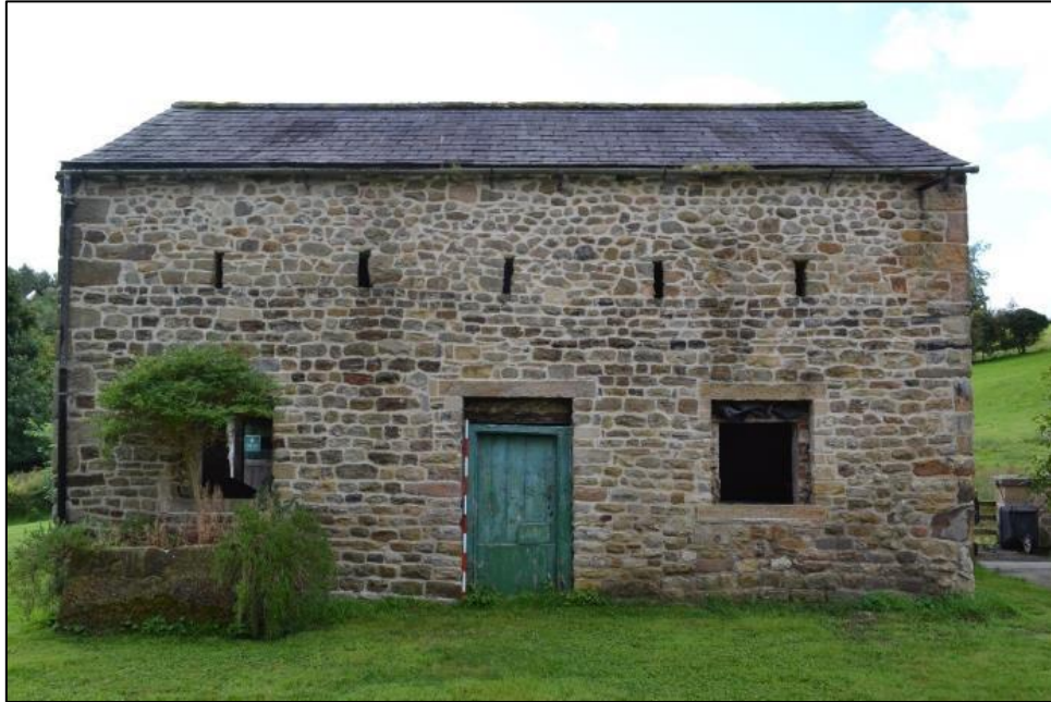
Plate 8. The north elevation (scale 2m)
