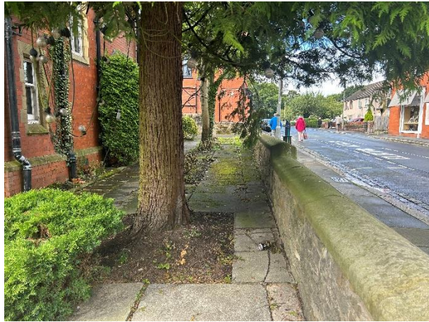
Photo 4: Existing wall on the George Street side of the building.
