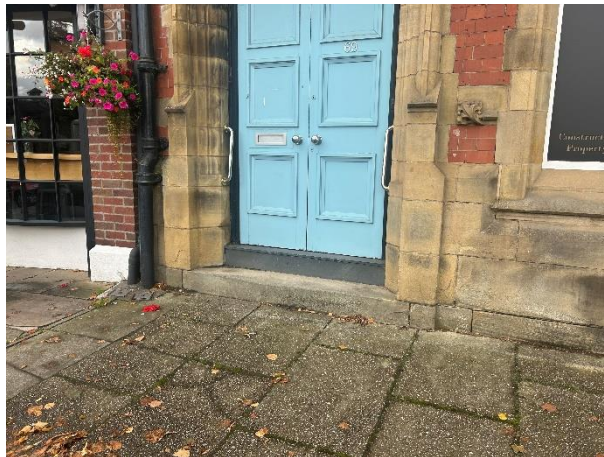
Photo 2: Existing front door on King Street with steps up from pavement.
