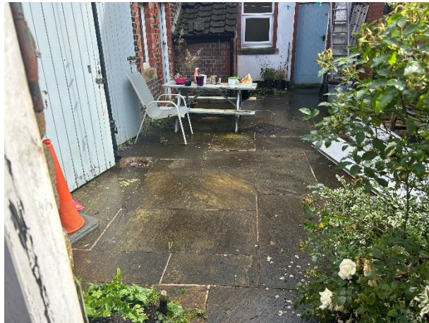
Photo 8: Rear of the building towards the outbuildings where the basement area is located.
