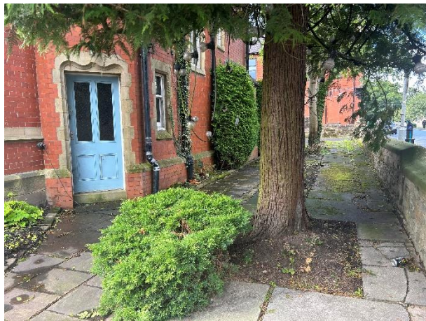
Photo 5: Side of building on George Street.
