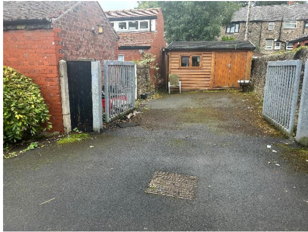
Photo 7: Rear of the building.
