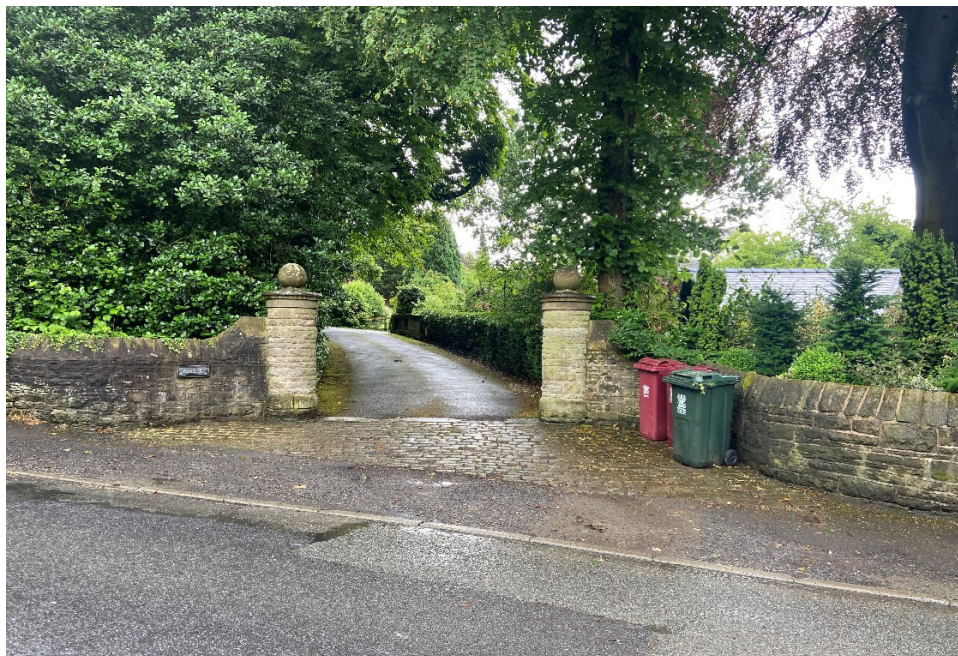
Figure 1 Existing Refuse Collection
