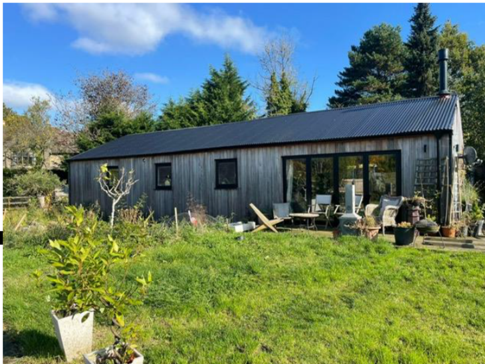
Figure 4 – Site Photograph of the dwelling
