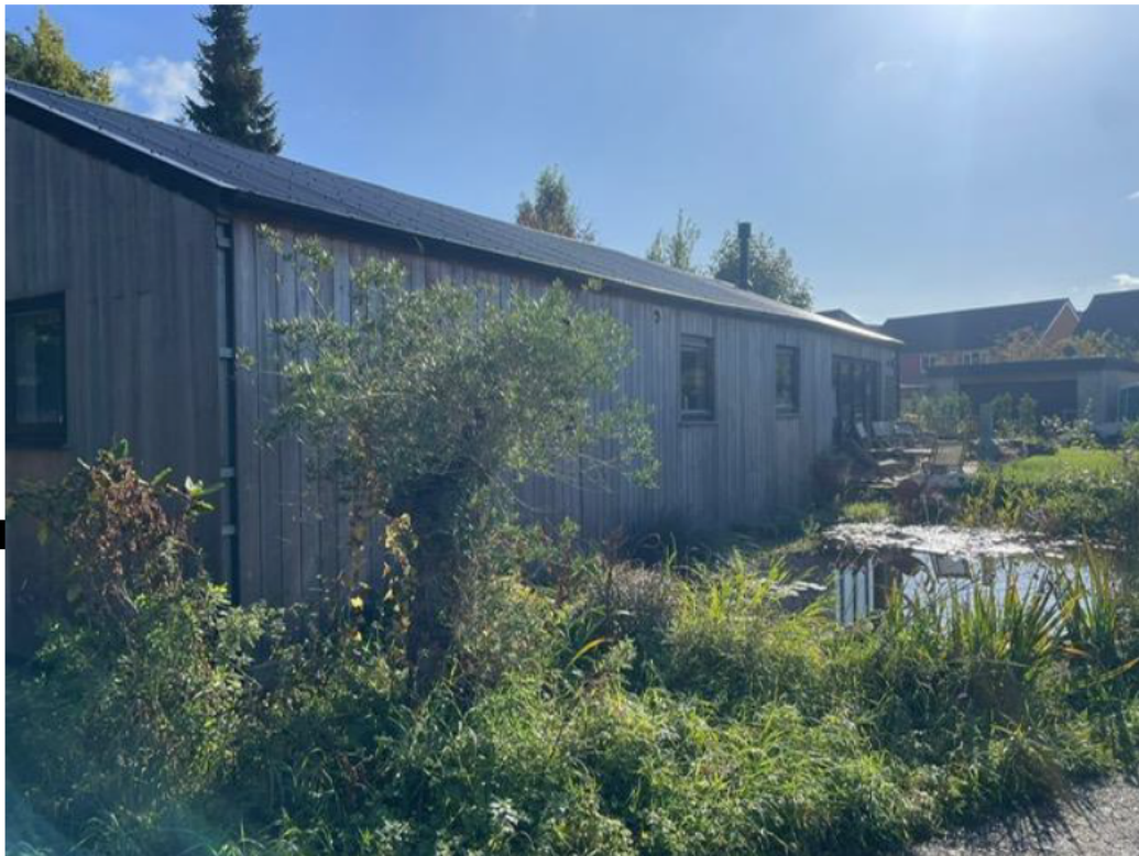
Figure 5 – Site Photograph of the dwelling
