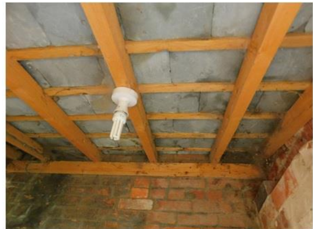
PHOTO 12 Underside of Outhouse Roof
