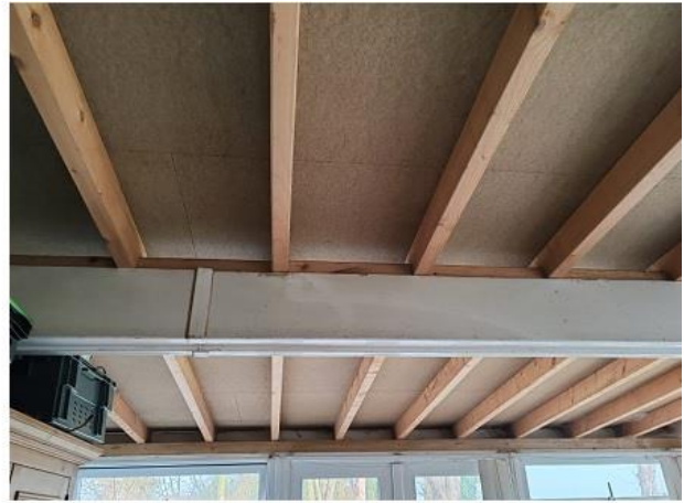
PHOTO 20 Underside of Extension Roof
