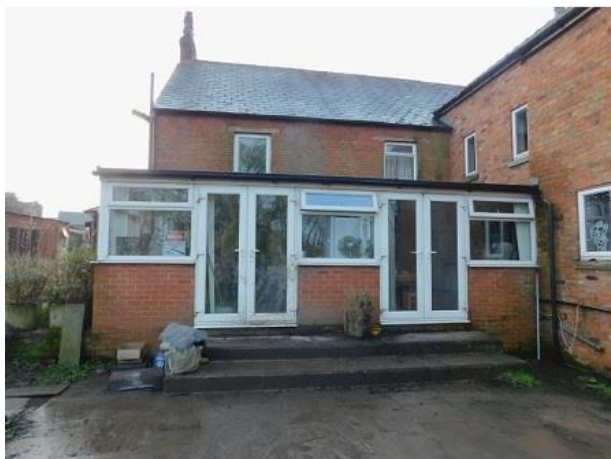
PHOTO 17 Northern Elevation of Extension
