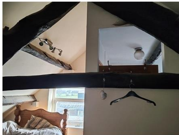
PHOTO 18 Underside of Central Ceiling
