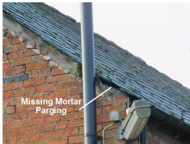
PHOTO 14 North-eastern Edge of Roof
