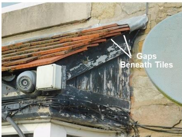
PHOTO 5 South-eastern Corner of Porch
