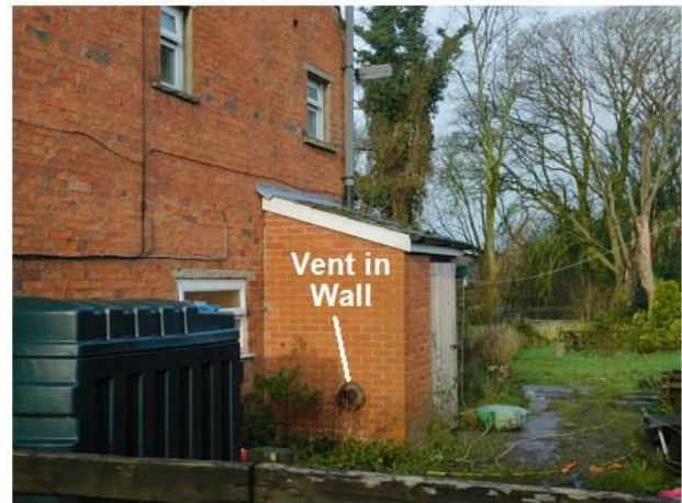
PHOTO 10 Southern Elevation of Outhouse
