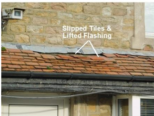
PHOTO 3 Part Central Southern Elevation
