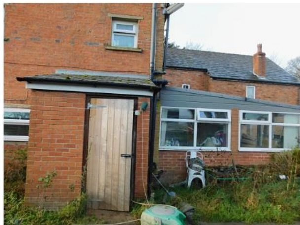
PHOTO 11 Eastern Elevation of Outhouse
