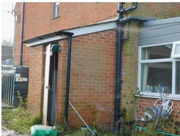
PHOTO 13 Northern Elevation of Outhouse
