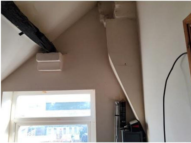
PHOTO 19 Underside of Eastern Part of Ceiling
