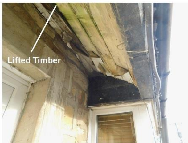
PHOTO 4 Underside of Southern Porch
