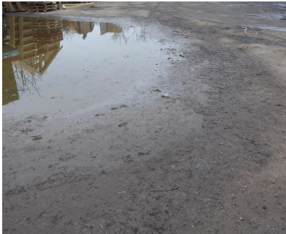
Urban sealed surface
