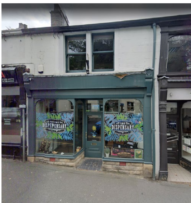
Fig 3. Existing "front" elevation, viewed from Moor Lane
