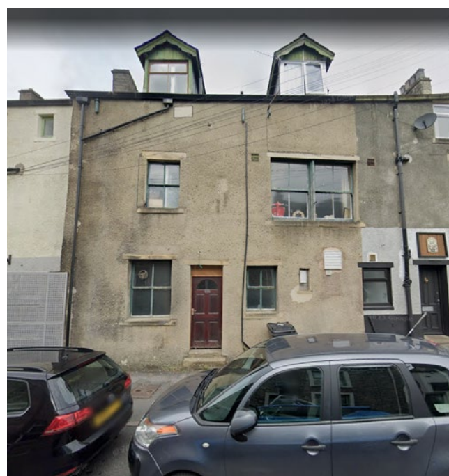
Fig 4. Existing "rear" elevation, viewed from Lowergate
