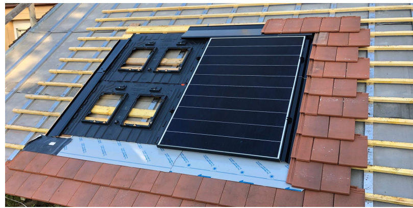
PV Roof Inset Detail
