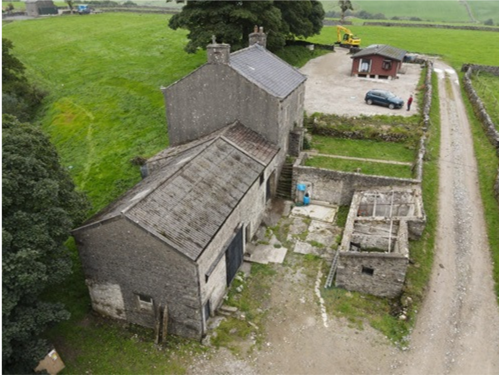
2. Aerial view from the west
