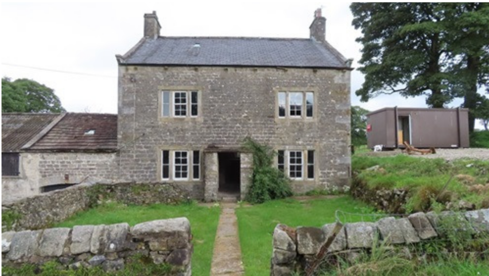
5. The front (south) elevation
