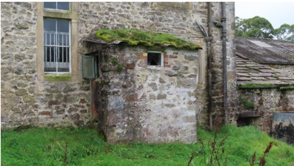
7. Improvised porch to north side
