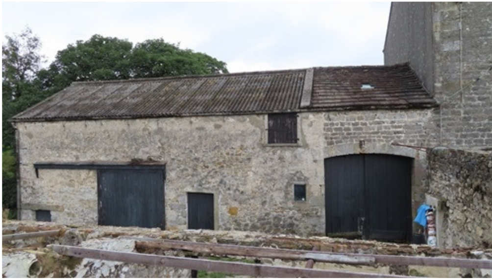
8. The south-facing trap house and barn; note that the masonry bonding of the house and trap house is continuous, indicating that they were built at the same time
