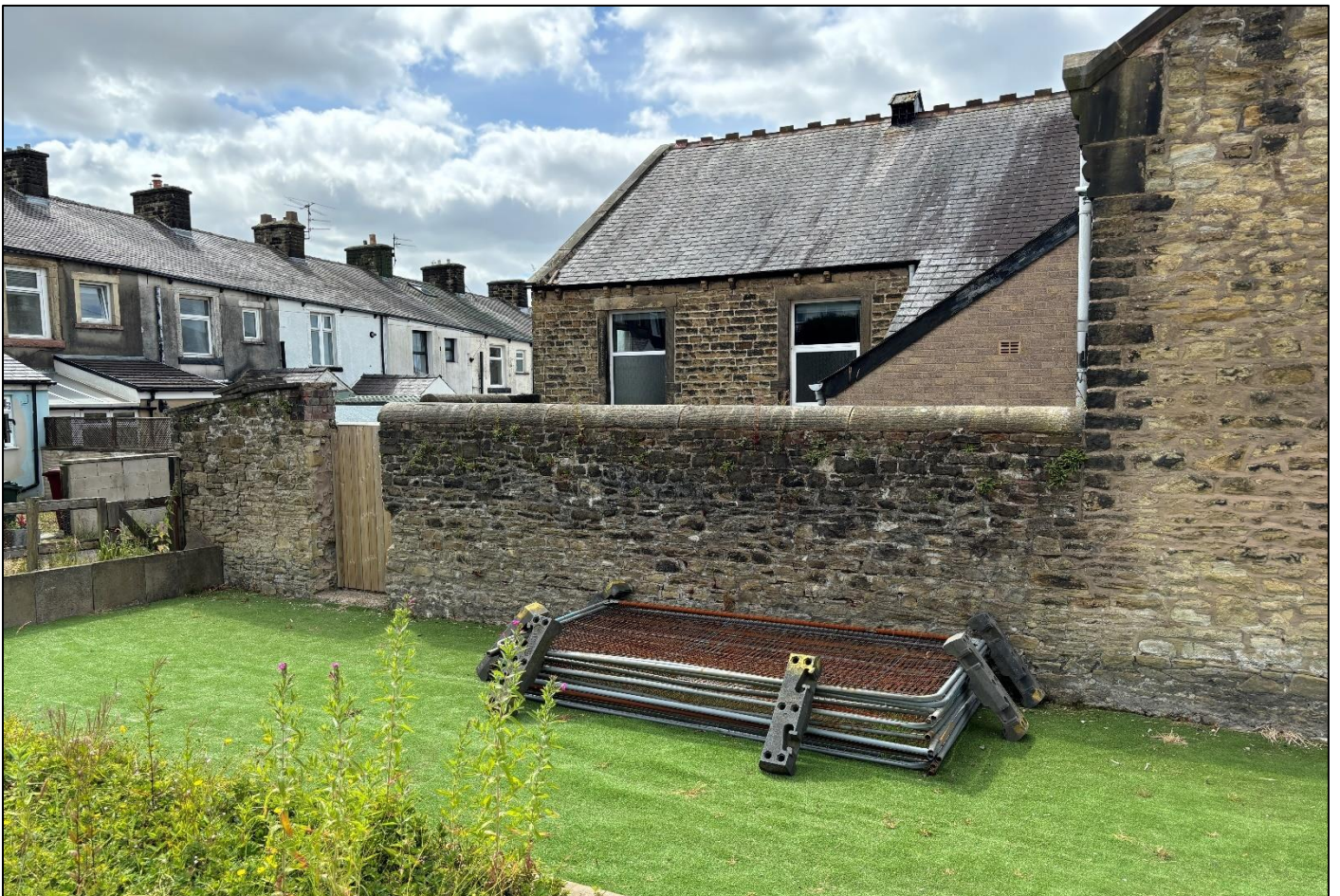
Fig 03: View towards the existing toilet block from the north.
