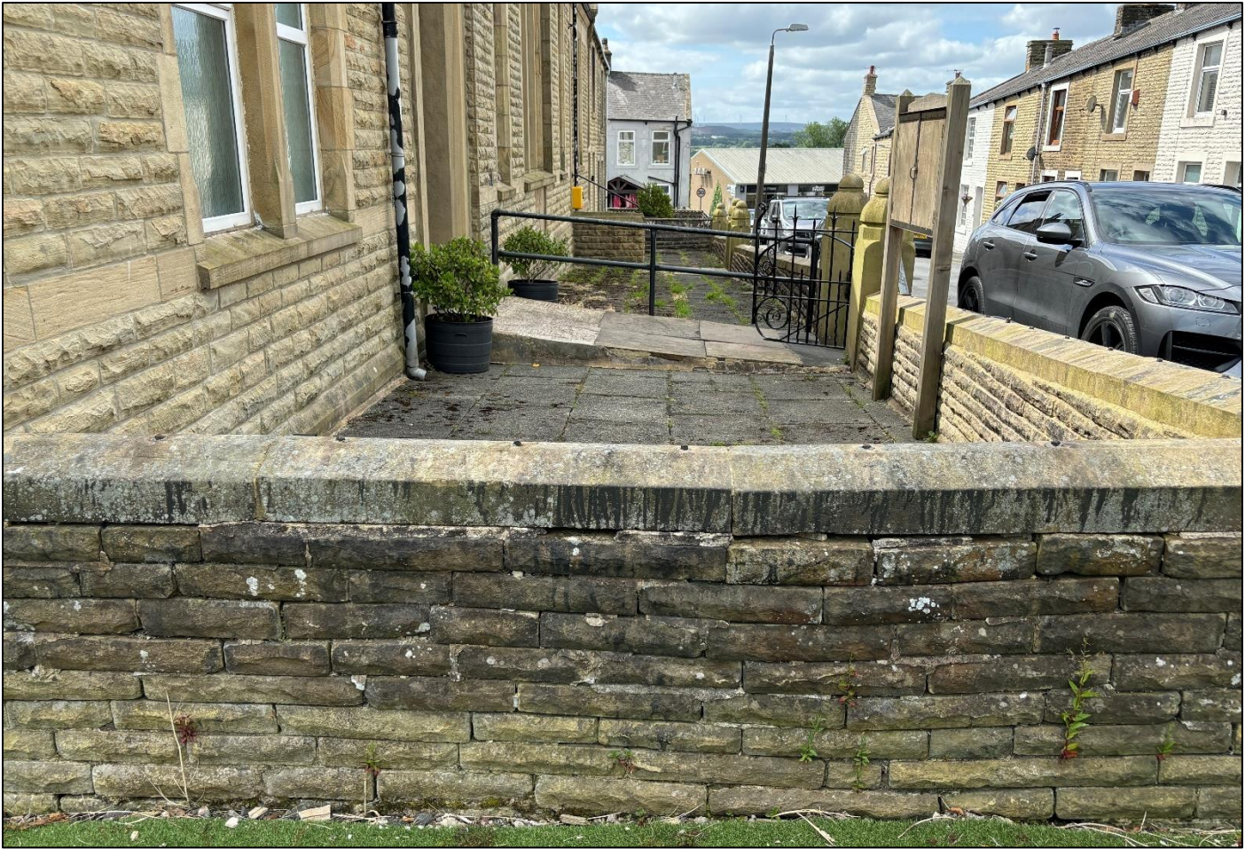
Fig 06: View of the location of the proposed building access ramp.
