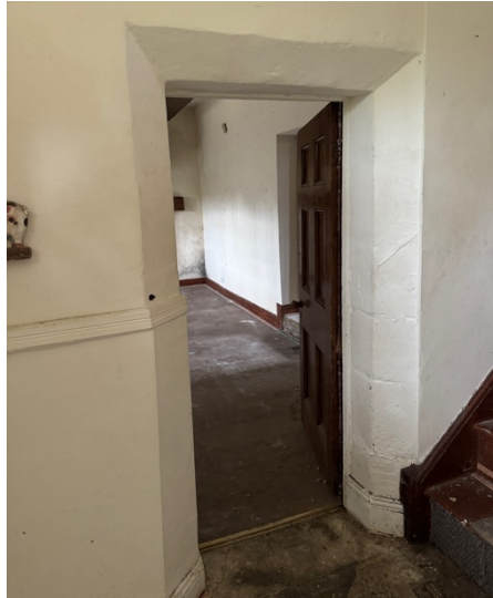
Figure 10: View of the chamfered internal doorways on the ground floor
