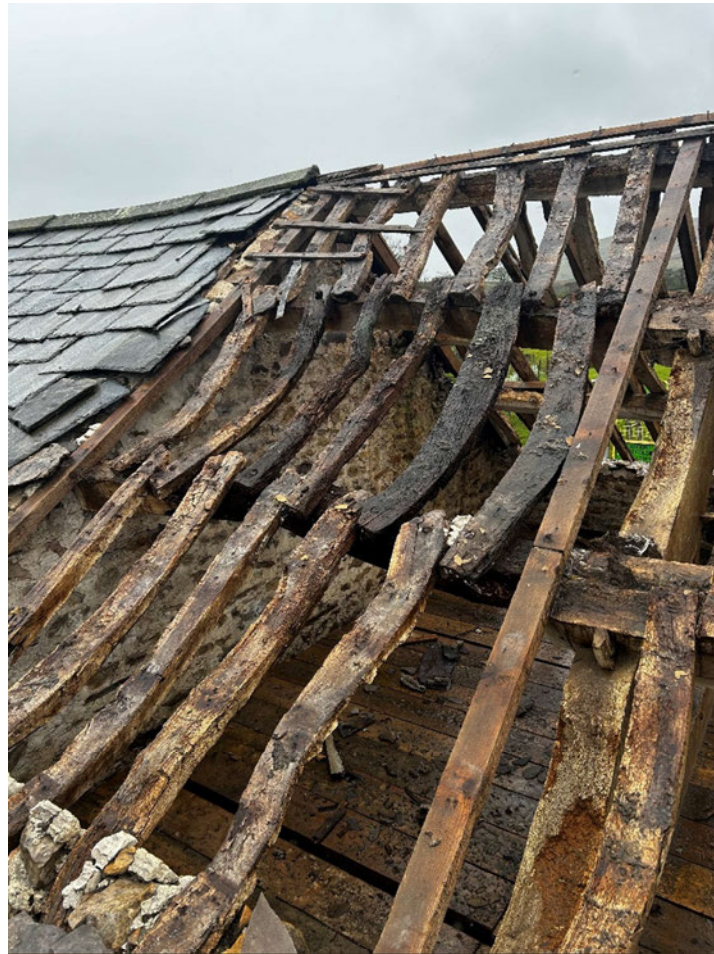
5. Original rafters in very poor condition
