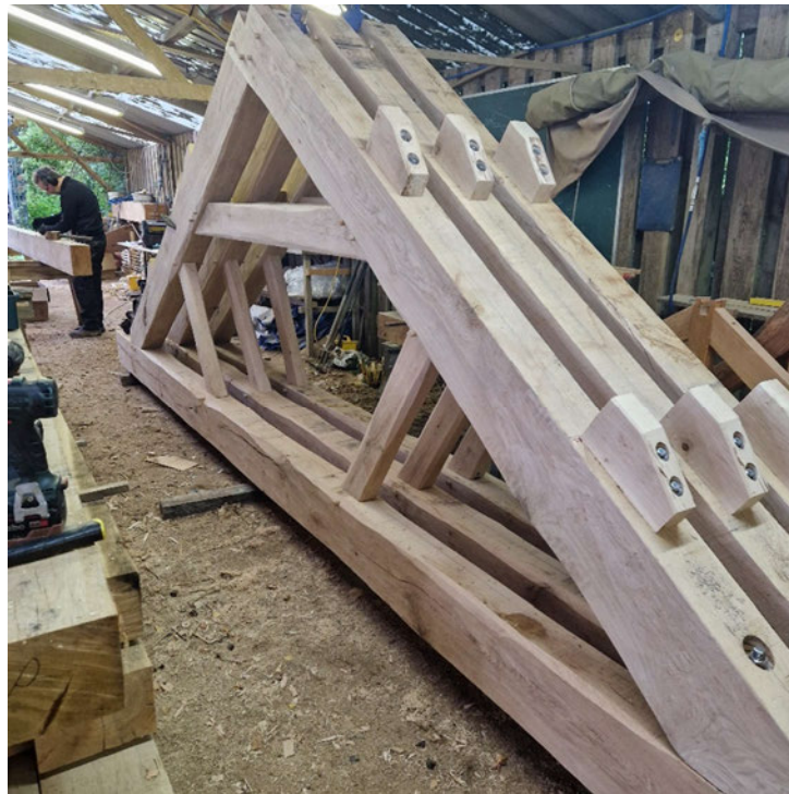
6. New trusses made to replicate old
