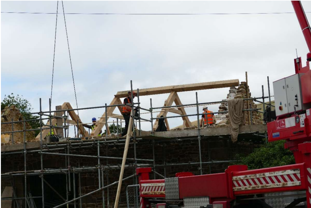
7. New trusses during installation
