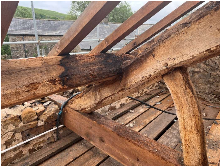
2. Rot and beetle attack to timbers
