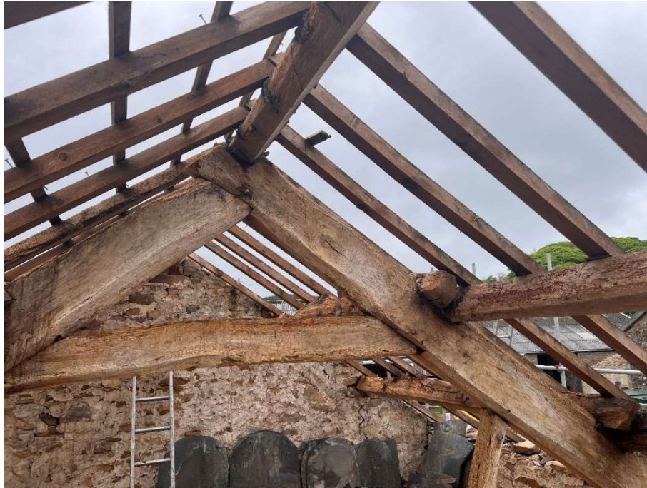
1. Details of existing trusses before removal
