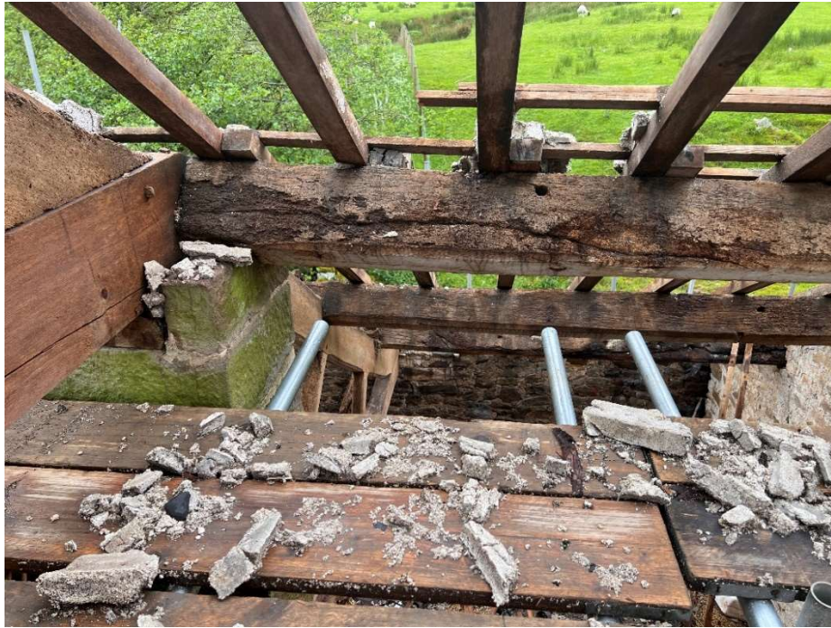
3. Significant rot to purlin on rear slope
