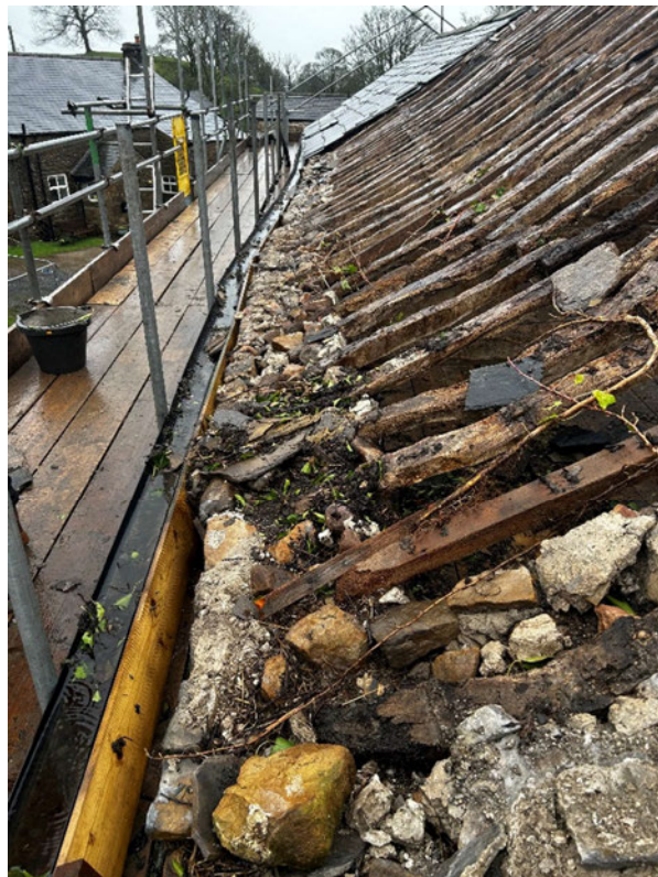
4. Rot visible to rafters
