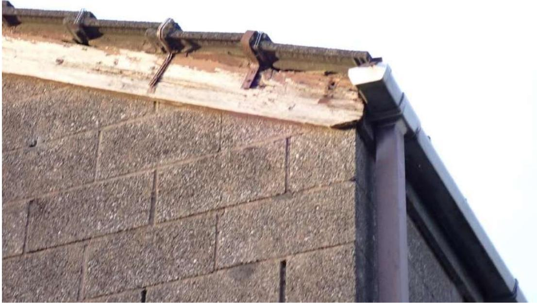
Photograph 5 – View of a damaged section of bargeboard on the western aspect of Building 1.
