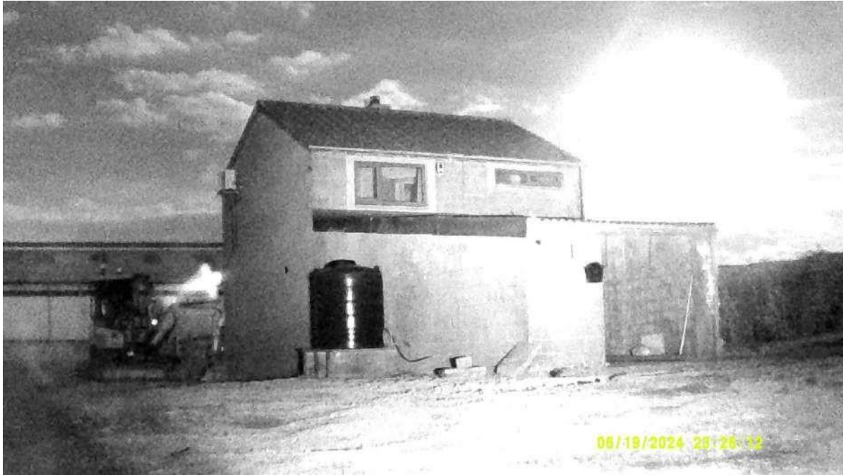
Photograph 1 – Infrared image of the northern aspect of Building 1 at the darkest point in the survey on the 19 th June 2024.
