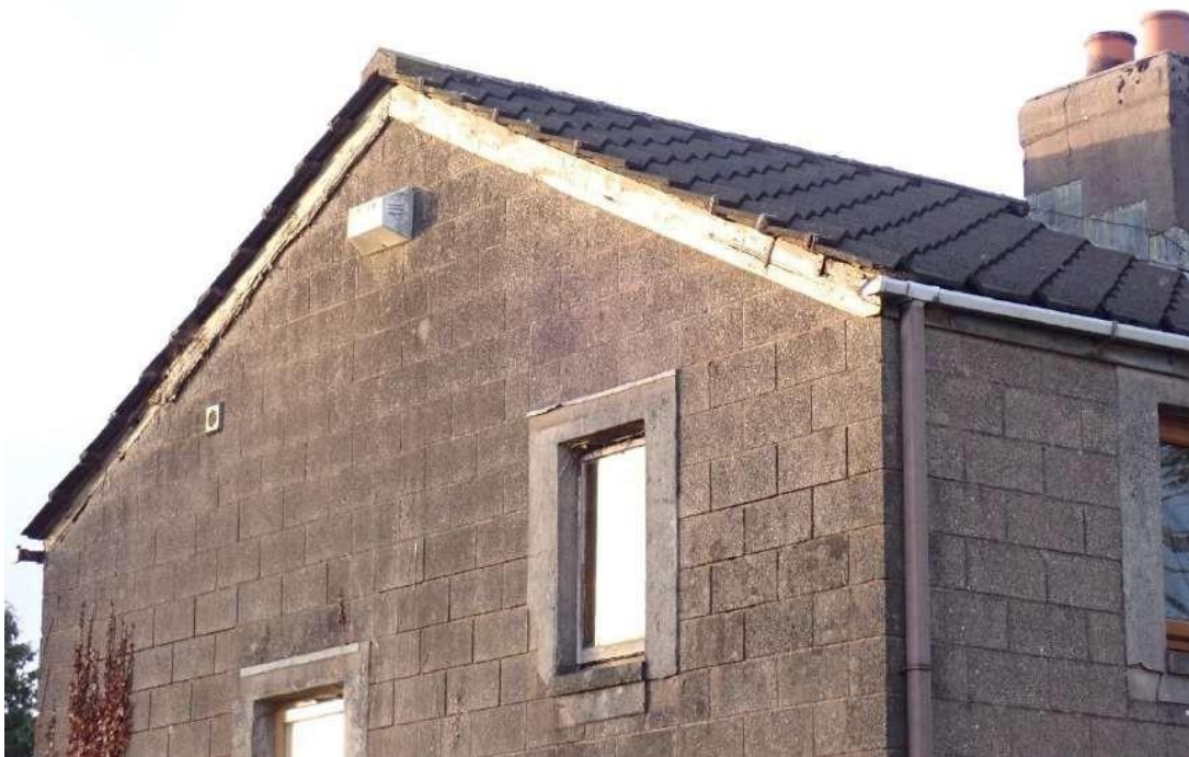
Photograph 2 – View of the pitched roof and western gable end of Building 1.
