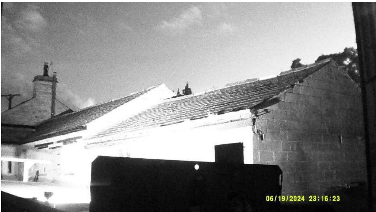
Photograph 4 – Infrared image of the eastern end of the southern aspect of Building 2 at the darkest point of the survey on the 19 th June 2024.
