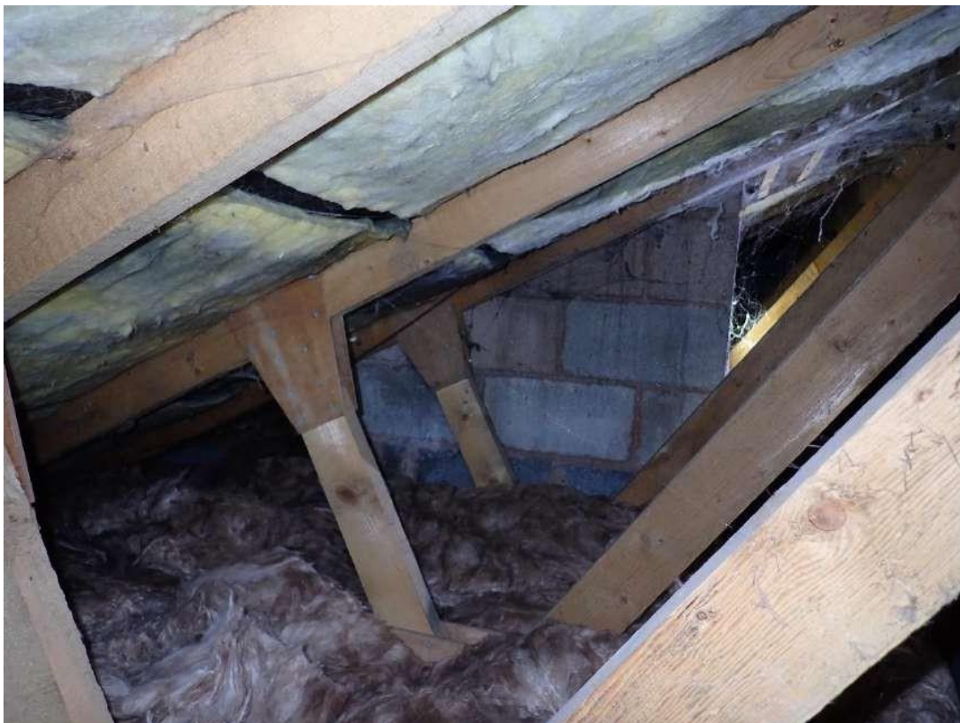
Photograph 34 - View of the single loft space located in Building 1.
