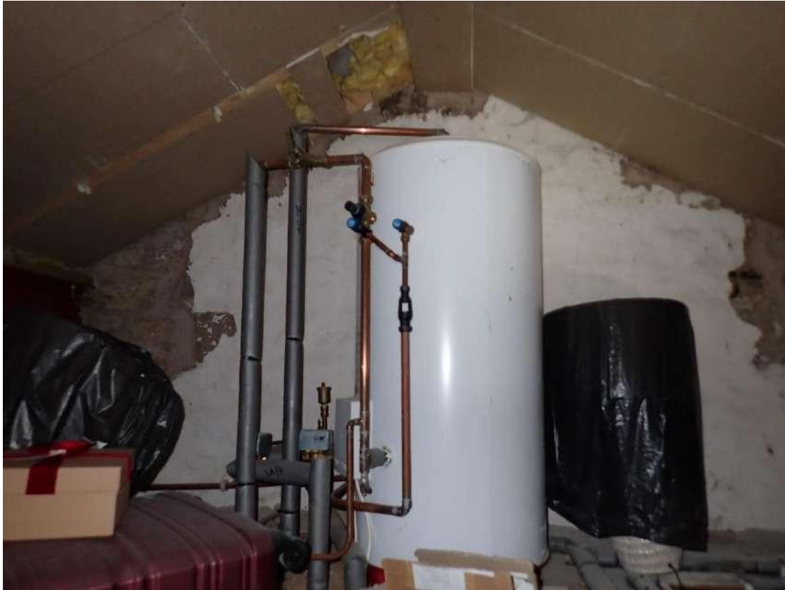
Photograph 37 – View of the interior loft insulation in the loft of Building 2.
