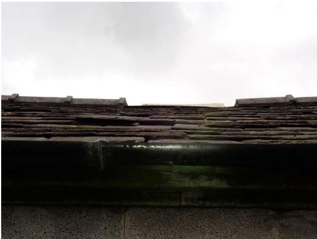
Photograph 12 - View of patches of raised roof tiles and missing ridge tiles on the roof of the eastern section of Building 2.
