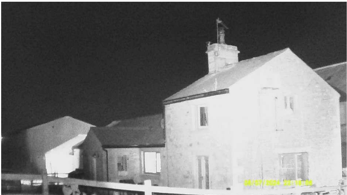
Photograph 8 – Infrared image of the eastern end of the northern aspect of Building 2 at the darkest point of the survey on the 7 th August 2024.
