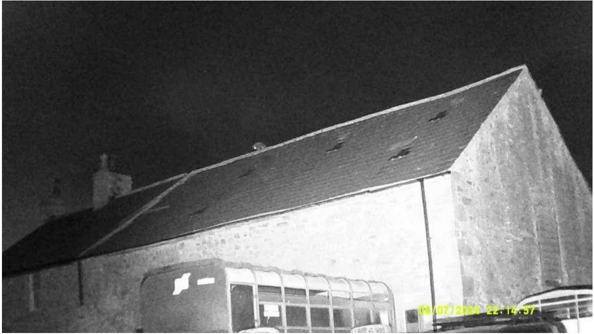
Photograph 11 – Infrared image of the eastern end of the southern aspect of Building 3 at the darkest point during the survey on the 7 th August 2024.
