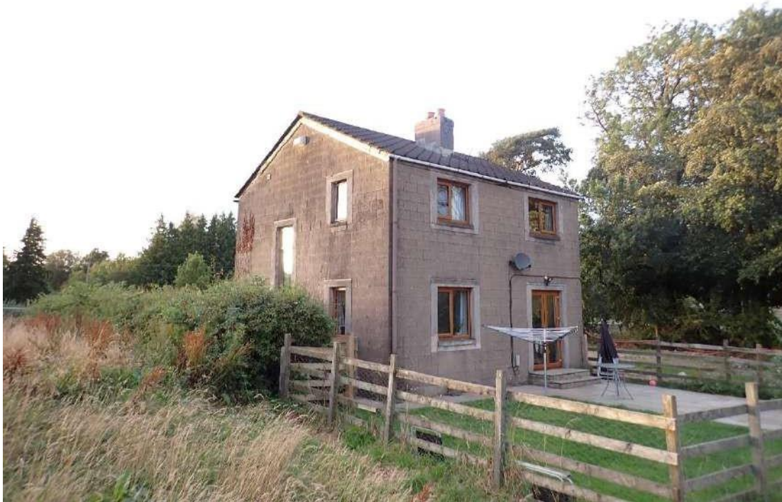
Photograph 1 – View of the southern aspect of Building 1.
