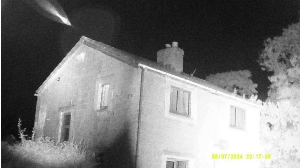
Photograph 7 – Infrared image of the southern aspect of Building 1 at the darkest point during the survey on the 7 th August 2024.
