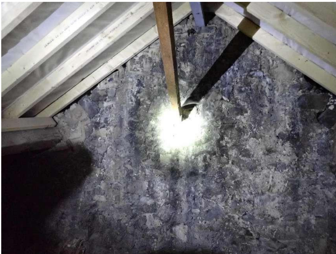
Photograph 54 – View of the numerous cracks and gaps in the internal walls allowing access to the wall cavity.
