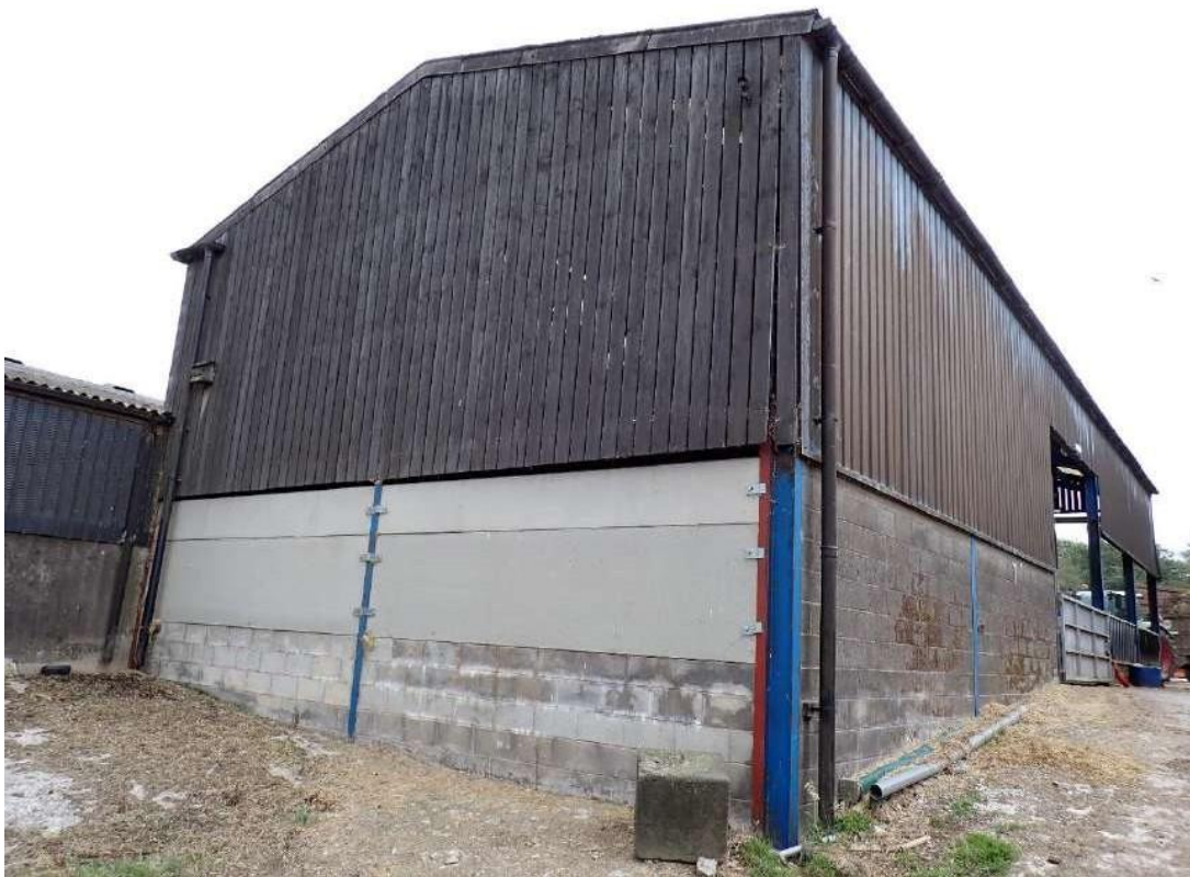
Photograph 32 - View of the gable end of Building 4.
