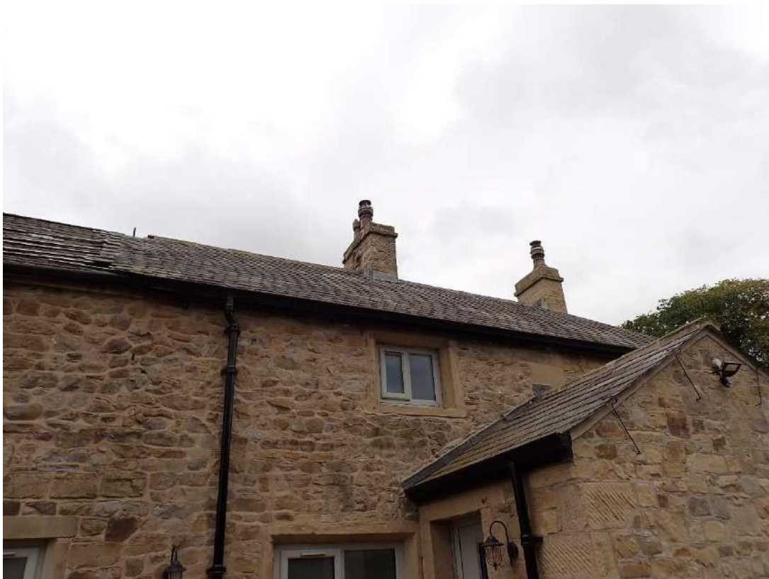
Photograph 30 – View of the porch on the northern aspect of Building 3.
