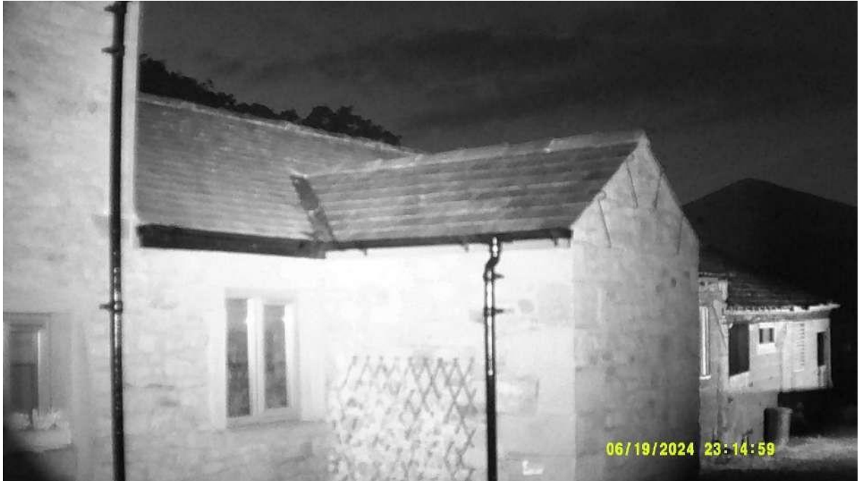
Photograph 3 – Infrared image of the western end of the southern aspect of Building 2 at the darkest point during the survey on the 19 th June 2024.
