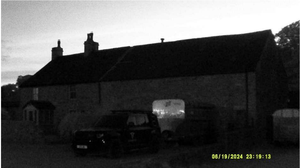
Photograph 5 – Infrared image of the southern aspect of Building 3 at the darkest point of the survey on the 19 th June 2024.
