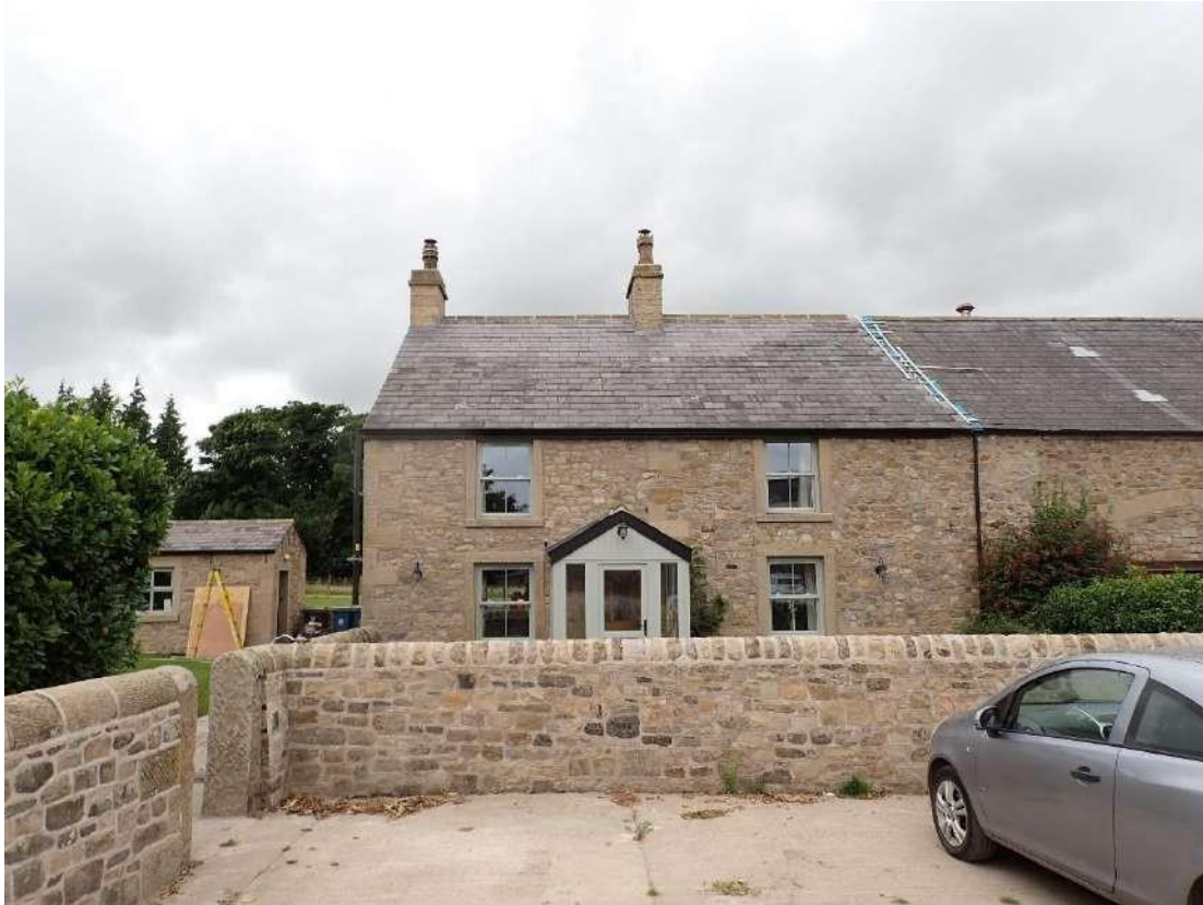
Photograph 31 - View of the porch on the southern aspect of Building 3.
