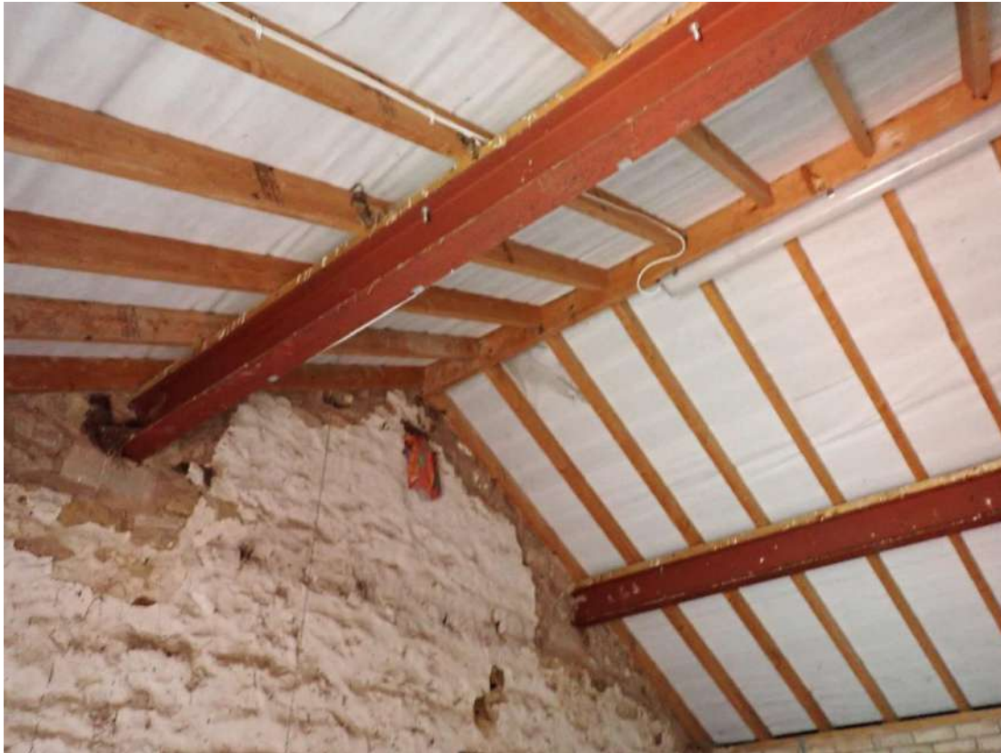
Photograph 39 – View of the underside of the roof in the western room of the pig styes in Building 2, showing the steel rafters and the breathable membrane lining.
