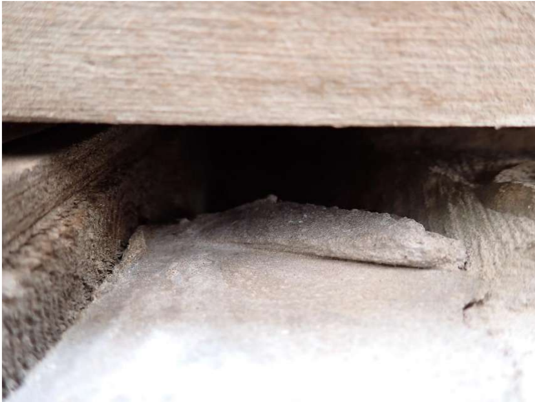
Photograph 25 – View of the cavity extending up to the wall plate, located behind the fascia board on the southern aspect of Building 3.
