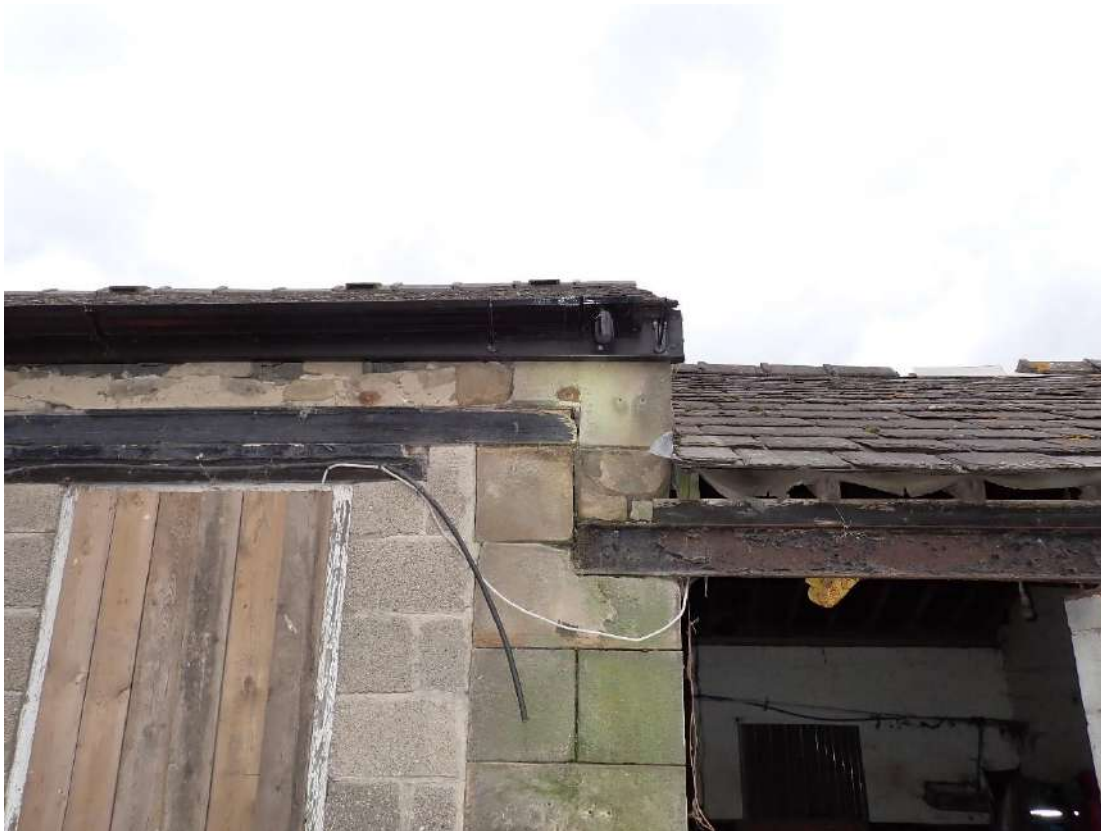
Photograph 17 – View of gaps in the brickwork on the southern aspect of Building 2.
