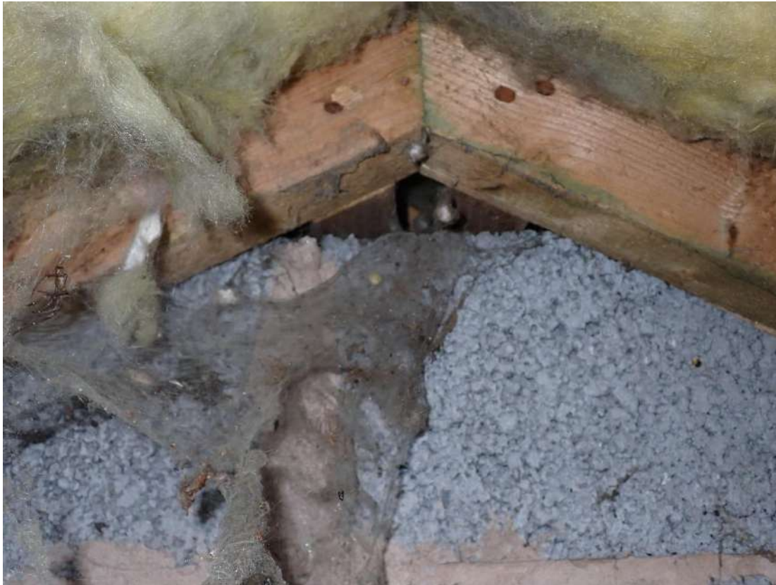
Photograph 35 - View of the gaps in the interior walls which allow access to the wall cavities.
