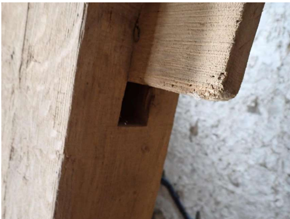
Photograph 58 – View of a PRF in the form of a gap around mortice joints in the wooden beams in the barn section of Building 3.
