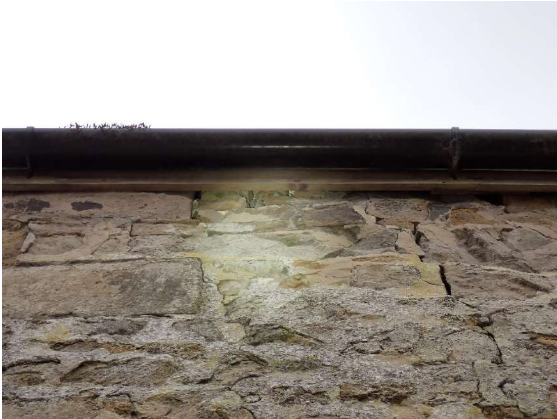
Photograph 13 – View of access points into Building 2 formed from missing mortar behind the fascia boards.
