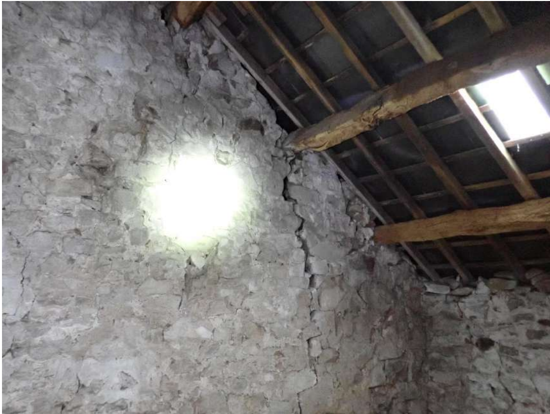
Photograph 61 - View of the cracks in the gable end and missing mortar at the wall plates in the barn section of Building 3.
