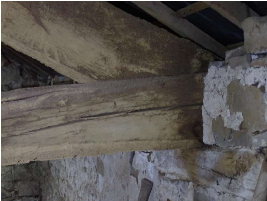
Photograph 60 – View of a PRF formed from cracks in the timber beams in the barn section of Building 3.
