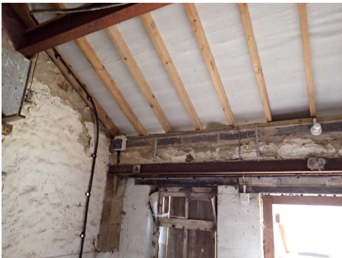
Photograph 41 - View of the gaps above the wall plate in the western room of the pig styes of Building 2.
