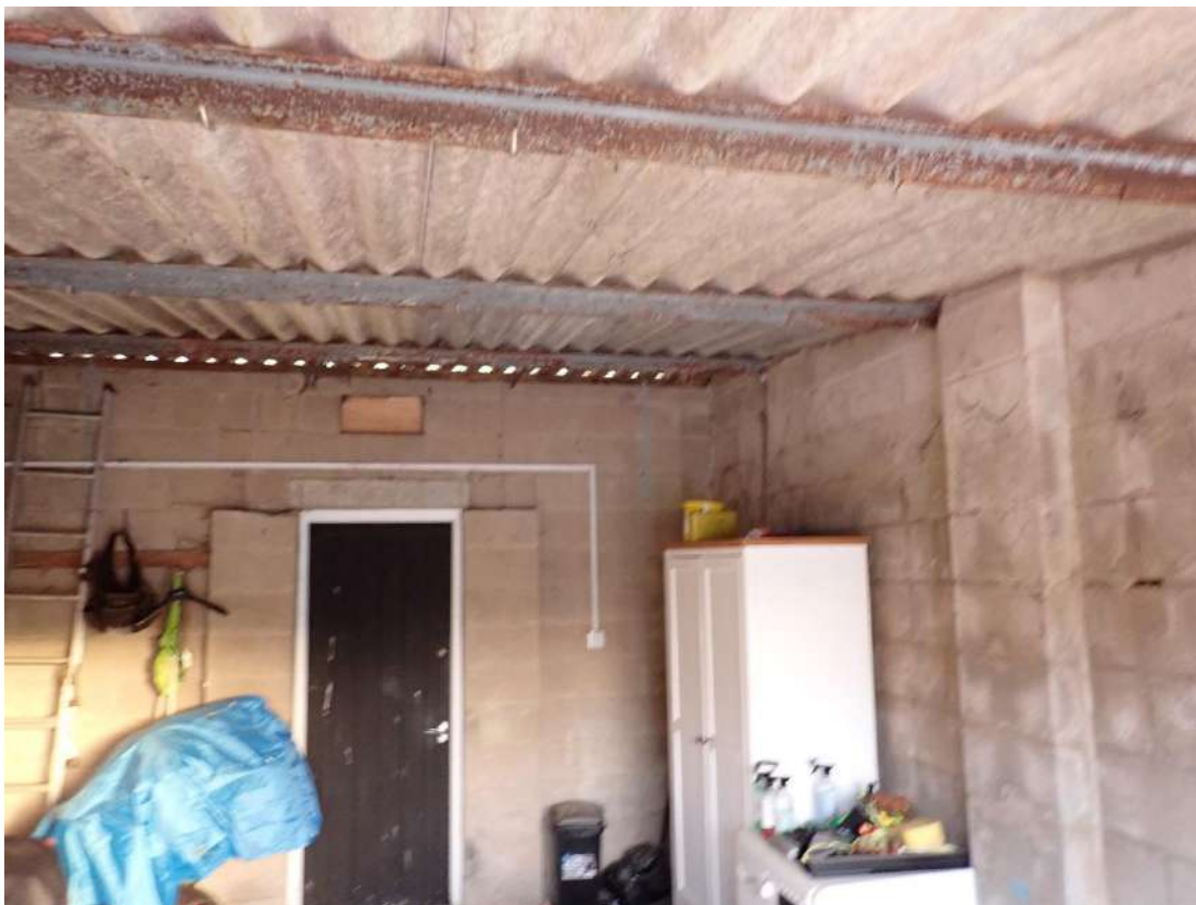
Photograph 8 – Internal view of the gaps behind the fascia boards in the garage attached to Building 1.
