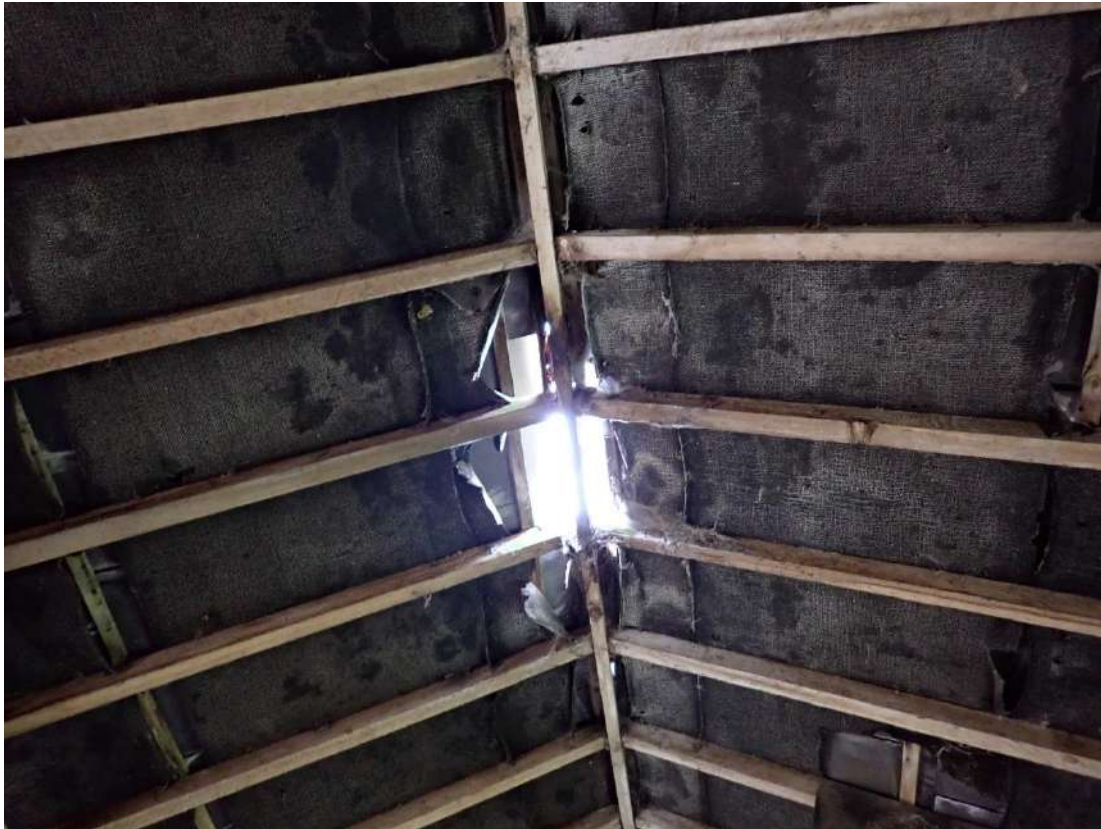
Photograph 45 – View of the damaged bitumen lining in the eastern room of the pig sty section of Building 2.
