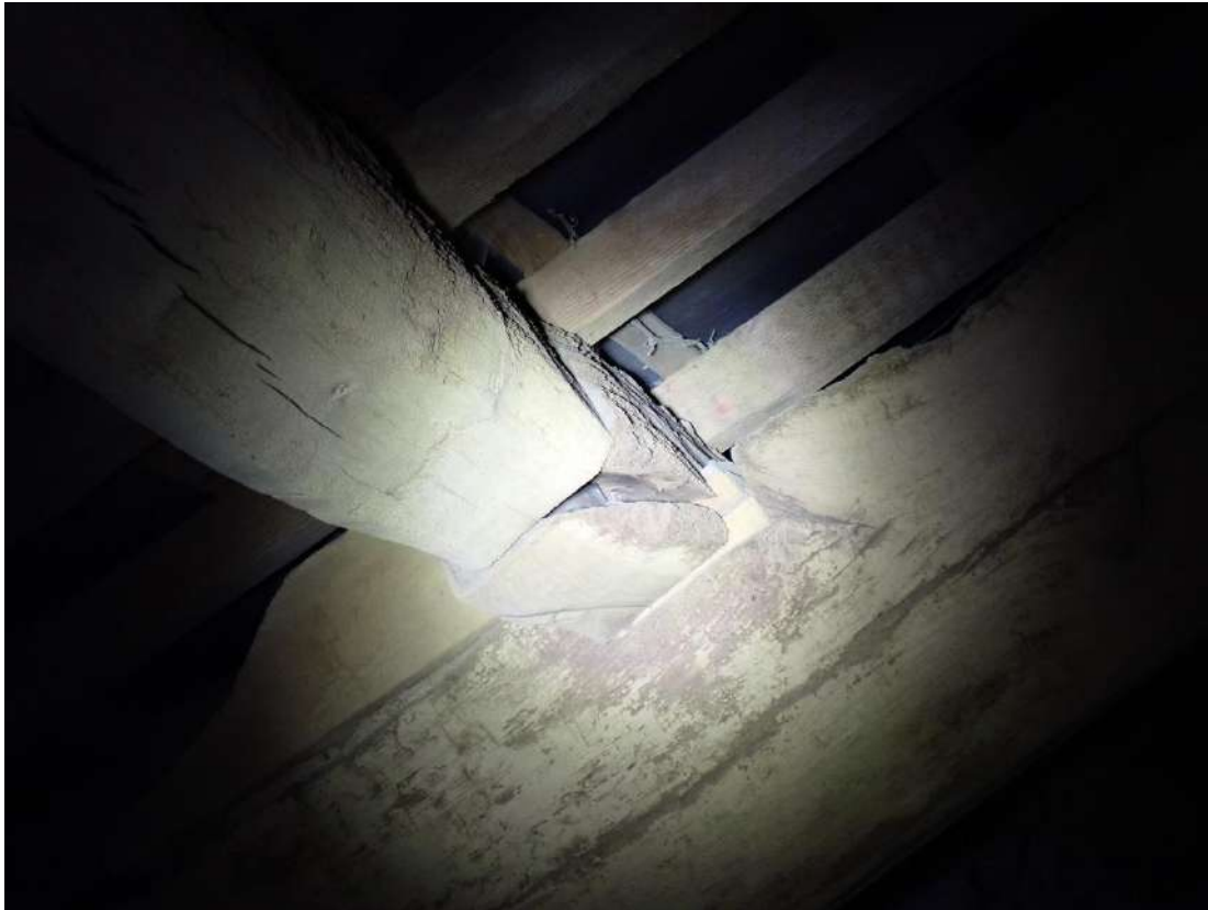
Photograph 59 – View of a PRF formed by ill-fitting joints in the timber structure of the barn section of Building 3.
