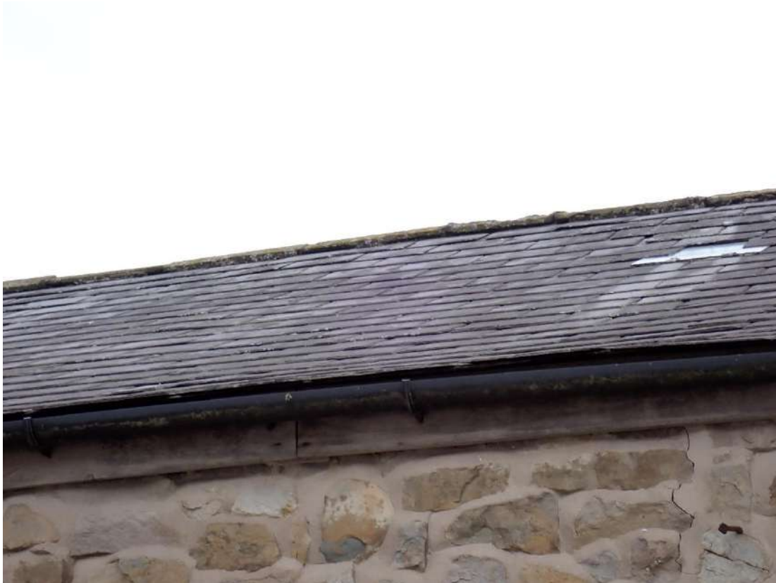
Photograph 23 – View of the gaps behind the fascia board on the southern aspect of Building 3.
