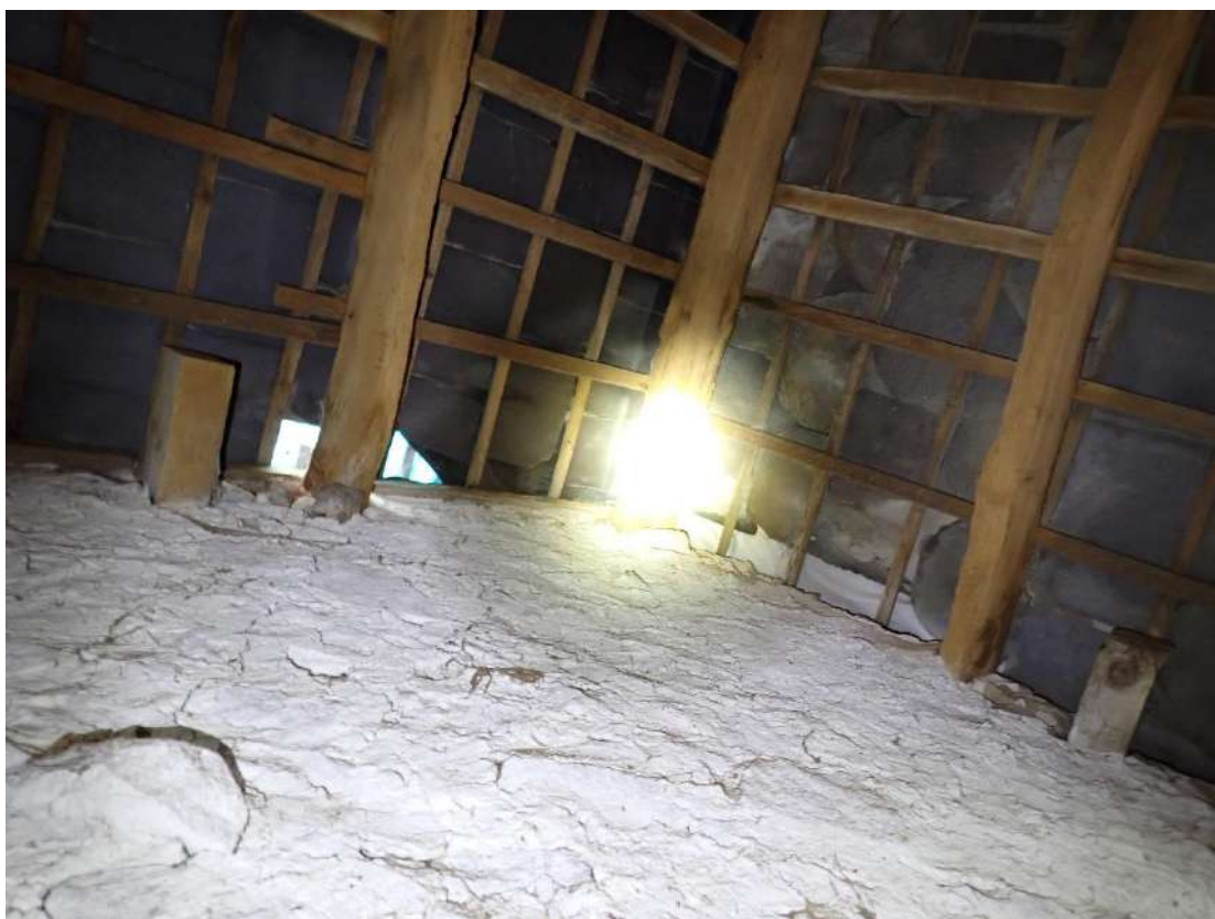
Photograph 57 – View of the underside of the roof of the barn section of Building 3, showing gaps in the tiles and an absence of lining.
