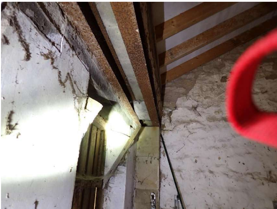
Photograph 14 - View of the wood and metal joists which comprise the eaves of the eastern section of Building 2.
