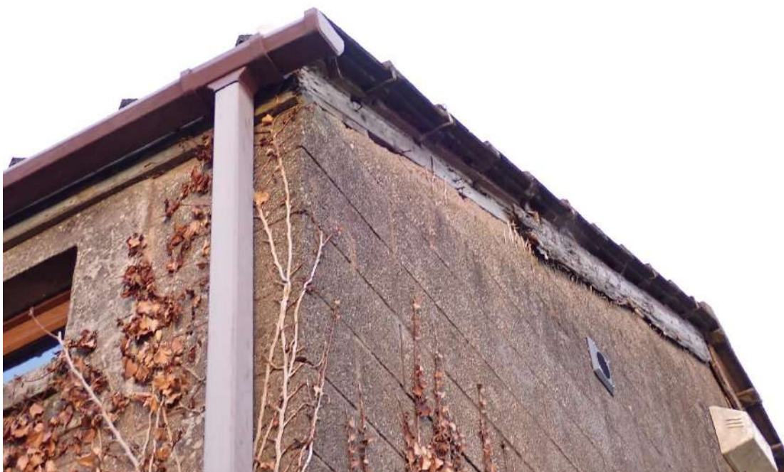
Photograph 6 - View of a missing section of bargeboard on the western aspect of Building 1.
