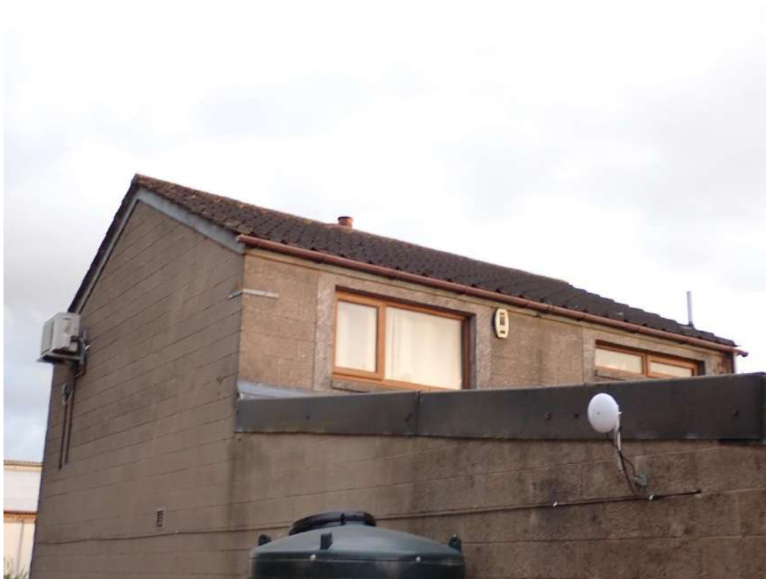
Building 9 – View of the lead flashing where the garage attaches to Building 1.
