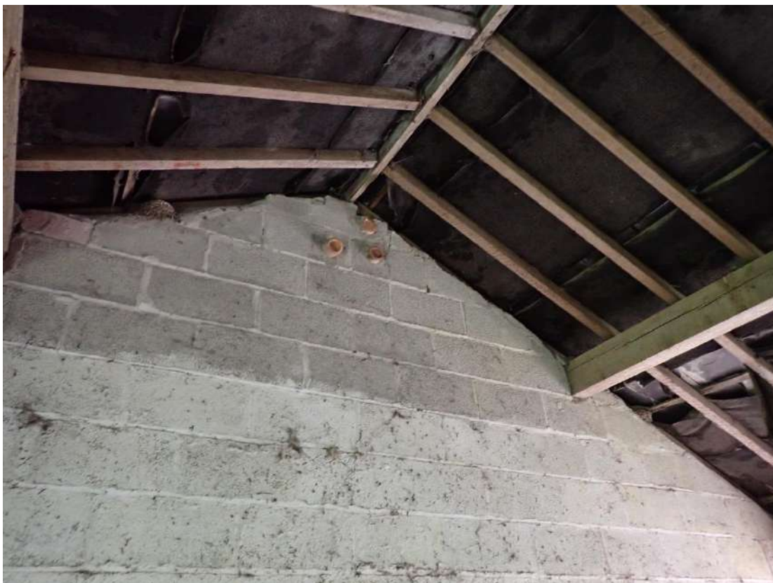
Photograph 46 - View of the damaged sections of the brickwork in the internal walls of the pig sty section of Building 2 leading to the wall cavity.
