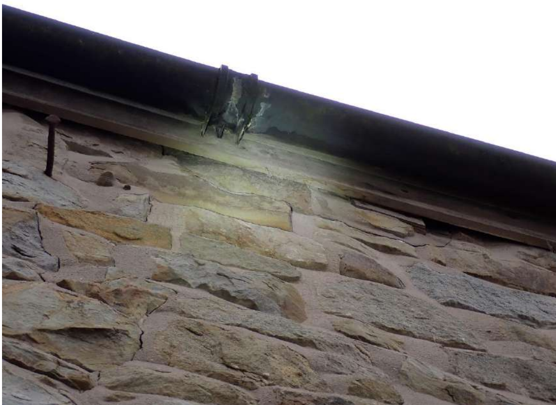
Photograph 24 – Close in view of the gaps between the fascia boards on the southern aspect of Building 3.
