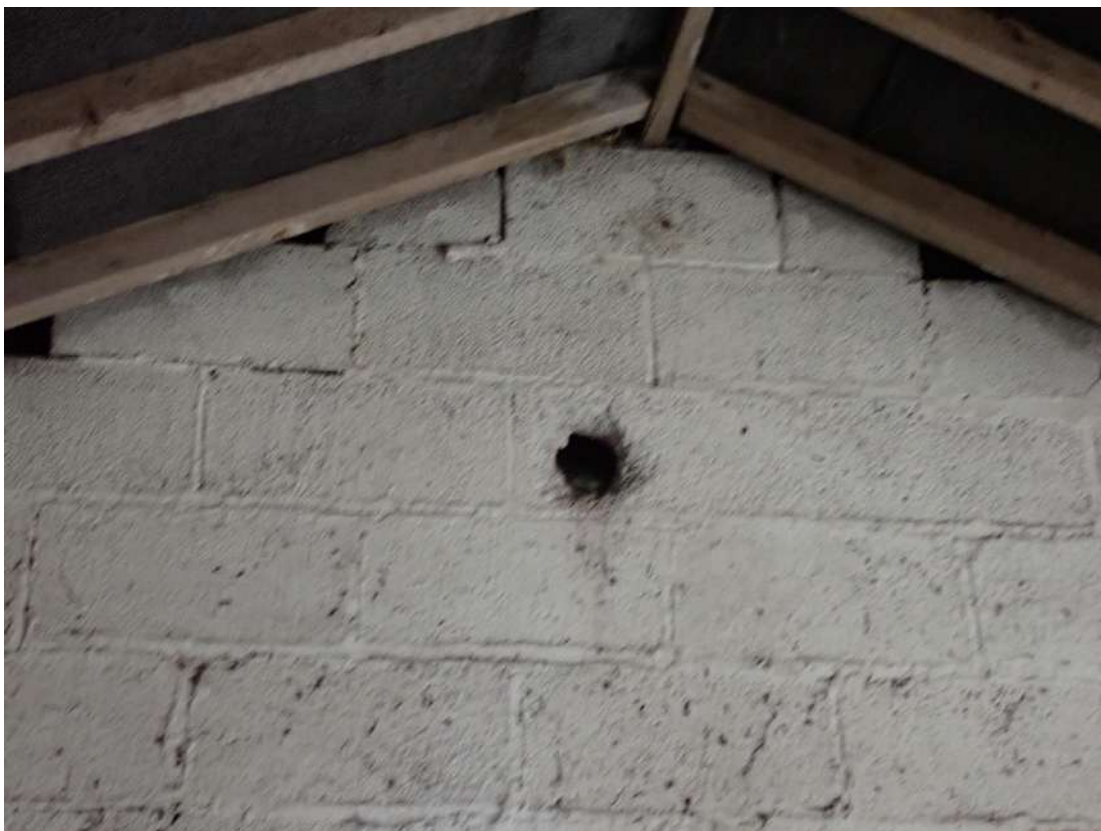
Photograph 48 – View of a hole in the breezeblocks at the gable end leading to the wall cavity in the eastern room of the pig sty section of Building 2.
