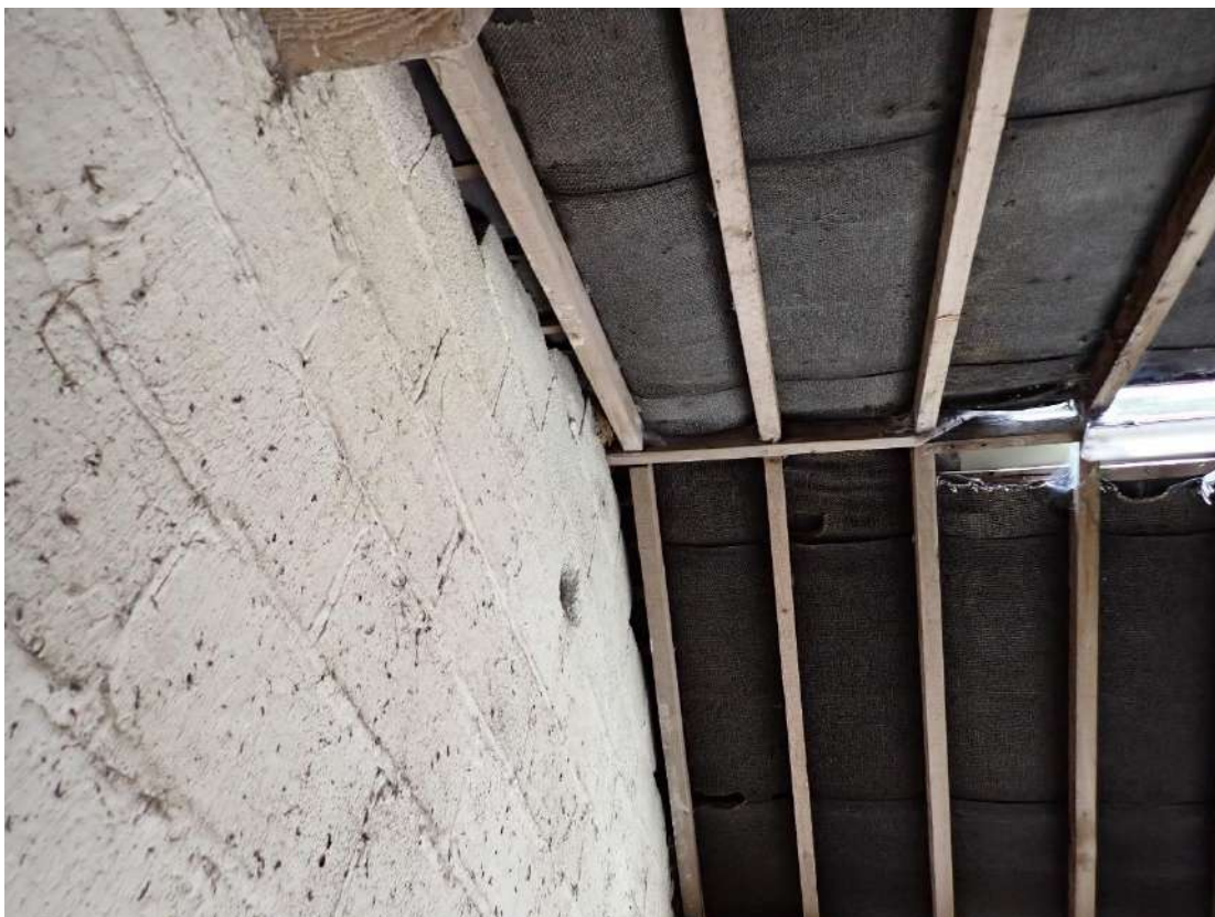
Photograph 44 – View of the gaps between the tiles and the bitumen lining forming PRFs in the middle room of the pig sty section of Building 2.
