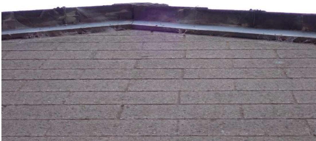
Photograph 4 – View of the gaps under the bargeboards on the eastern aspect of Building 1.
