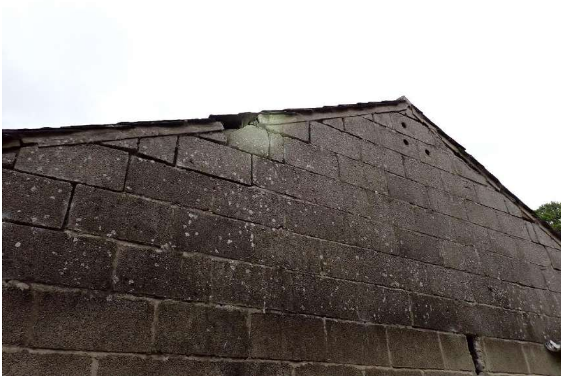
Photograph 15 – View of access points into the wall cavities of Building 2 via areas of damaged brickwork at the eastern gable end.
