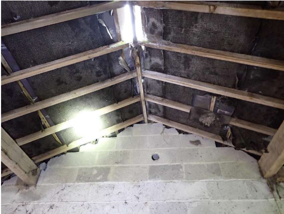
Photograph 43 - View of the damaged section of the bitumen lining of the middle room of the pig styes in Building 2.
