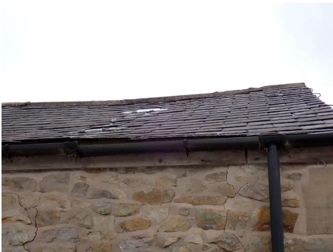
Photograph 21 - View of the raised tiles on the southern aspect of Building 3, forming PRFs.
