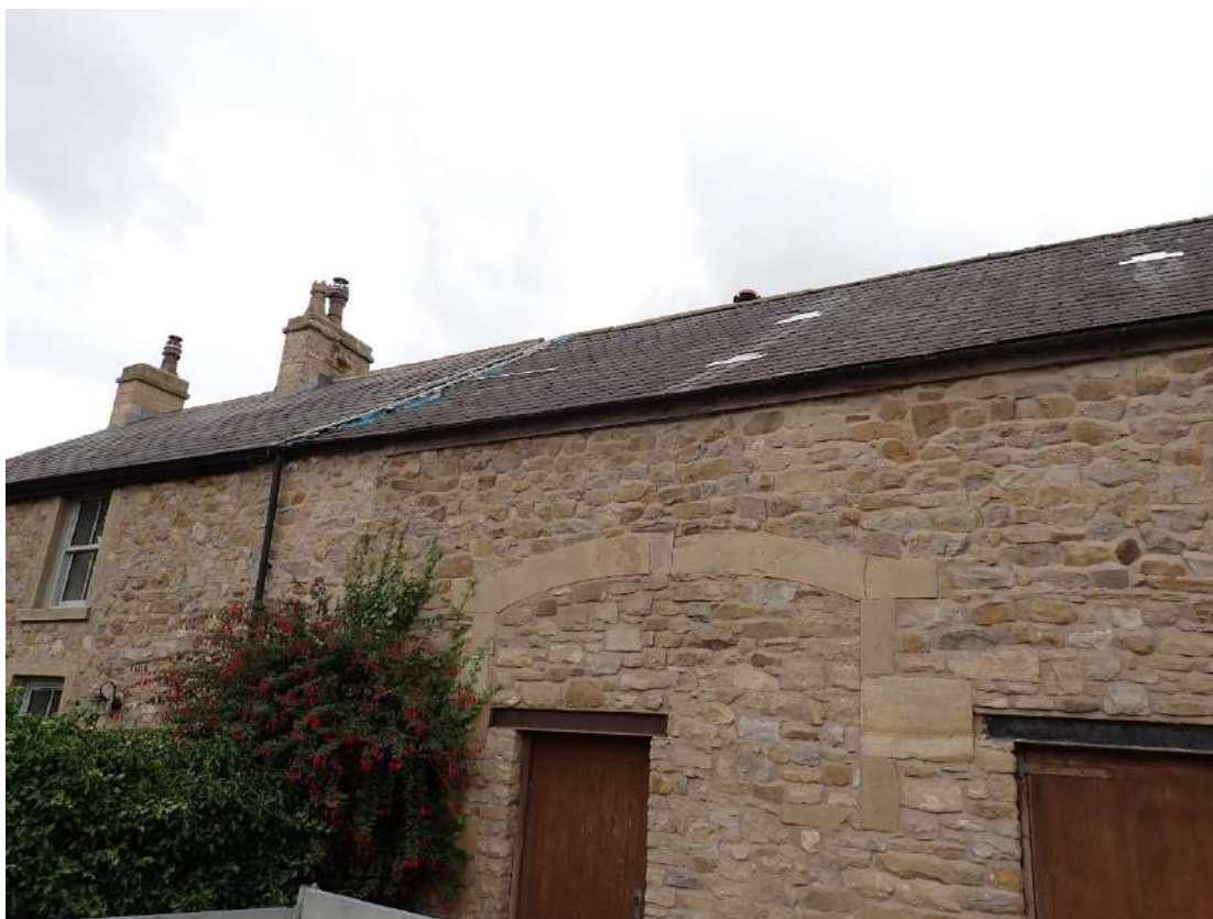
Photograph 22 – View of the southern aspect of Building 3 and the flashing around the chimneys and the skylights which is in good condition.
