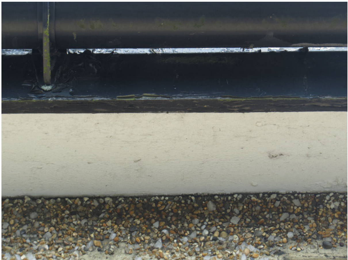
4 – Timber fascia boards and soffits at the eaves are fixed tightly against brickwork.
