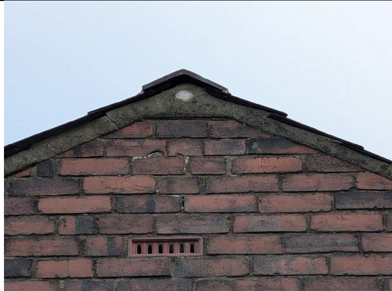
Photo 5. Roof verge and pointing on rear elevation.
