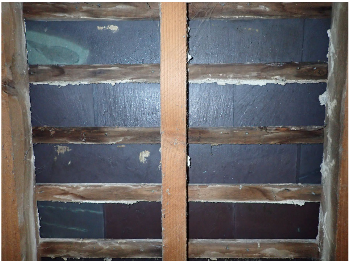
10 – The roof is not lined, tiles are in good condition with no gaps.
