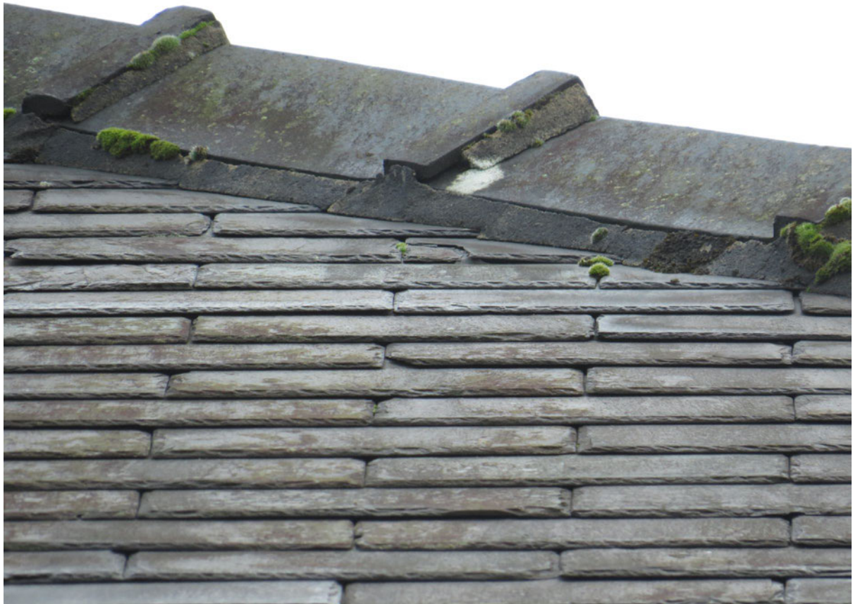
3 – Roof and ridge tiles are in good condition with no suitable gaps.
