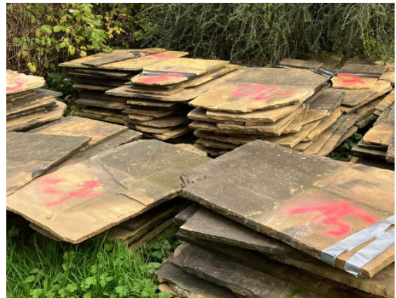
Removed slates fully recorded in order
