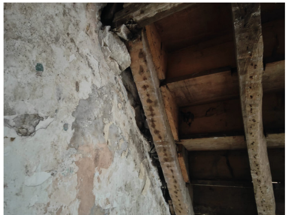
Boron-based preservative treatment to timbers while drying
