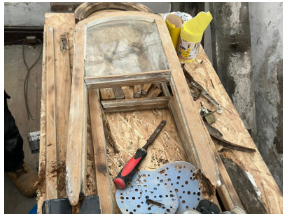
Main window frames retained and refurbished
