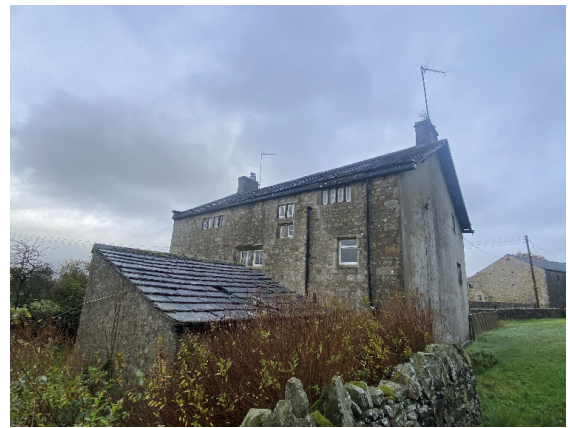
Farmhouse West Elevation
