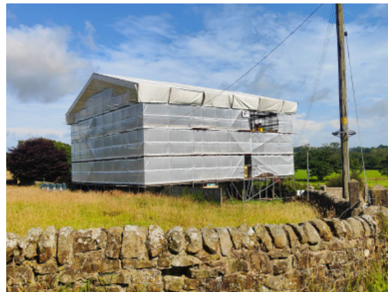
Weather Protection for Drying Out
