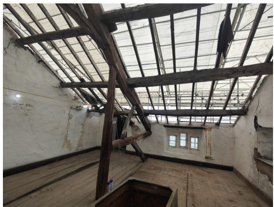
Refurbishing and repairing the frame for longevity
