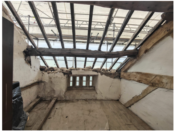
Existing Oak Purlins Retained
