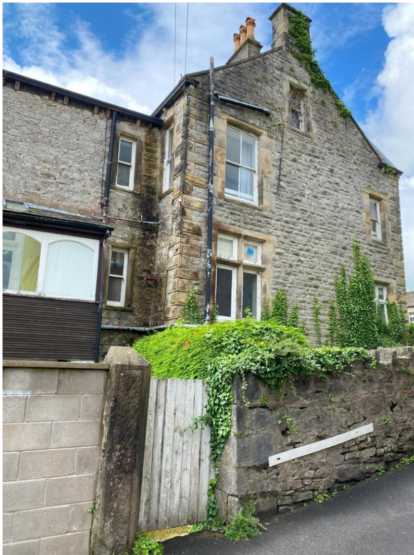
6 North east elevation showing hierarchy of window openings.
