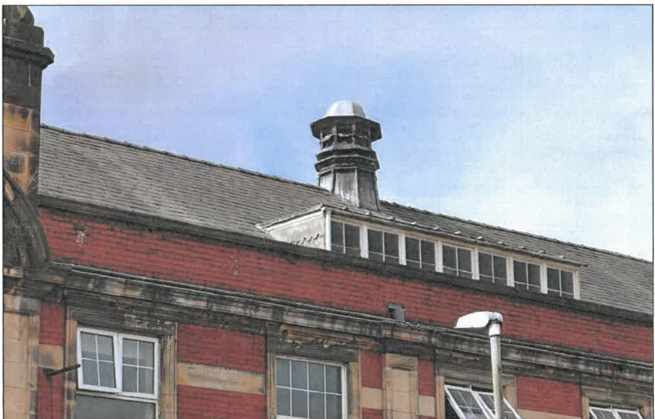
Photo 8: Detail of roof, with cupola (vent) and dormer window, George Street elevation, looking south-west
