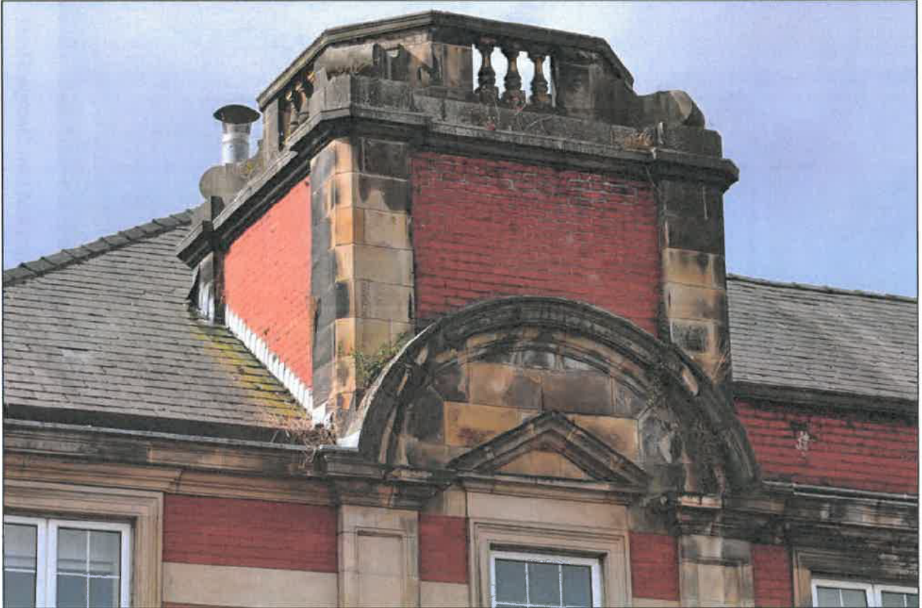
Photo 7: Detail of east turret, looking south-west, George Street elevation, looking south-west
