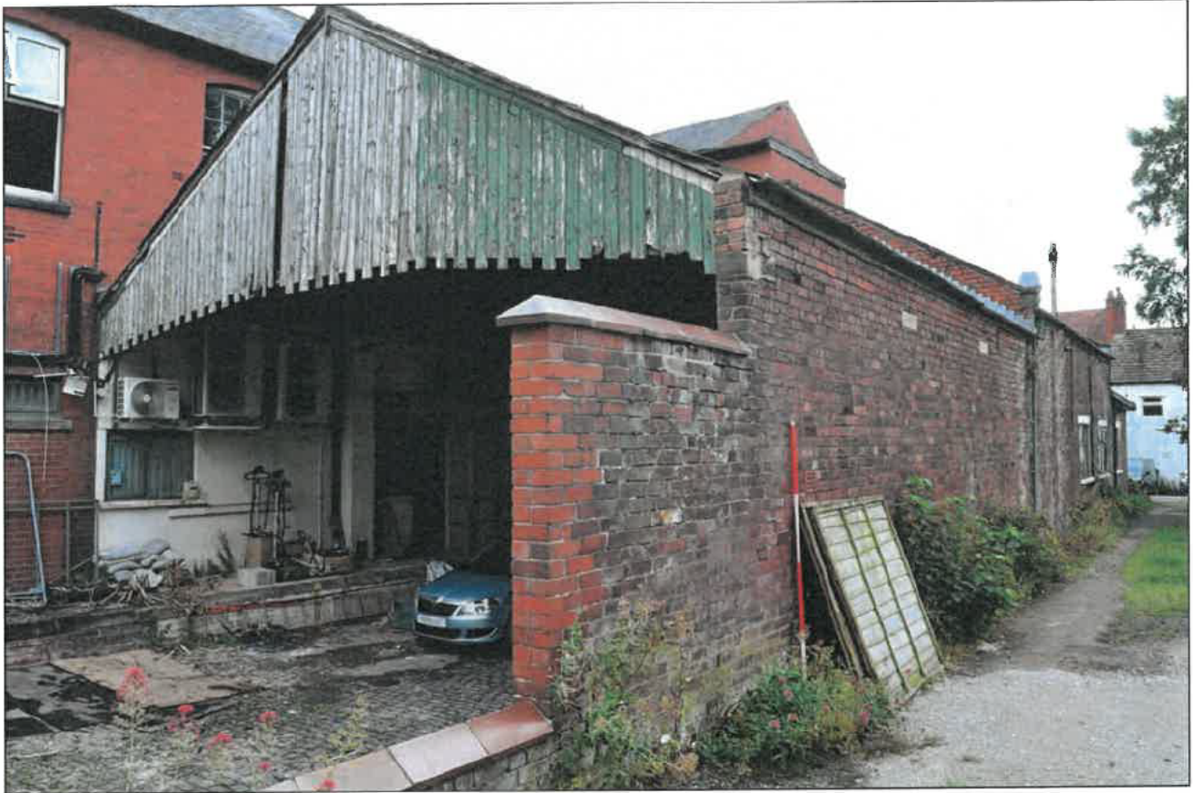
Photo 15: Covered loading area at rear of building, looking north-east
