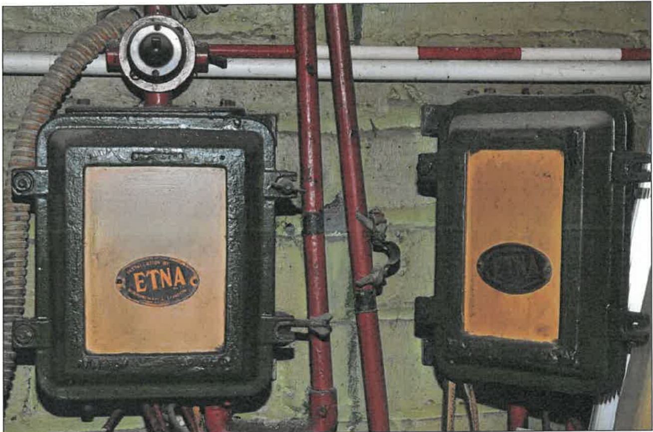
Photo 46: Detail of wiring installation on north side of projection room
