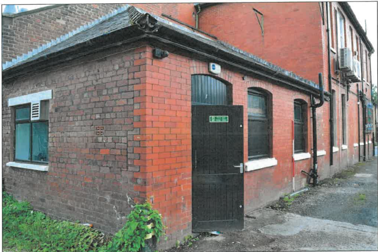
Photo 10: South-east corner of the building
