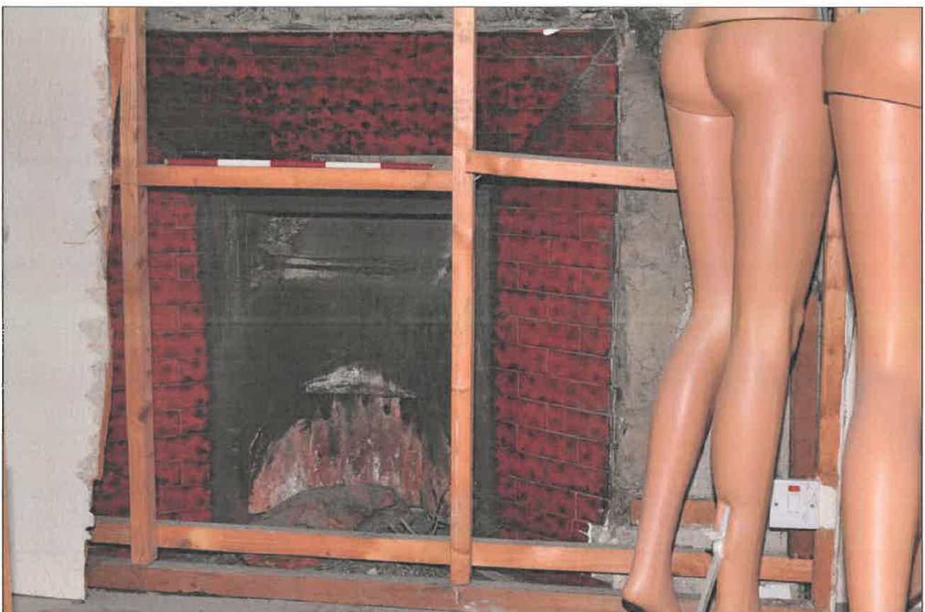
Photo 28: Detail of fireplace in board room or similar, looking south
