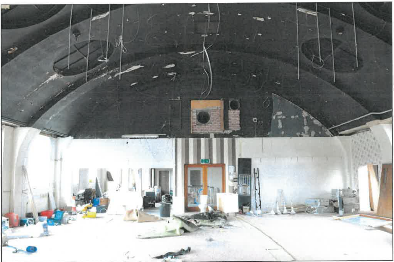
Photo 32: Former cinema, looking east
