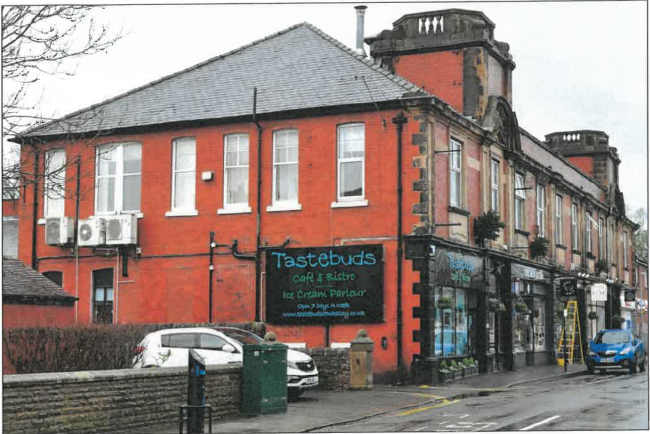
Photo 9: General view of the building, looking south-west across George Street
