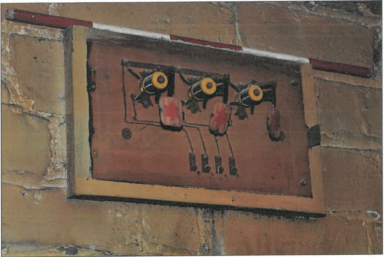
Photo 45: Detail of wiring installation on west side of projection room
