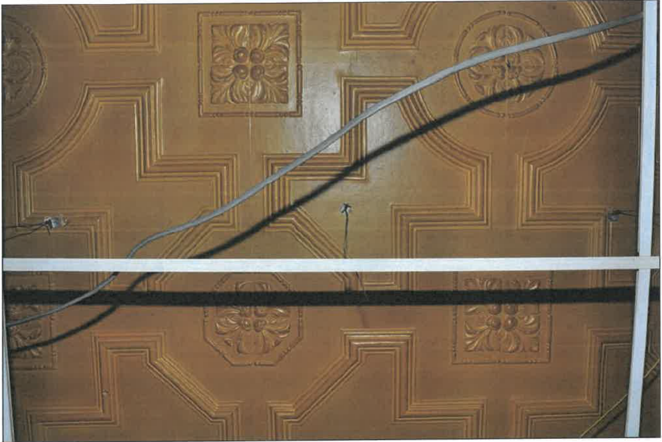
Photo 30: Detail of ceiling over board room or similar
