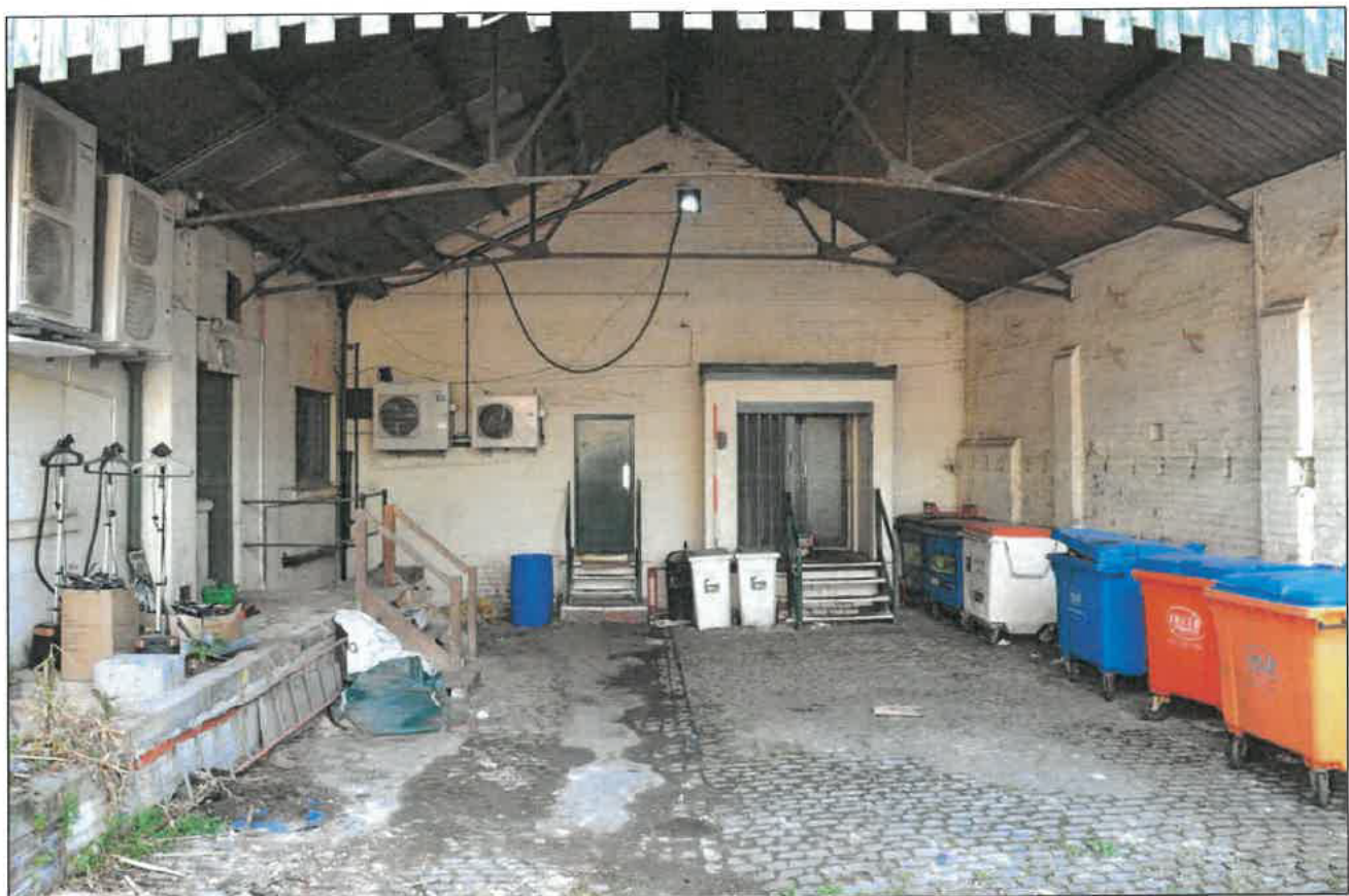
Photo 17: Interior of covered loading area, looking east
