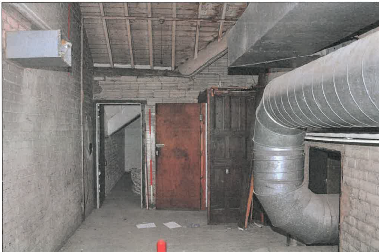
Photo 39: Main second floor room, looking south
