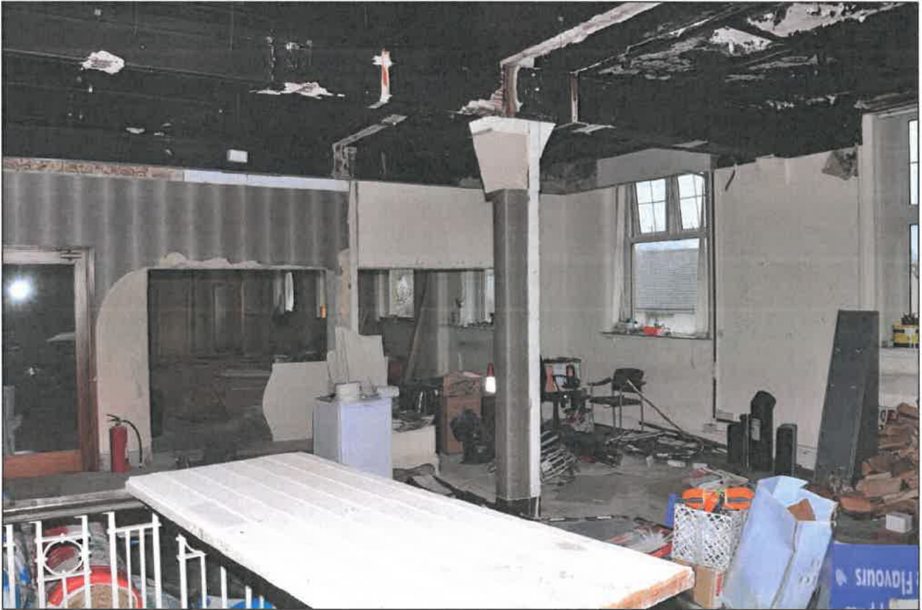
Photo 24: Former foyer to cinema, on first floor, looking north-west
