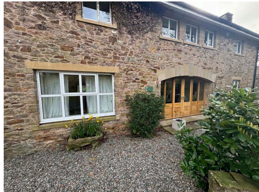
'Fake' stone arch and corbelled roof overhang
