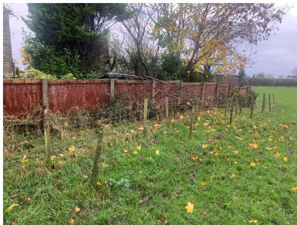
Photograph 2 – A southern section of H1, present in between fencing
