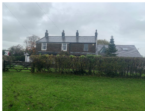
Photograph 5 – Western half of H2
