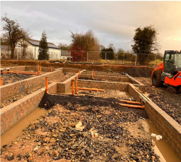
Fig 7 - Internal drainage pop up installation.
