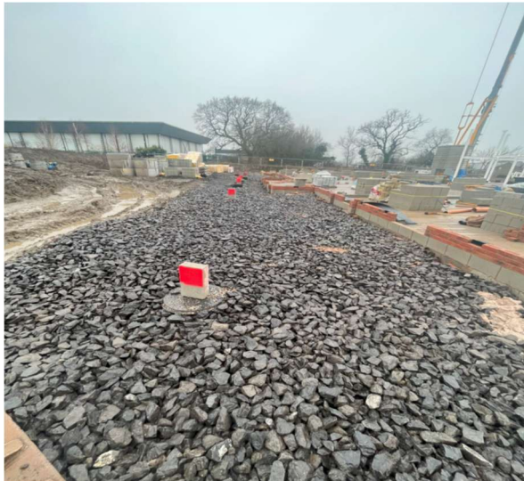
Fig 8 - External drainage run installation.
