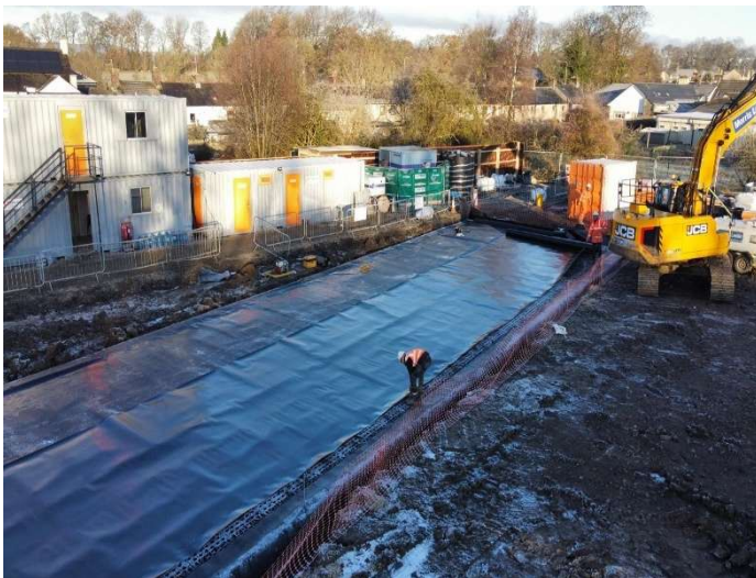
Fig 3 – Attenuation crates wrapped in impermeable membrane.
