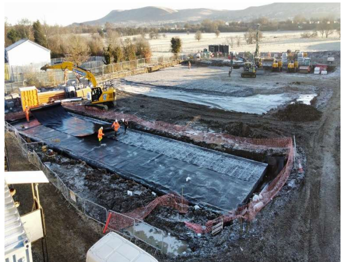
Fig 4 – Attenuation crates wrapped in impermeable membrane.
