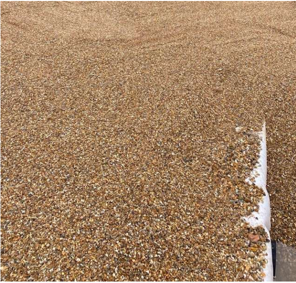
Fig 5 - Fleece protection & Bedding infill around tank.
