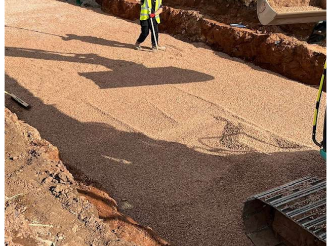
Fig 2 – Attenuation Hole excavated filled with bedding.
