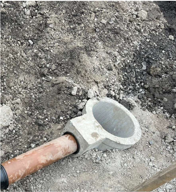
Fig 11 - Gully installation to carpark as per design.
