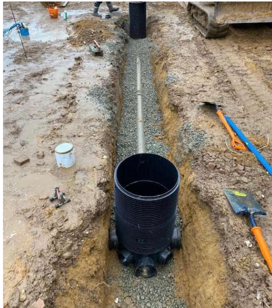
Fig 12 - External drainage run installation.
