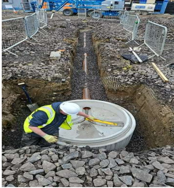
Fig 12 - External drainage run installation.
