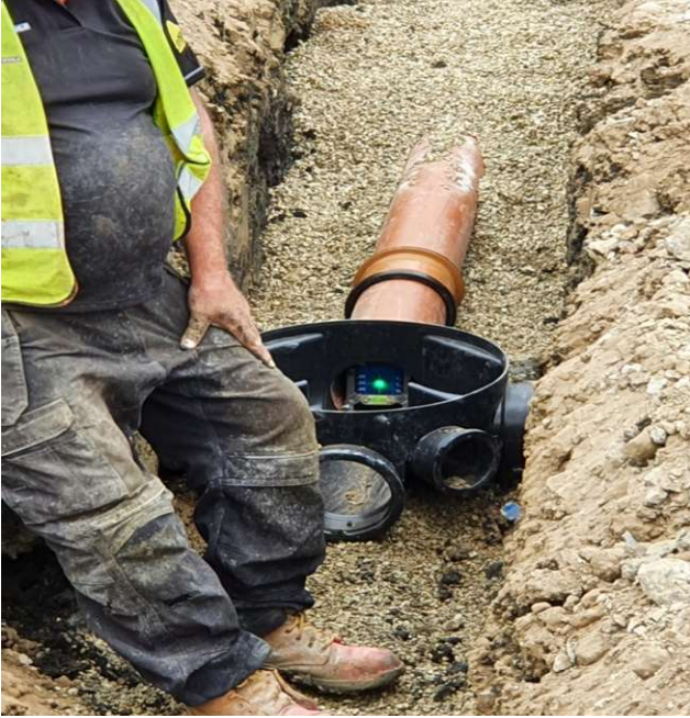
Fig 11 - Gully installation to carpark as per design.
