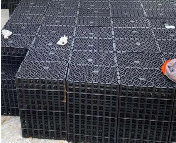
Fig 1 – Attenuation crate stockpile on site.
