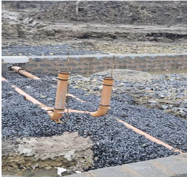
Fig 6 - Internal drainage pop up installation.
