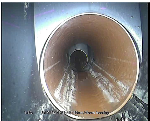
F34X_35994a9d-506a-4404-8cf3-6aa3551530a1_20250113_081354_950.jpg, 00:00:50, 6.83 m Finish node, manhole, reference: F33
