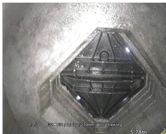
F32X_11d08de3-ed06-4626-9b91-d94624265668_20250113_082035_028.jpg, 00:01:02, 5.78 m Finish node, manhole, reference: F31
