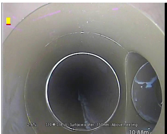
S19X_c9a65b3a-d43f-4d96-aee1-a3b521ab065a_20250113_082447_027.jpg, 00:01:13, 10.88 m Junction at 3 o'clock, diameter: 100mm
