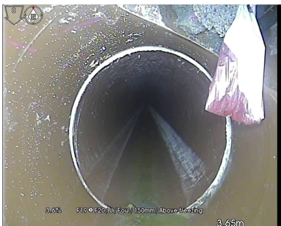
F20X_4226e9a2-02a5-4848-8a22-caf435f20f7a_20250113_094424_560.jpg, 00:00:28, 3.65 m Junction at 1 o'clock, diameter: 100mm
