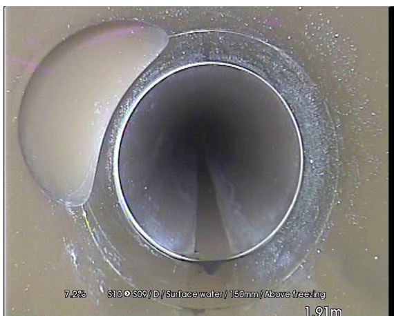
S10X_f9446d50-ba42-498e-849a-1707c933ff99_20250113_084646_473.jpg, 00:00:13, 1.91 m Junction at 10 o'clock, diameter: 100mm
