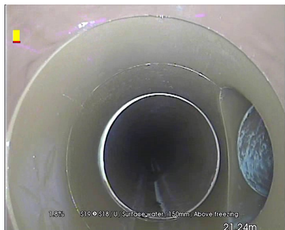
S19X_0696d987-2a7a-43a5-9448-b5d8fa67a5ff_20250113_082611_492.jpg, 00:02:14, 21.24 m Junction at 3 o'clock, diameter: 100mm
