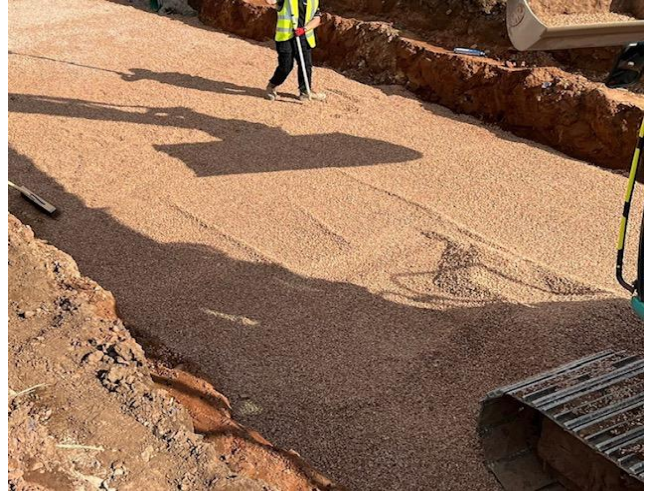
Fig 2 – Attenuation Hole excavated filled with bedding.
