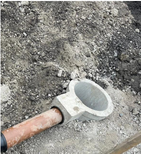
Fig 11 - Gully installation to carpark as per design.
