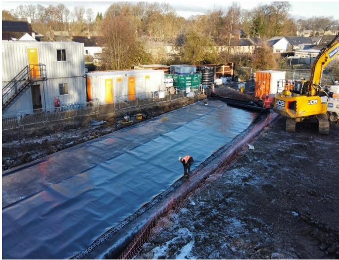
Fig 3 – Attenuation crates wrapped in impermeable membrane.
