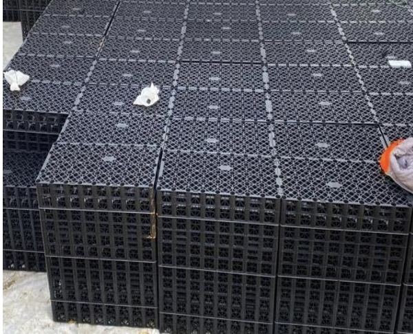
Fig 1 – Attenuation crate stockpile on site.
