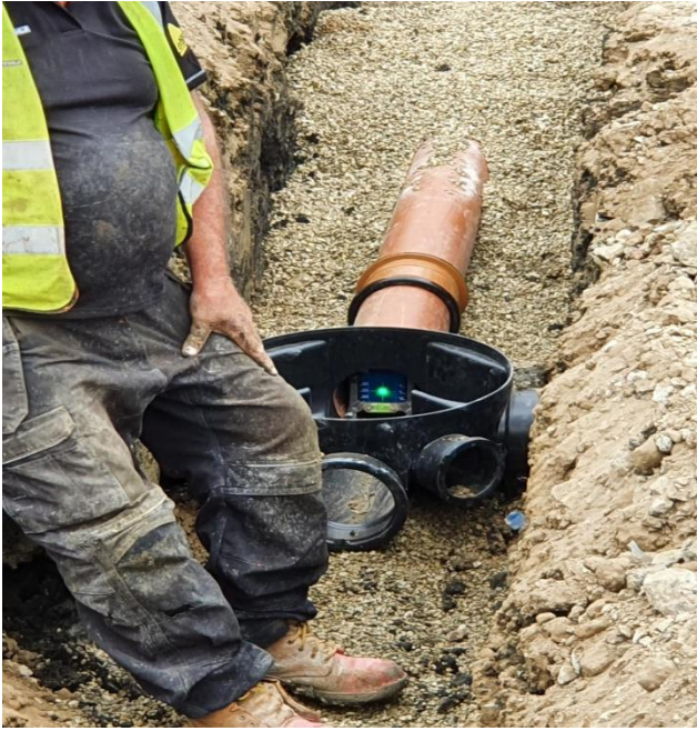
Fig 11 - Gully installation to carpark as per design.
