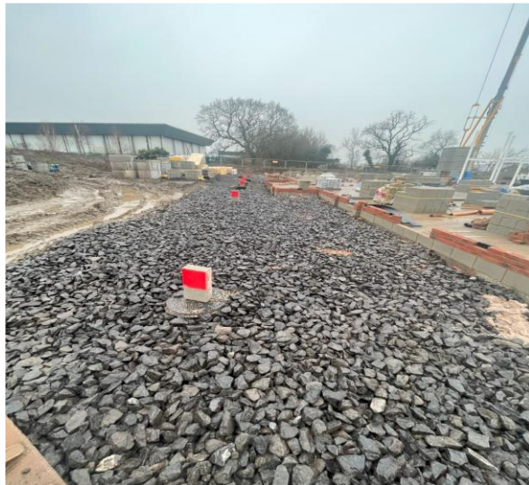
Fig 8 - External drainage run installation.
