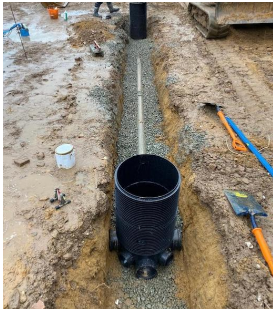
Fig 12 - External drainage run installation.
