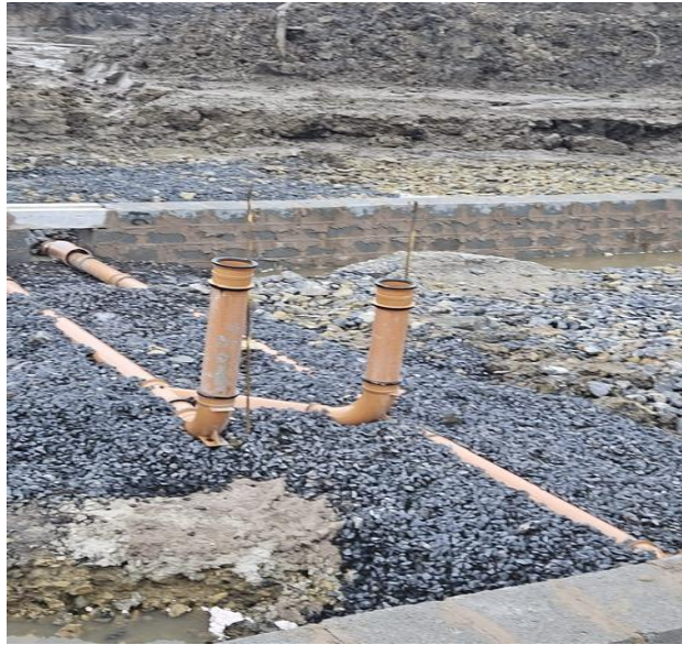
Fig 6 - Internal drainage pop up installation.
