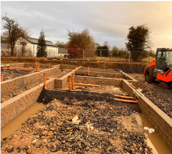
Fig 7 - Internal drainage pop up installation.
