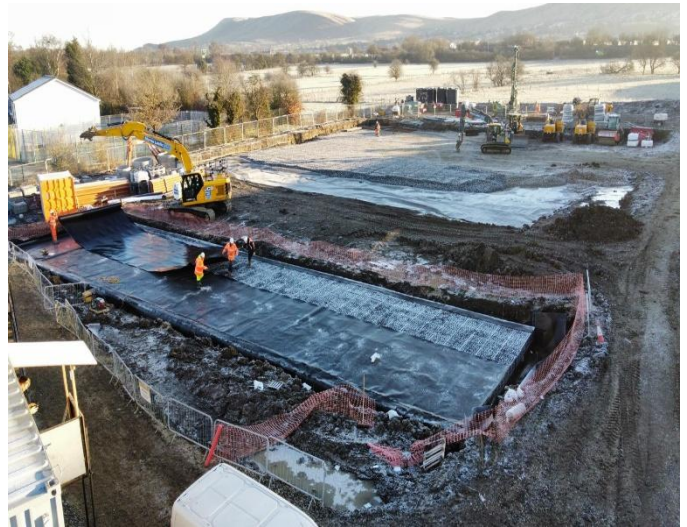
Fig 4 – Attenuation crates wrapped in impermeable membrane.
