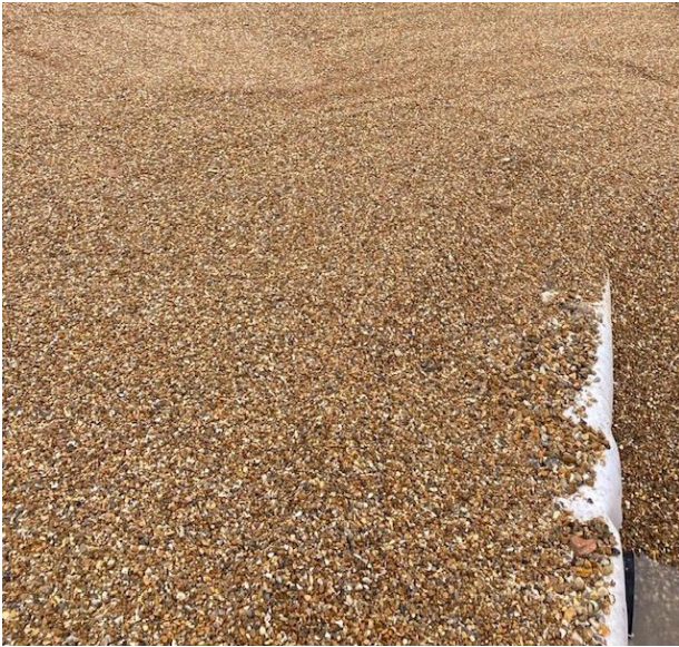
Fig 5 - Bedding infill around tank.
