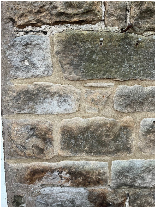
Sample images of re-pointing in lime – Between doorways on Northeast Elevation
