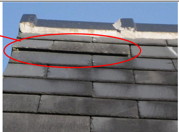
Photo 6: Lifted slate on southern elevation of Building 1
