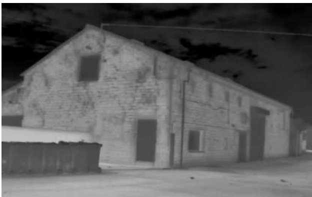
Thermal camera coverage at end of survey
