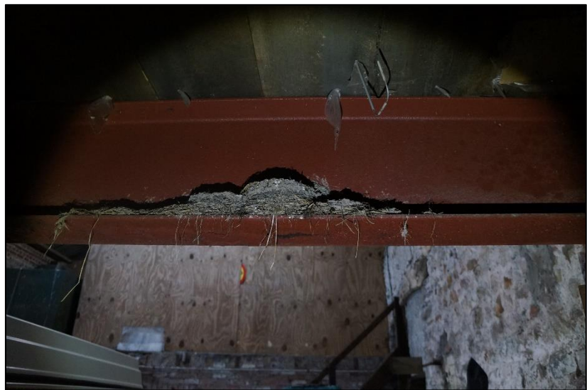
Photo 7: Swallow nests on the girder supporting the mezzanine in the main barn.
