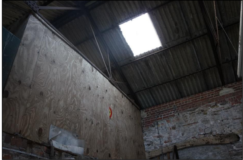
Photo 6: Example of the new roof materials.
