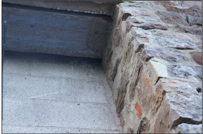
Photo 4: Close up of gaps in lintel and blockwork on the east elevation of the barn showing evidence of birds nesting above the wood lintel, and the smaller gap suitable for bats to roost..
