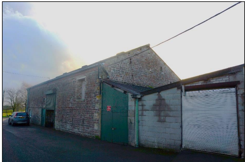
Photo 4: East elevation of the barn and single story extensions.
