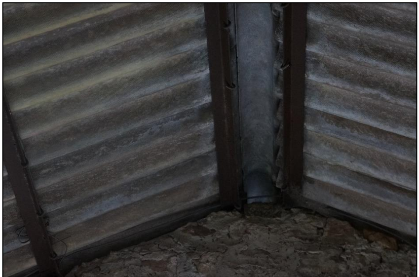
Photo 5: Example of the roof materials.
