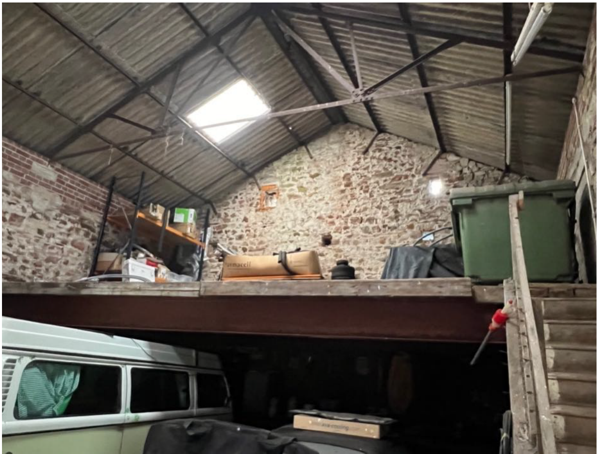
Photo 17 – Internal looking North West
