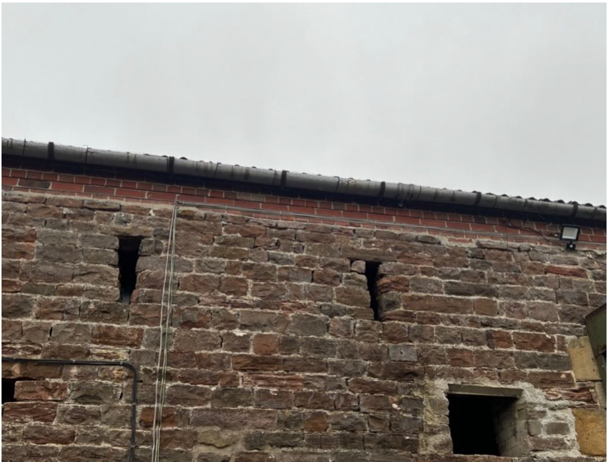
Photo 7 – North East Elevation
