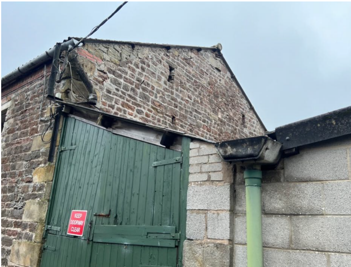
Photo 13 – North West Elevation
