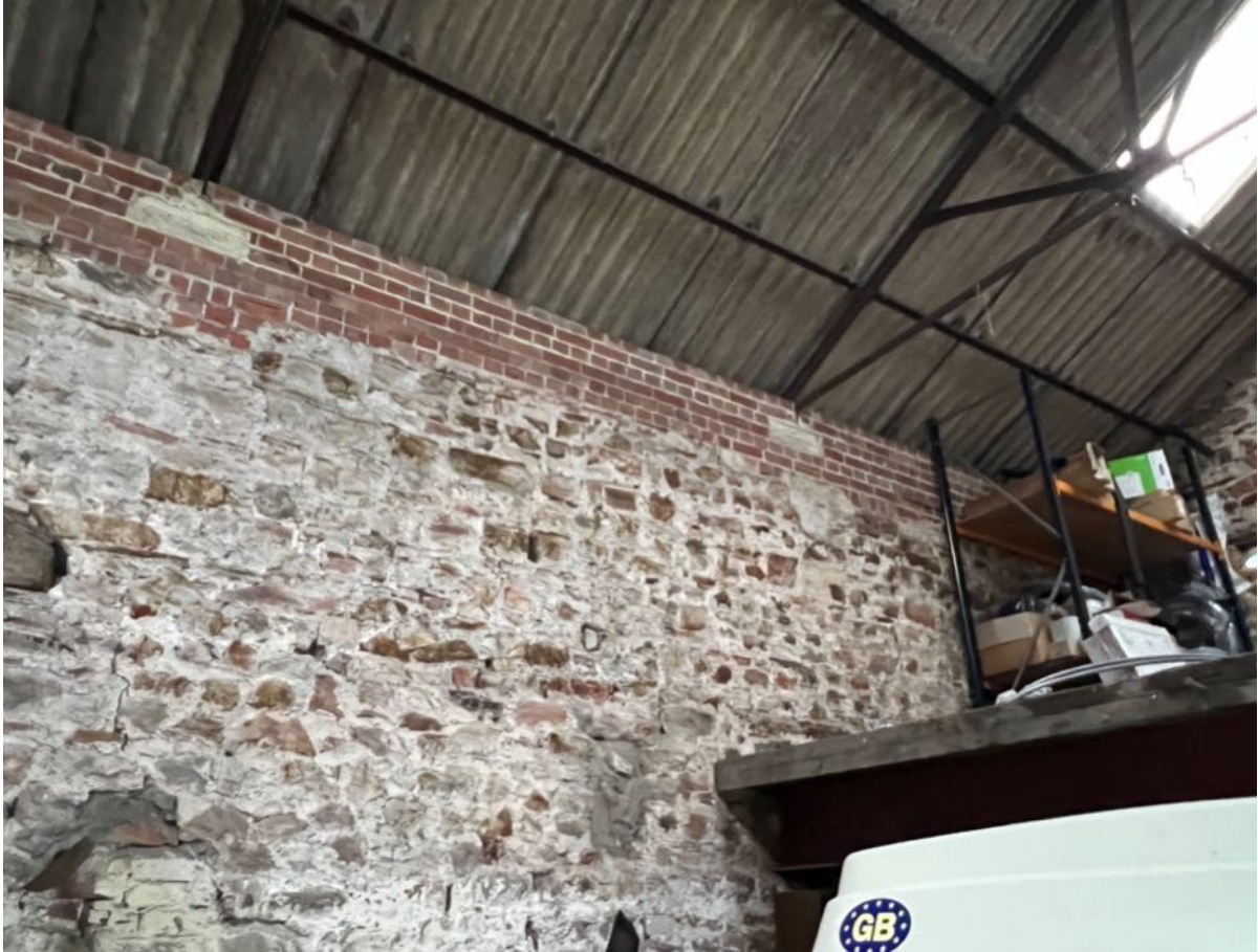
Photo 22 - South West Wall Internal with storage mezzanine at North West end
