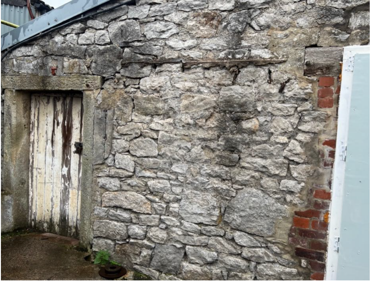
Photo 12 - South East Elevation
