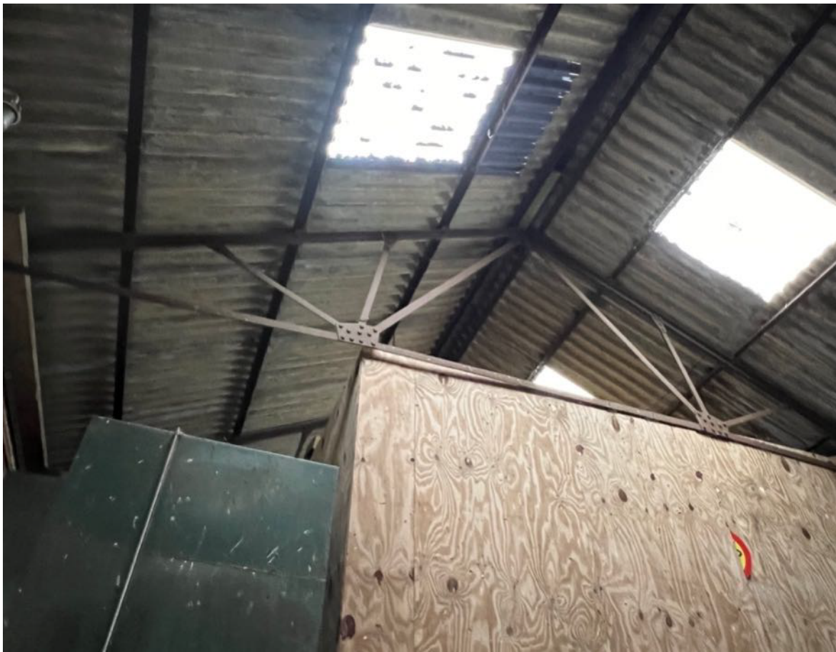
Photo 19 – Internal with storage at North East End
