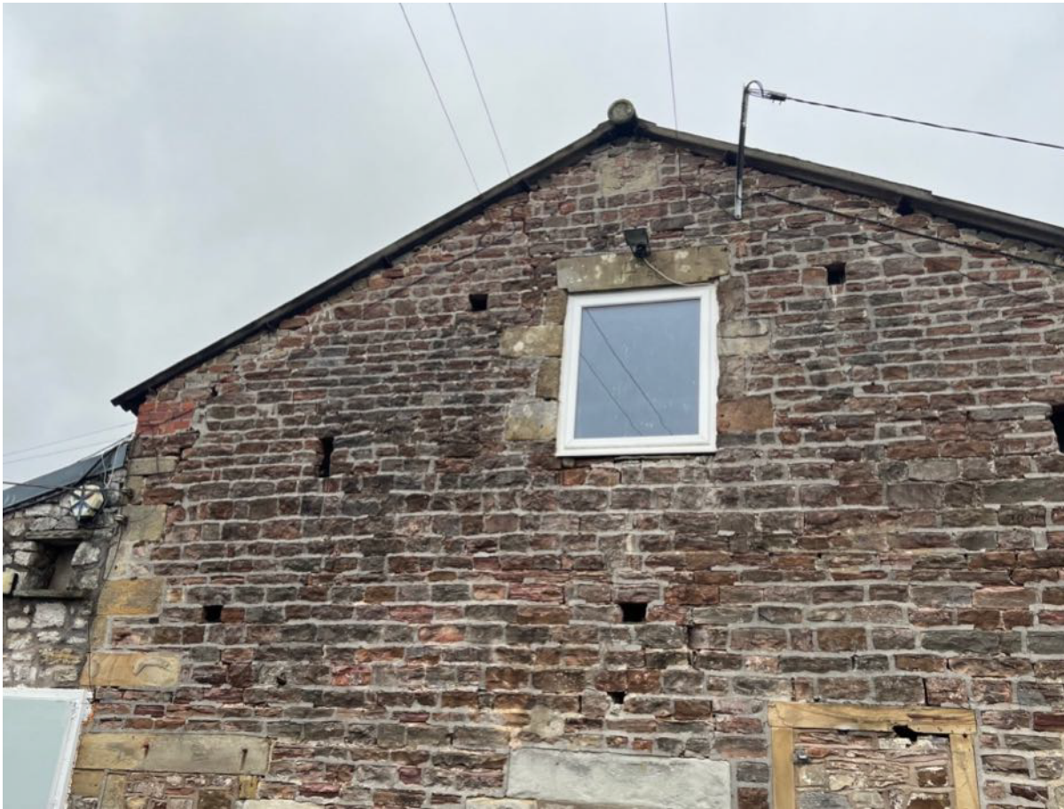
Photo 10 – South East Elevation
