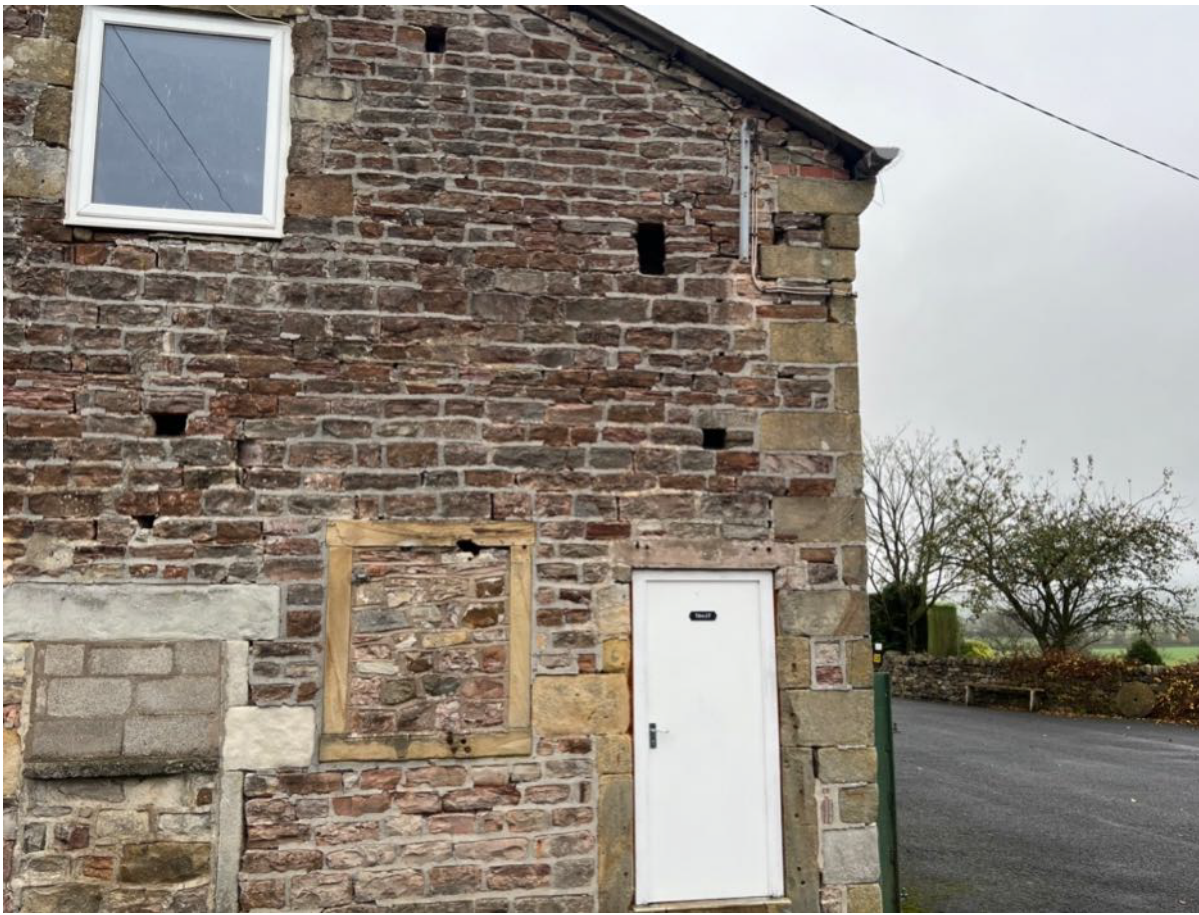
Photo 9 – South East Elevation
