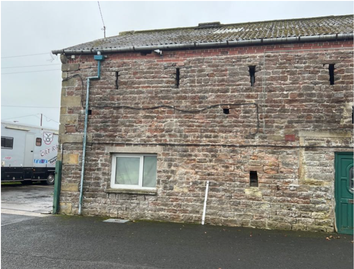
Photo 6 – North East Elevation
