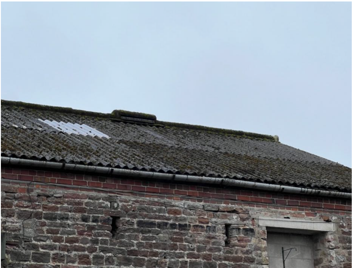
Photo 5 – North East Elevation and roof
