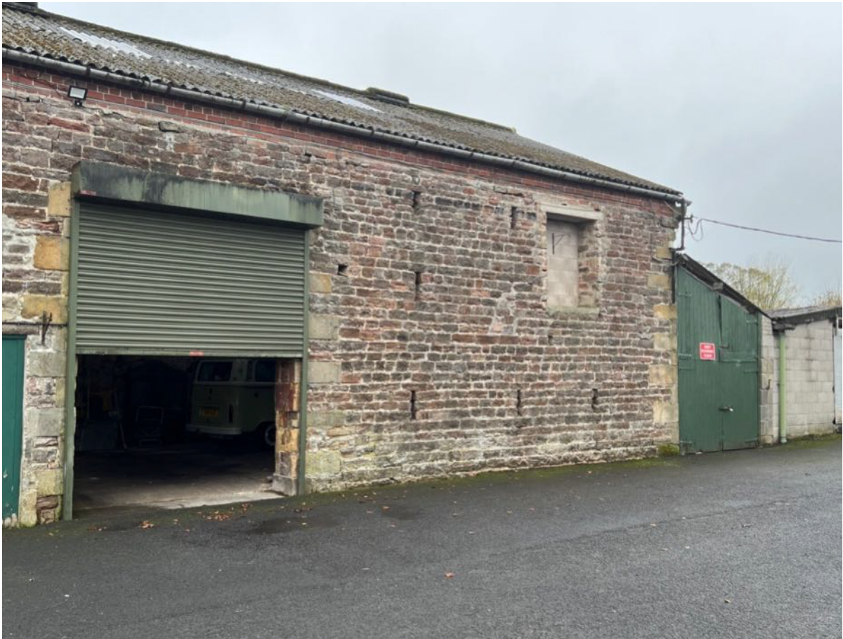
Photo 2 – North East Elevation
