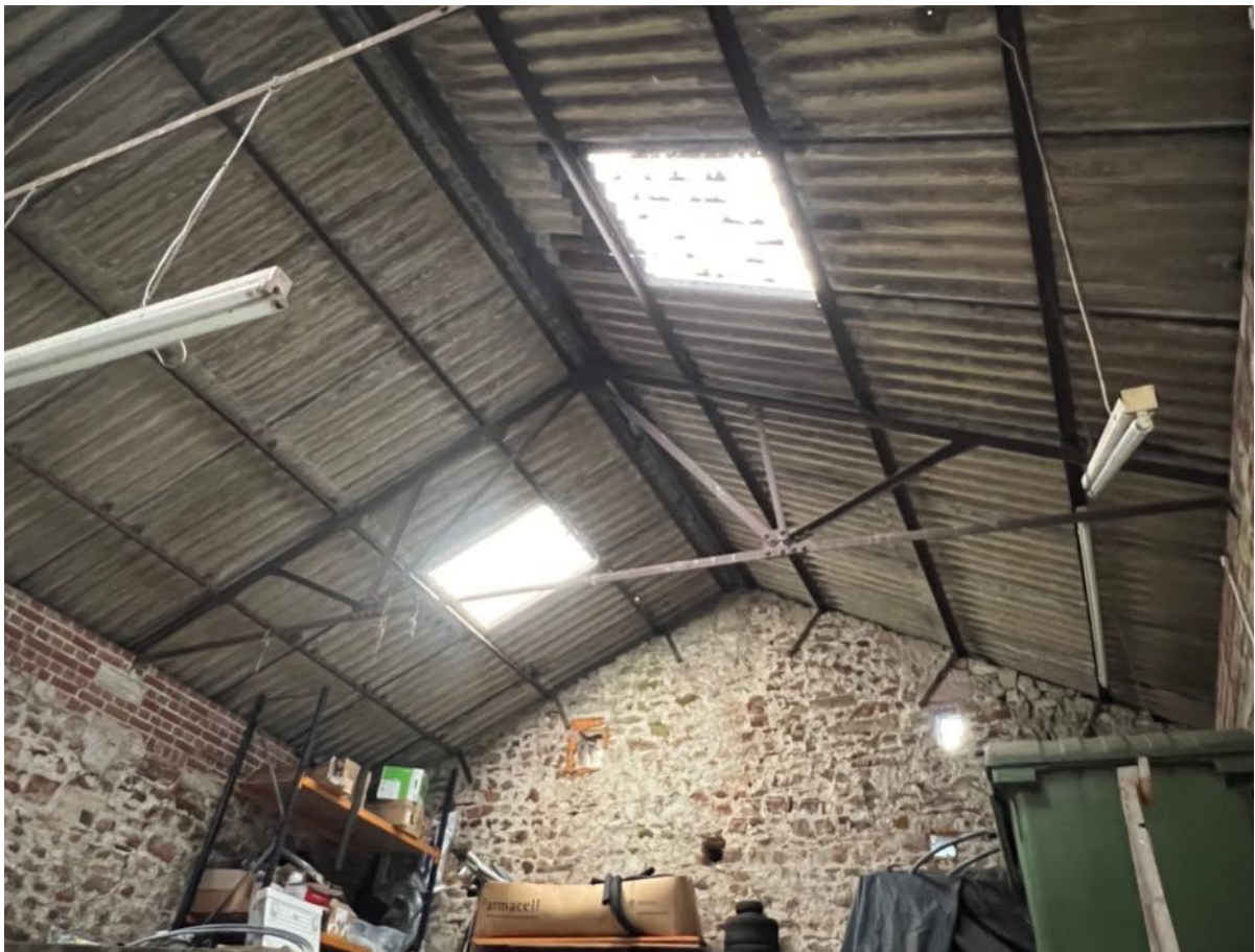
Photo 18 – Internal showing steel trusses and purlins
