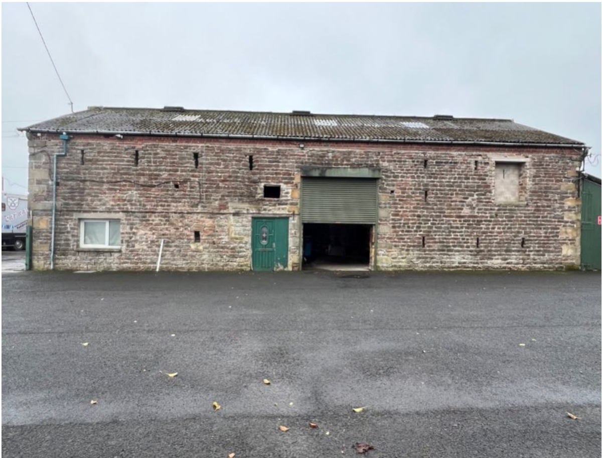
Photo 1 - North East Elevation
