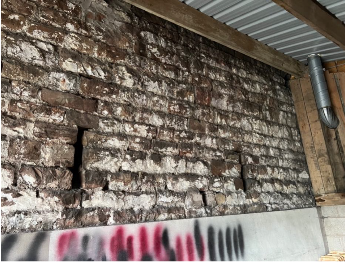
Photo 30 - Rear south west wall of main barn in rear lean to
