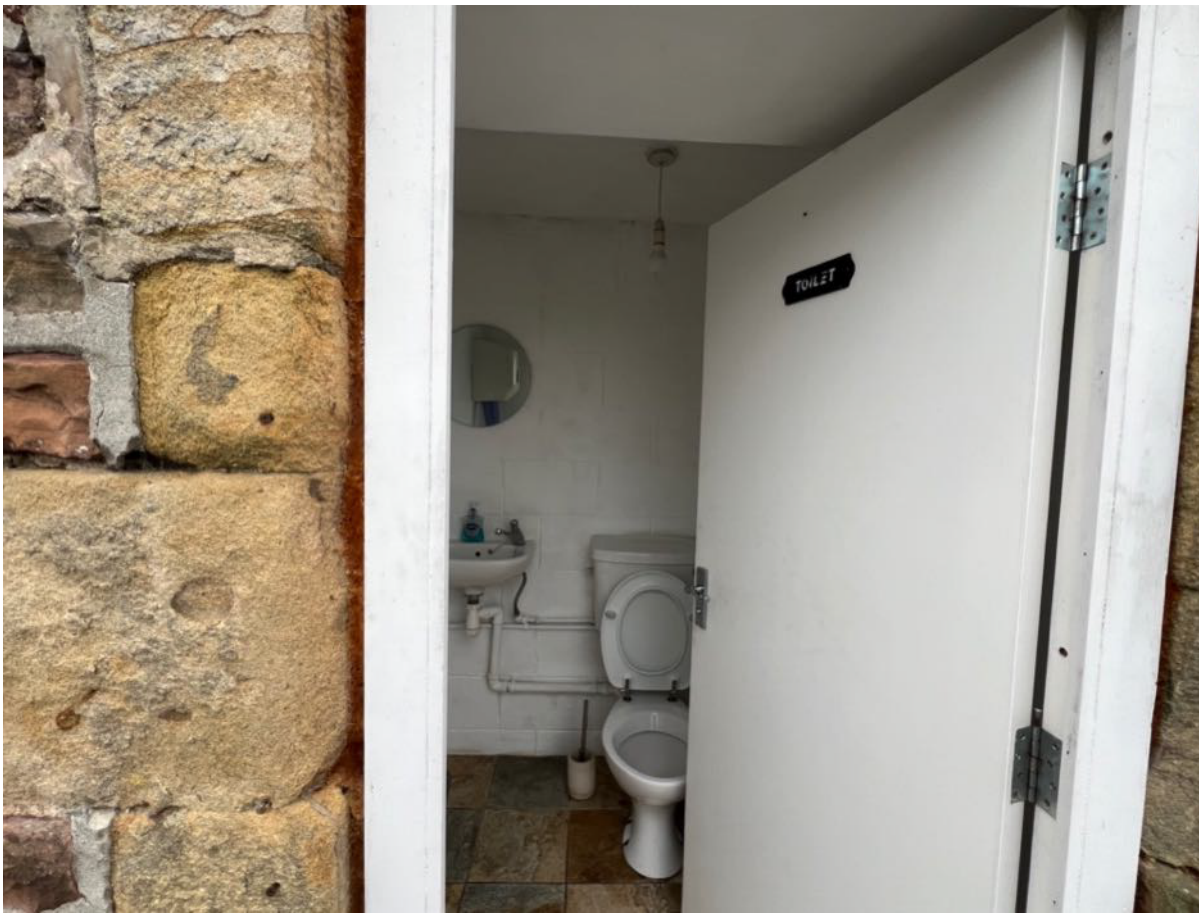
Photo 27 – Toilet at south east elevation
