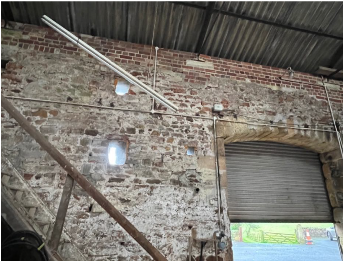
Photo 25 – Internal north east elevation and main door
