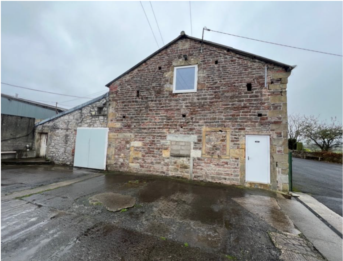
Photo 8 – South East Elevation
