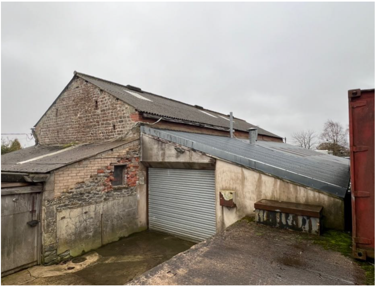
Photo 15 - North West Elevation, rear lean to section and roofs
