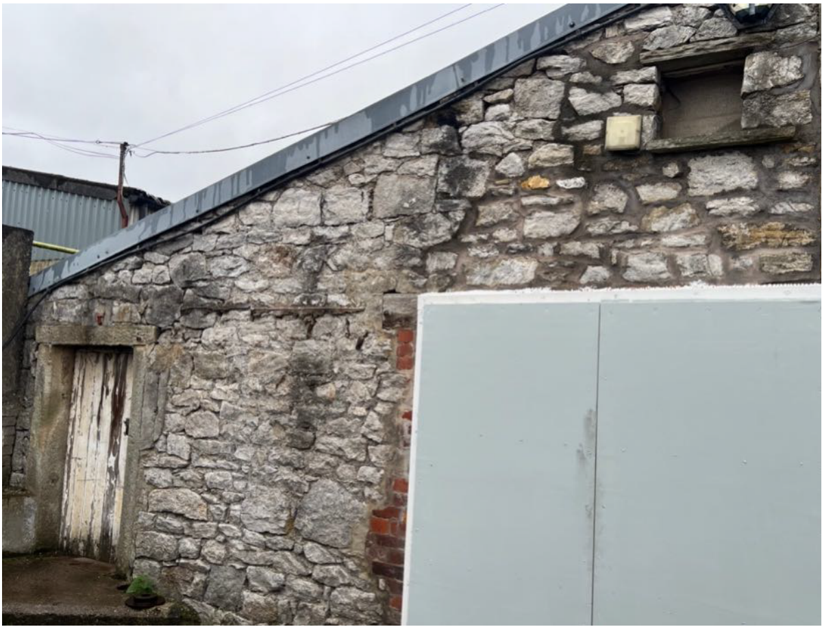
Photo 11 - South East Elevation
