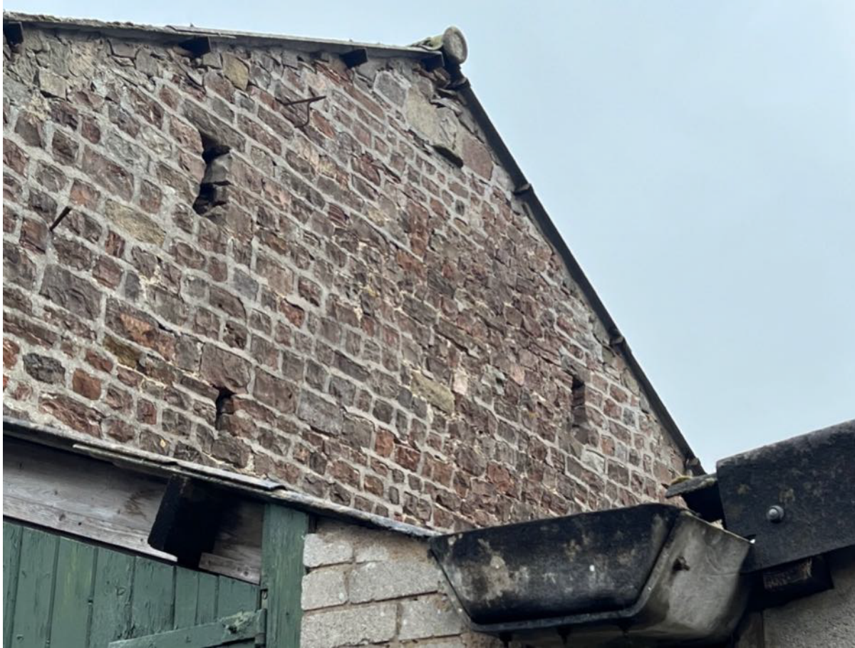
Photo 14 - North West Elevation
