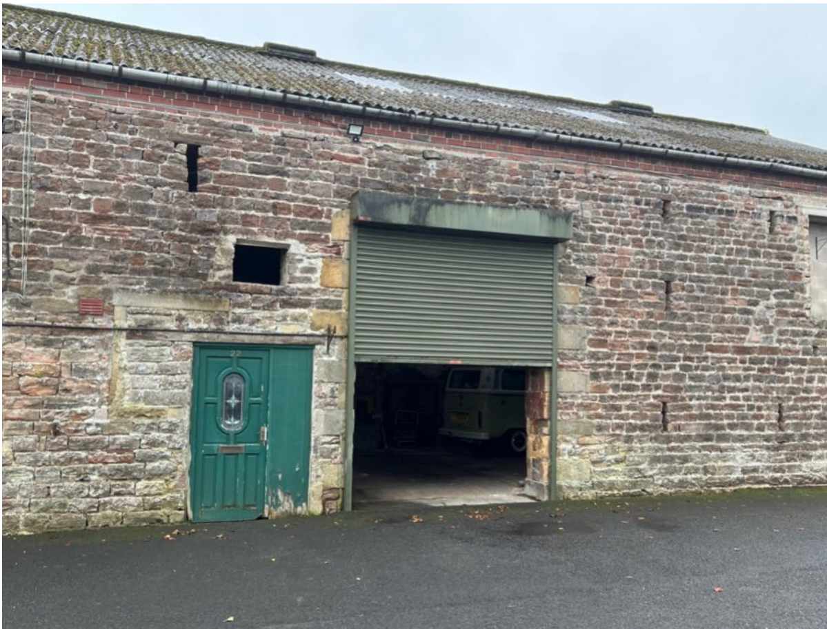
Photo 3- North East Elevation
