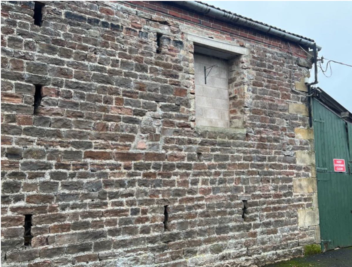
Photo 4 - North East Elevation
