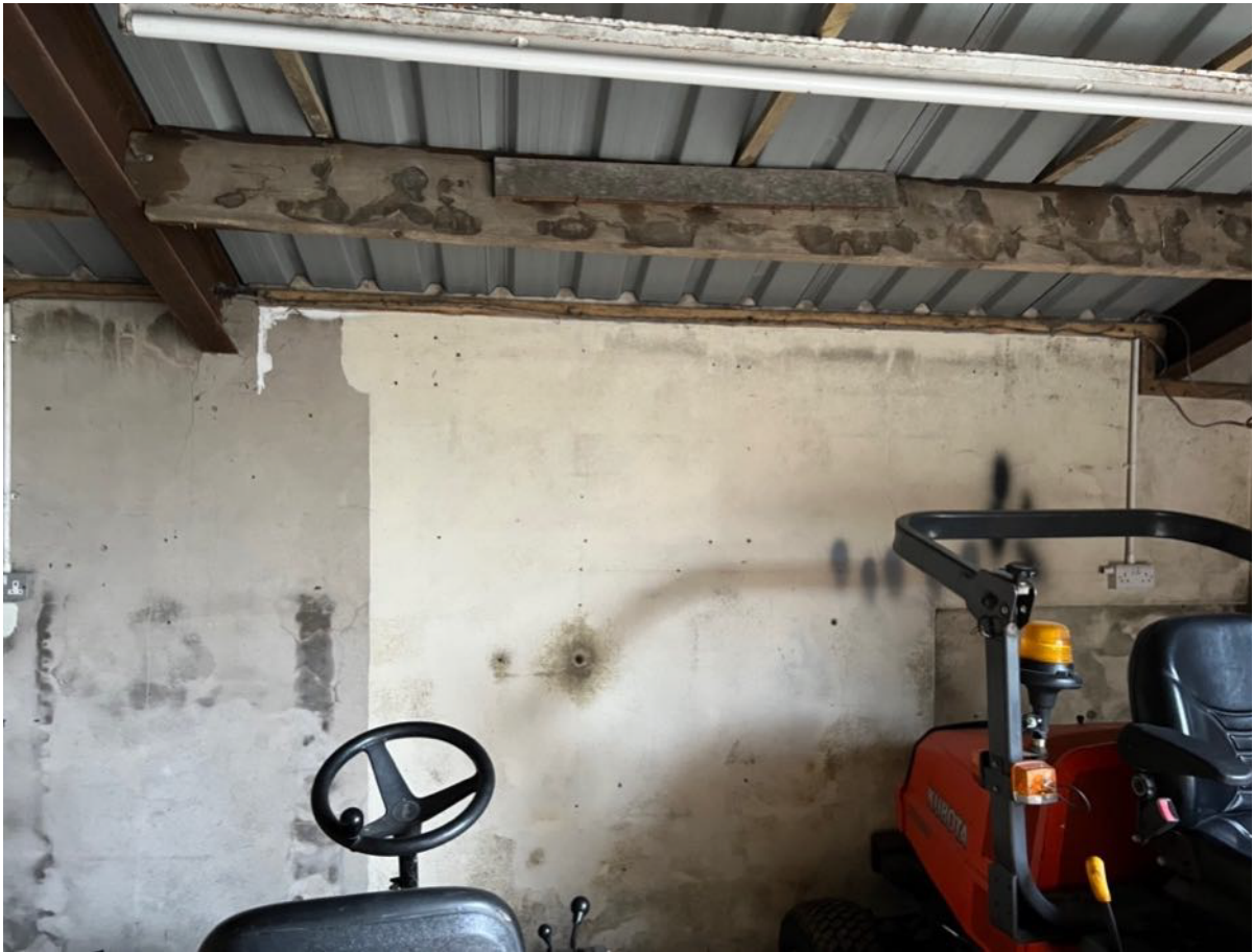
Photo 28 – Rear wall of lean to on south west elevation
