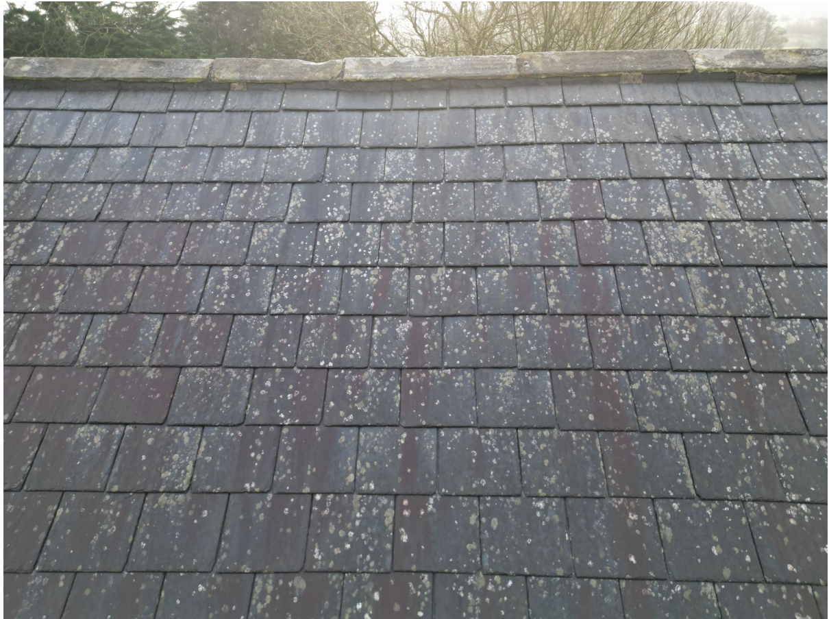
3 – Roof and ridge tiles are in good generally condition.
