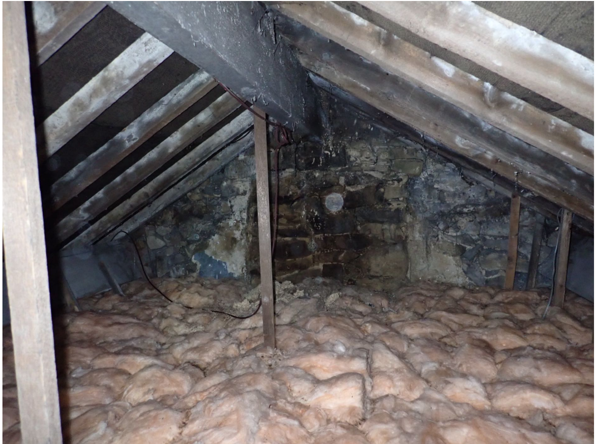
9 – The house has four separate roof voids.
