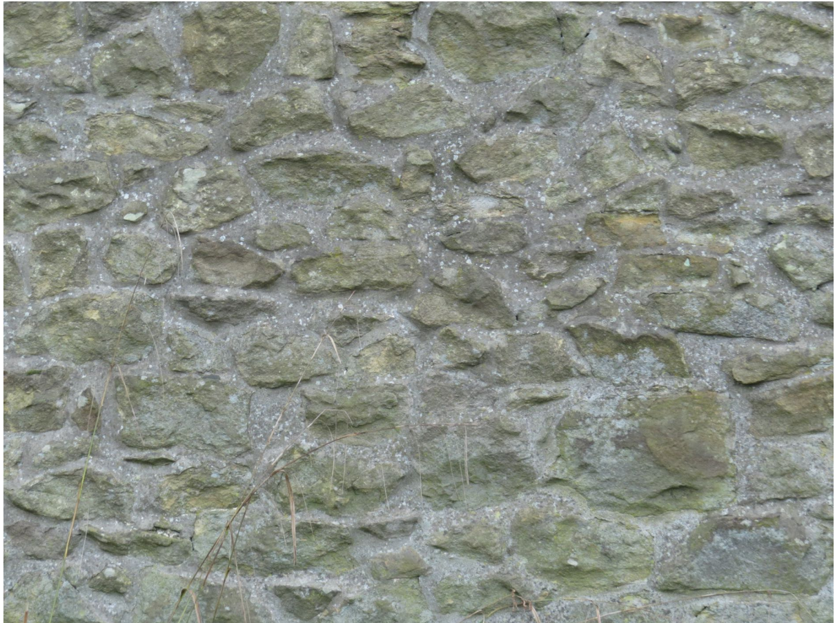
7 – Stonework and mortar is in generally good condition.
