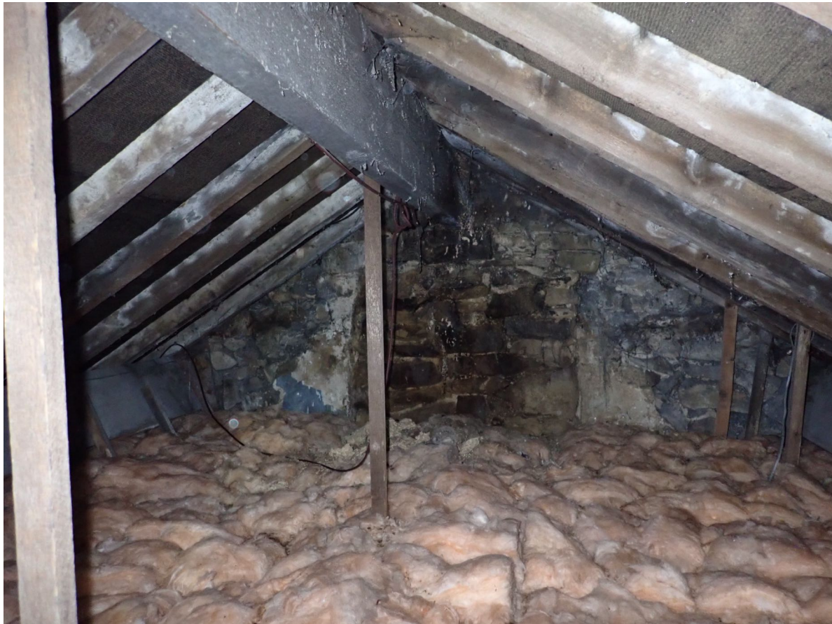
3.2a – A section of the roof void.
